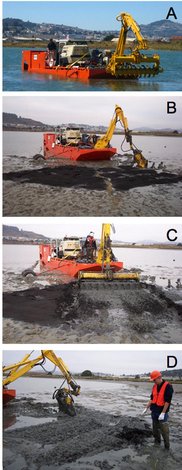
Fig. 2. (A) Mobilizing Aquamog to Plot A at high tide; (B) before, (C) during, and (D) after mixing activated carbon into sediment.
