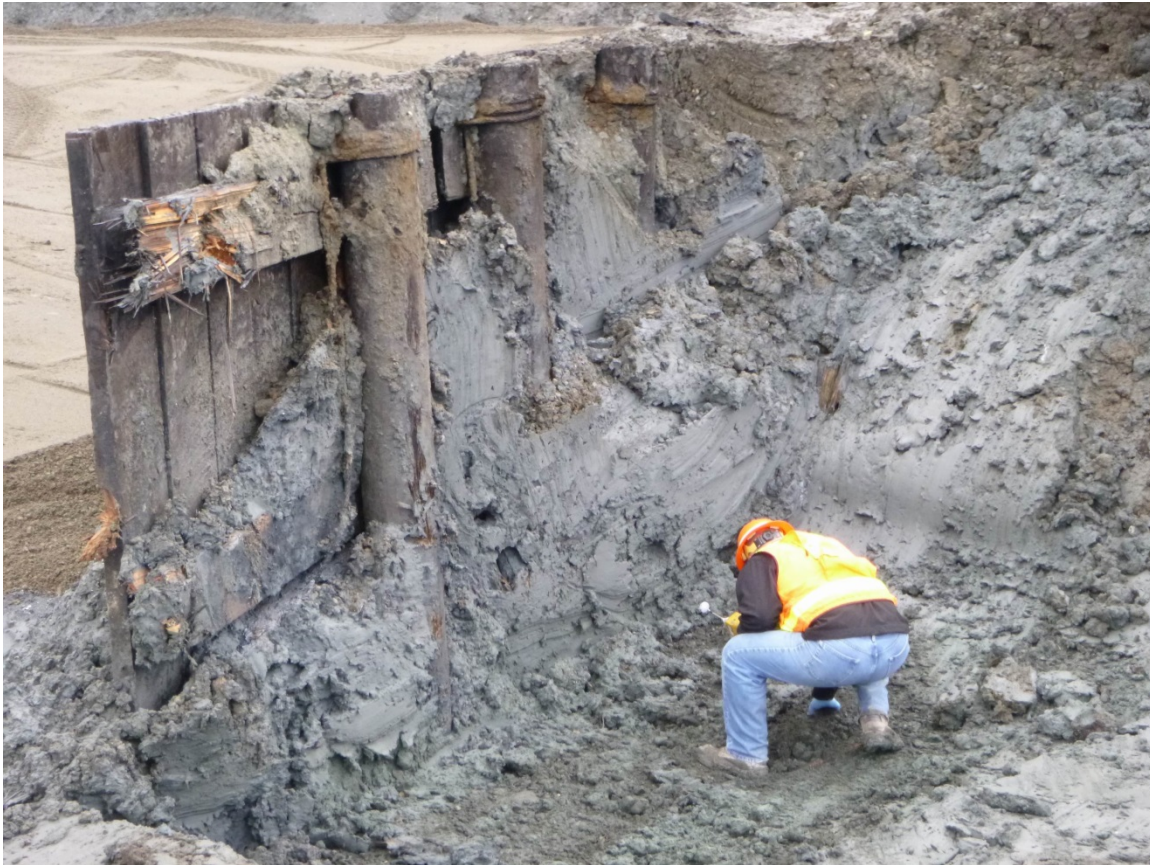
Figure 4: Overview of exposed portion of southwest section of bulkhead, southwest face, along the middle portion of the bulkhead. Note vertical boards, horizontal braces, and cable-wound piles (view to east).
