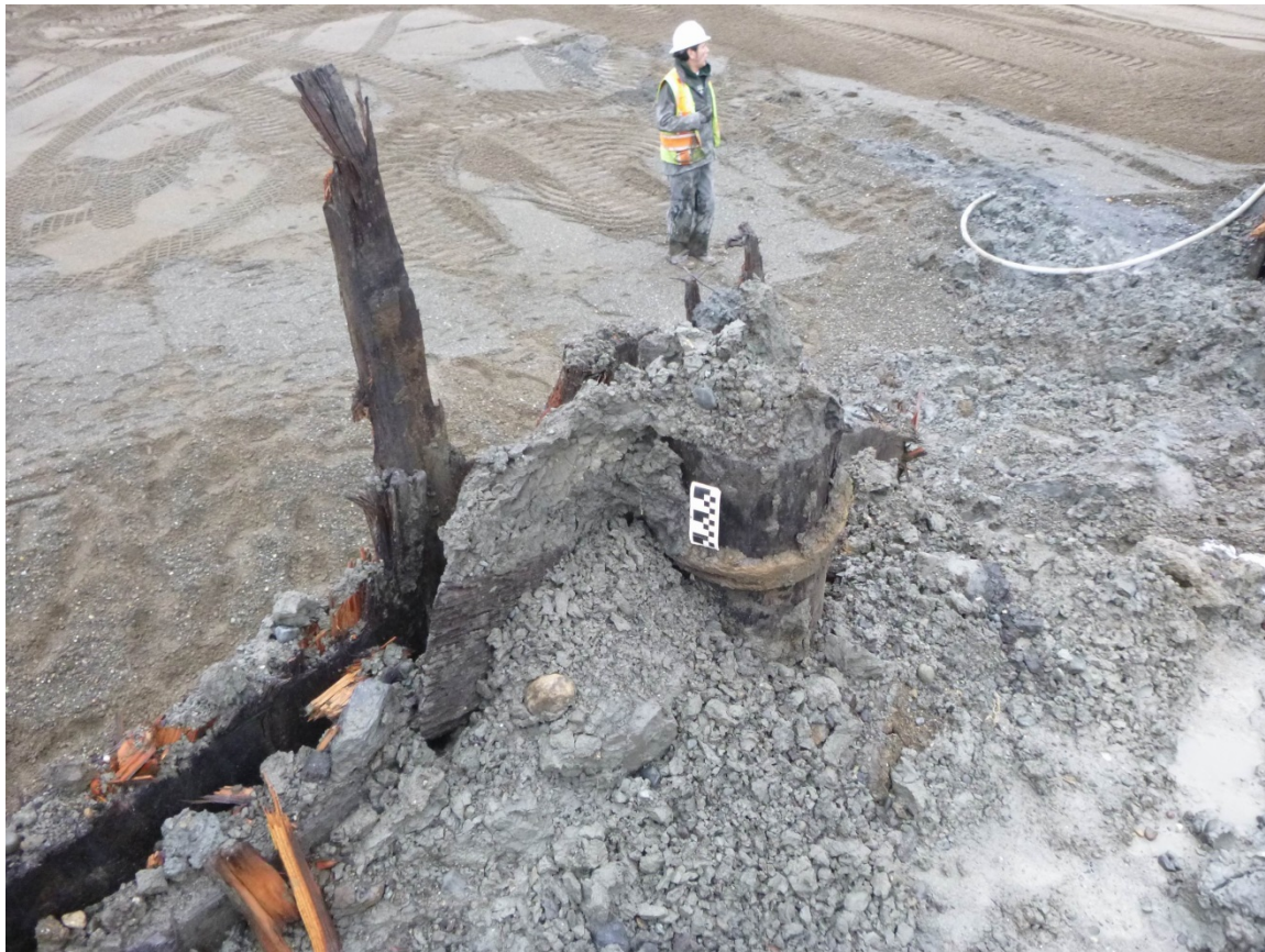
Figure 7: Overview of upper portion of a cable-wound support pile, showing diameter and size of cable (view to southeast).
