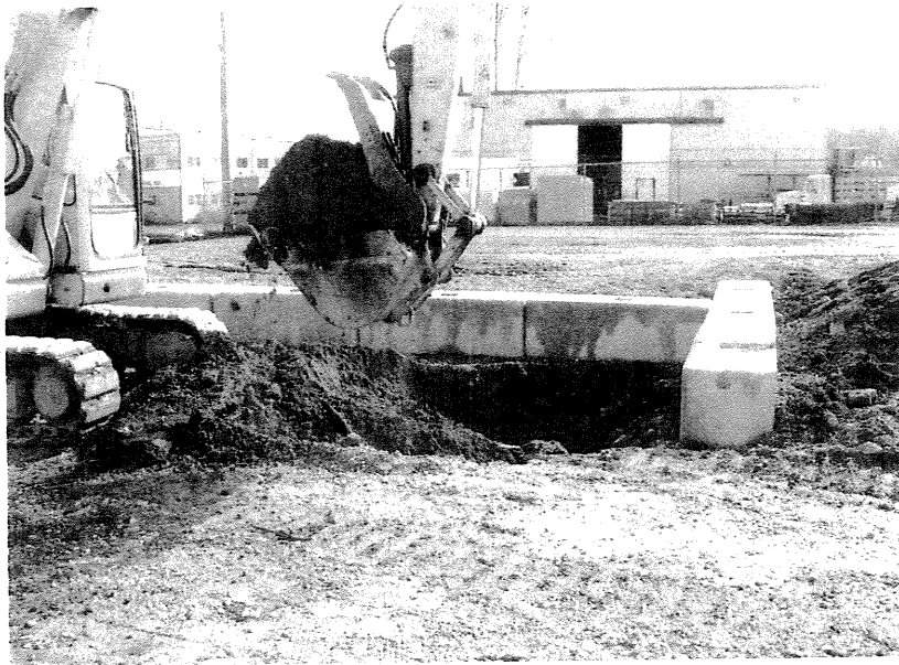
EXPLORATORY EXCAVATION OF SOUTH-EAST YARD.
