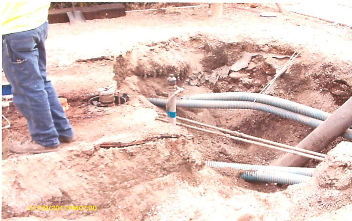
This picture shows the continued vacuuming process and the product lines. This picture was taken looking in an easterly direction.
