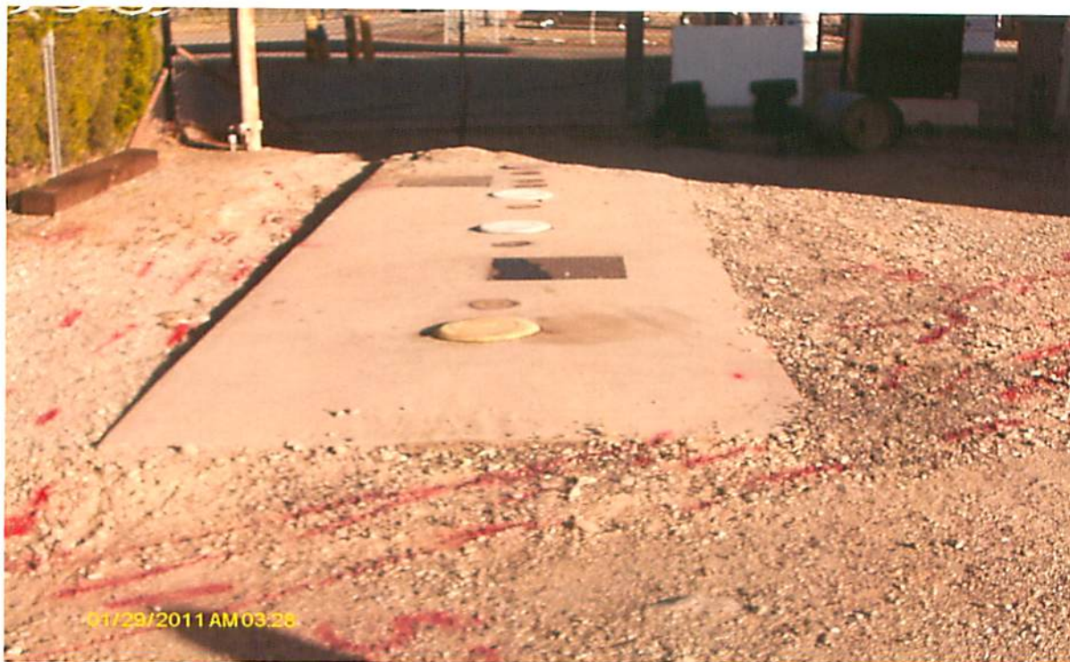
This is the site when ACT first arrived. The release occurred from the far white fill cap. This picture was taken looking in a southeasterly direction.
