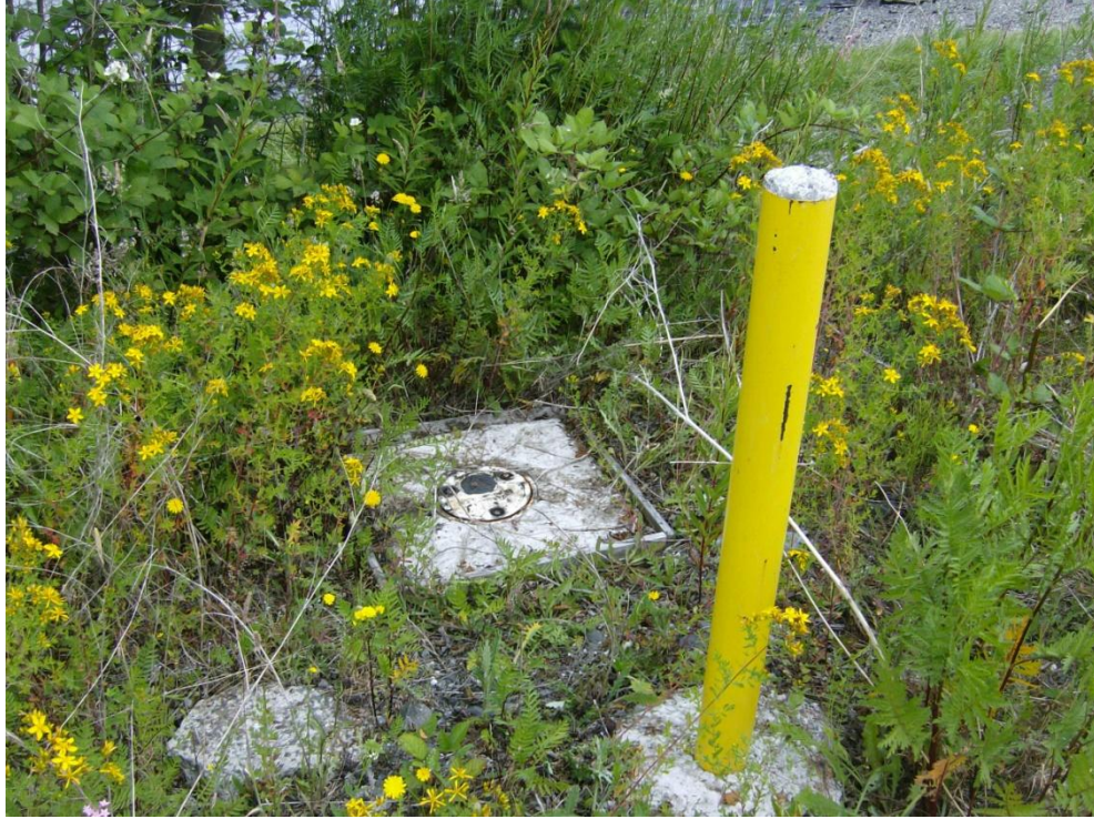
Photo 3: Monitoring Well - near surface water (Snohomish River)
