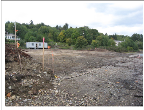
Photo 25. Area E looking northwest after debris screening.
