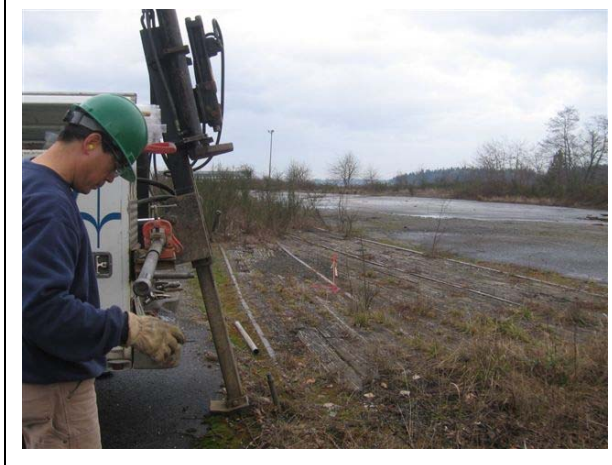
Photo 1. Area A prior to construction during the Phase II Rail Spur Investigation looking northeast.
