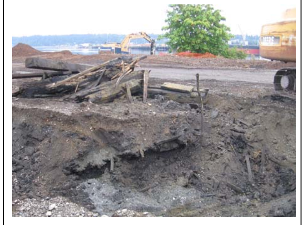
Photo 10. Excavation at Area B looking east. Large timbers noted throughout excavation.
