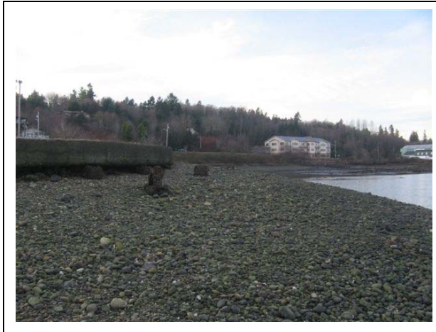
Photo 15. Former wood burner foundation looking north at Area D prior to construction.
