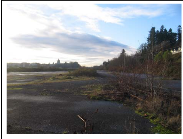
Photo 13. Area C prior to construction looking south along the rail spur.
