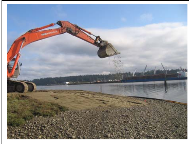
Photo 19. Compacting Area D after additional excavation, looking northeast.
