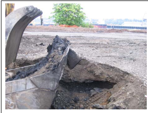
Photo 11. Excavating additional material at Area B looking east.
