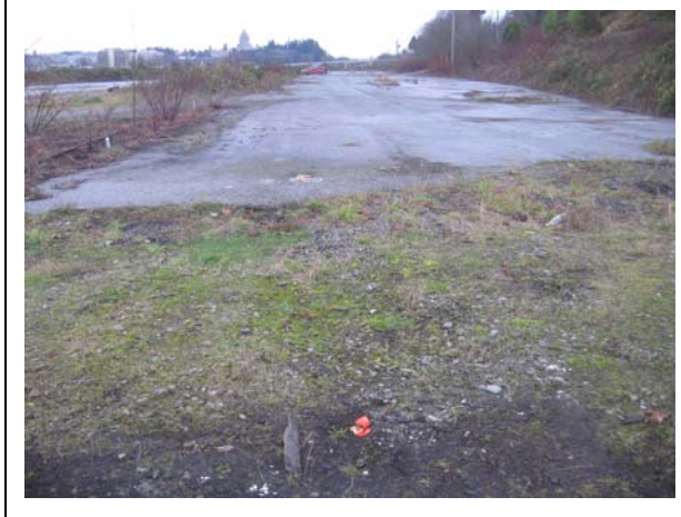
Photo 9. Area B looking south prior to construction.
