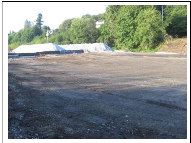
Photo 8. Area A looking southwest completely backfilled and restored.
