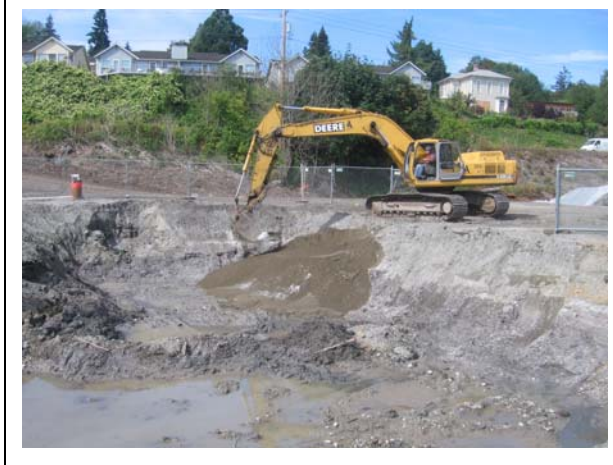
Photo 5. Mixing ORC with clean imported backfill material looking northwest.
