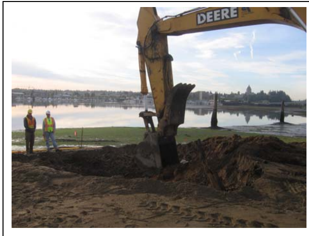
Photo 17. Excavating Area D during low tide looking south.
