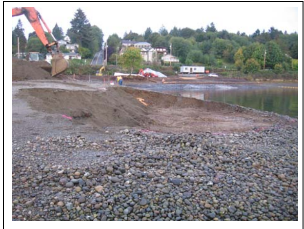
Photo 18. Additional excavation at Area D looking west.
