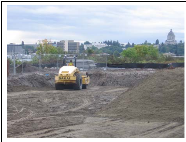
Photo 7. Compacting backfill material looking south towards the Capitol Building.
