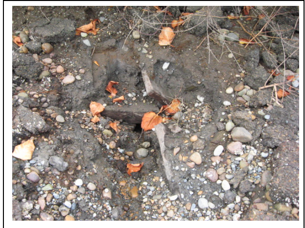
Photo 26. Flume during exploratory excavation showing flow stopped.
