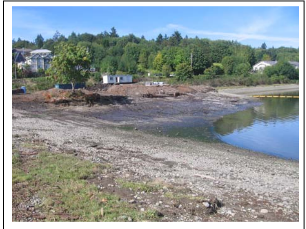
Photo 24. Shoreline looking northwest after pilings have been removed.
