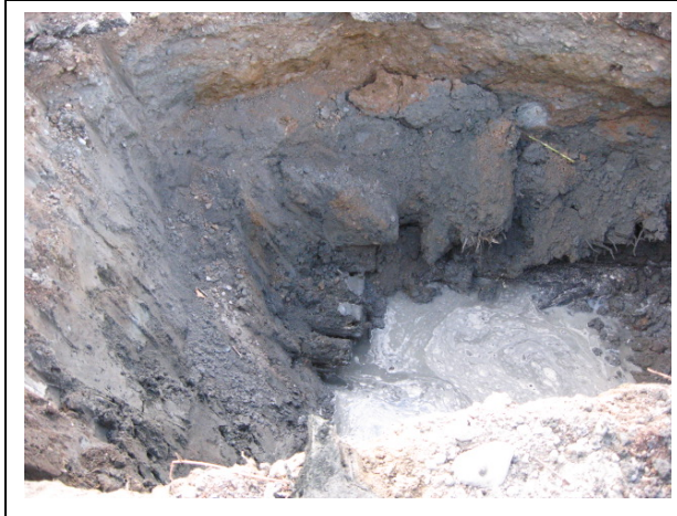
Photo 27. Exploratory excavation for flume.
