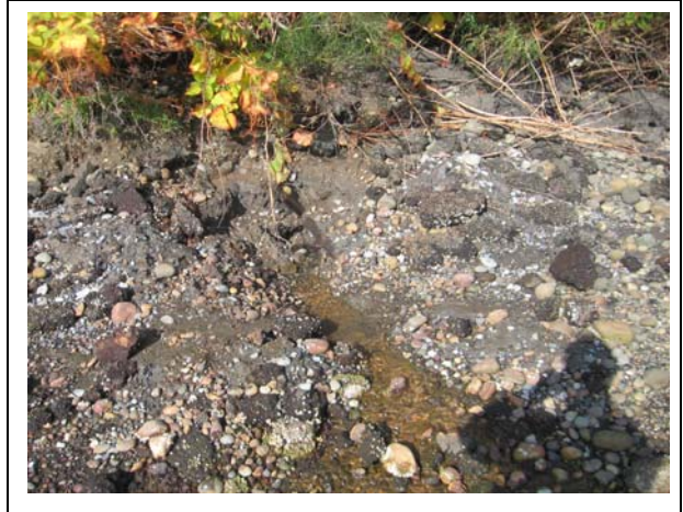
Photo 28. Flume flowing again at same rate four days later after concrete was placed in the pit in Photo 27.
