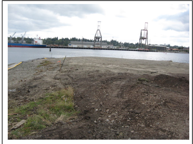
Photo 20. Remediation completed at Area D looking east.
