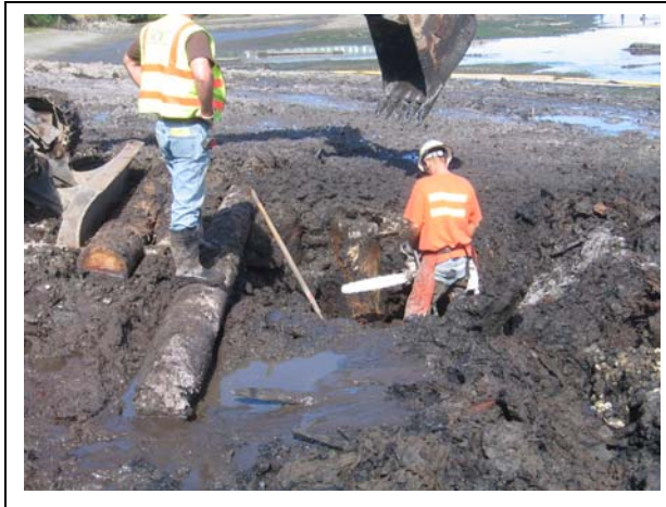
Photo 23. Pilings cut two feet below mudline with a chainsaw, looking north.
