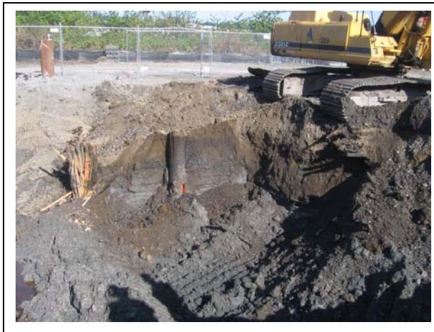
Photo 3. Excavating Area A looking southeast.
