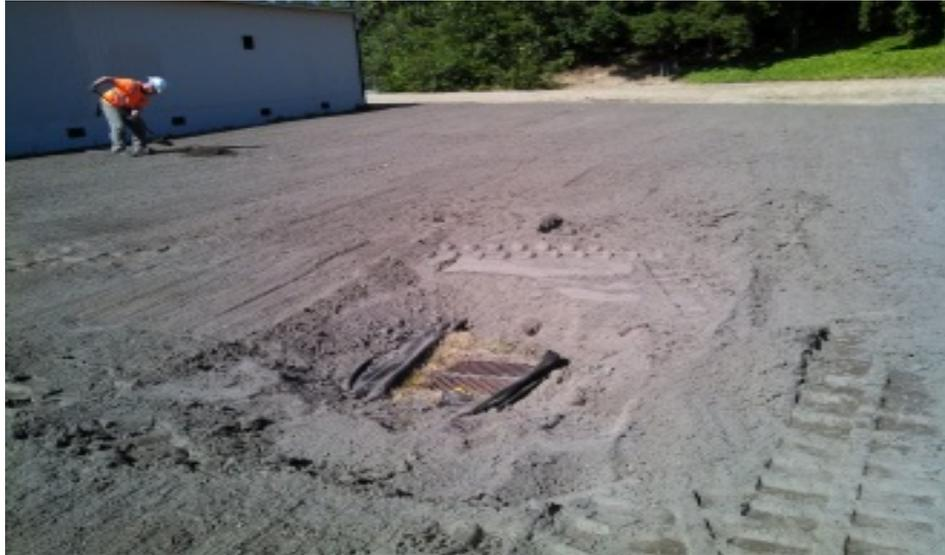
Photograph 1 – Grading of additional soil cover in the North Landfill Area on August 8, 2013. Note underlying geotextile fabric and pre-existing catch basin in foreground.
