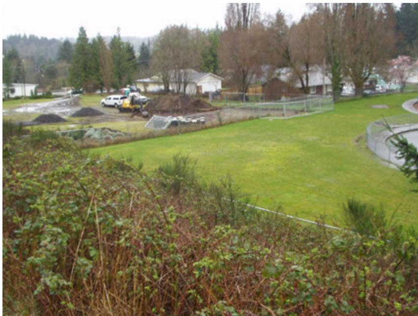
Photograph 2 – Excavation in progress on March 30, 2012. Note the two piles of quarry spalls to the left (east) of the excavation. These rocks were spread over the mud for better truck access to site. The barrels shown in this photo were removed with contaminated material.
