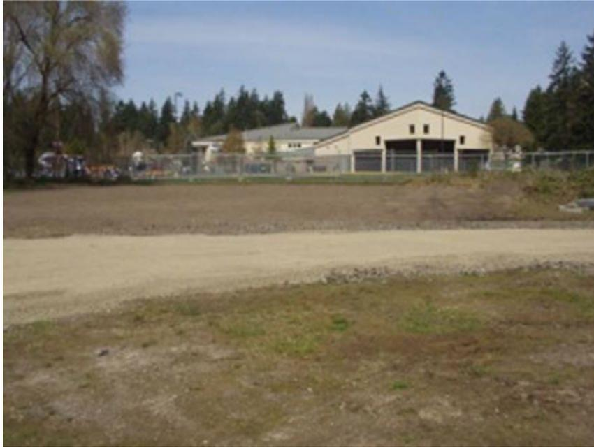
Photograph 11 – This photo taken on April 10, 2012 showing applied topsoil and ¾” minus gravel that has been spread and compacted on road/driveway running through site. This gravel was laid directly on top of quarry spalls laid down for truck access.
