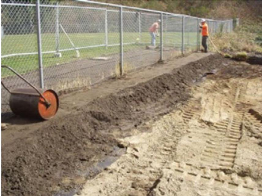
Photograph 7 – Photo taken on April 5, 2012 of the compaction of topsoil over geotextile fabric. Sod was laid on top of this topsoil.
