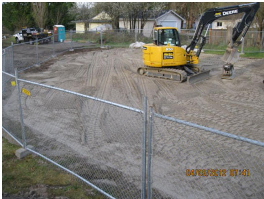
Photograph 10 – Security (fence around entire excavation extent) of site on April 5, 2012. This picture was taken from atop the pile of topsoil. A few inches of topsoil was spread over the compacted pit run fill. Note the compactor under the excavator bucket.
