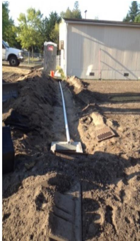
Photograph 2 – Installation of new storm drain line from northeast corner of portable classroom (North Landfill Area) to pre-existing catch basin on August 8, 2013.
