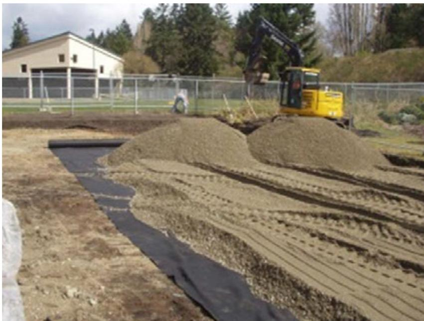
Photograph 8 –Spreading of pit run over geo-textile fabric on April 4, 2012. This material was compacted prior to the application of topsoil and hydroseed.
