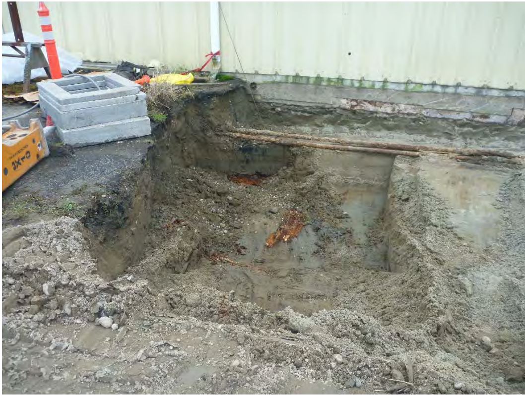
Photograph 11. Area G-1B After Removal of Roof Drain Cistern.
