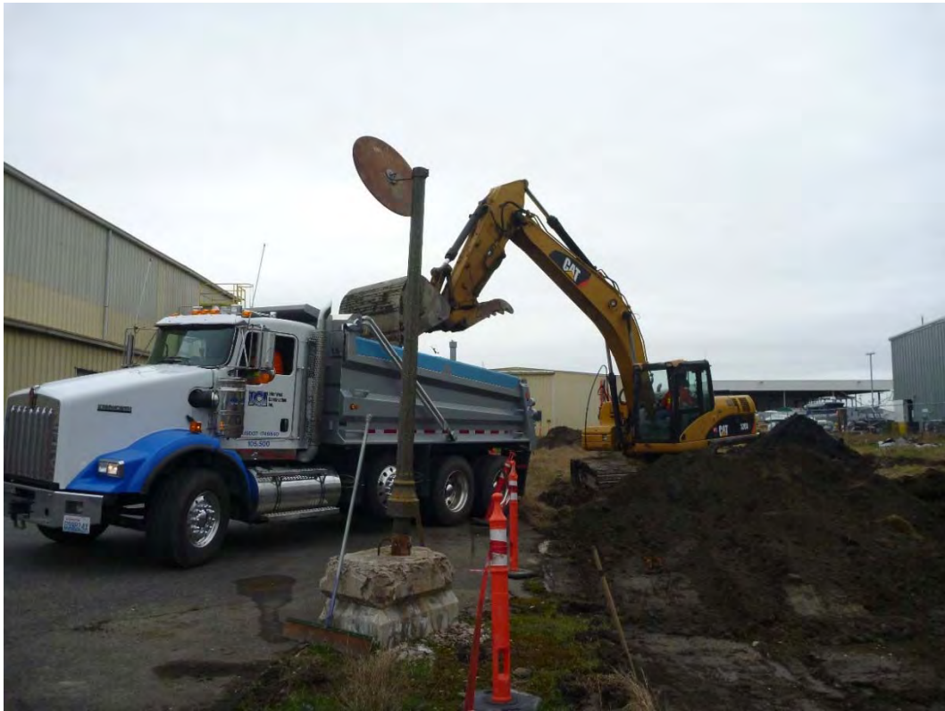
Photograph 1. Direct Loading Excavated Soil for Disposal.
