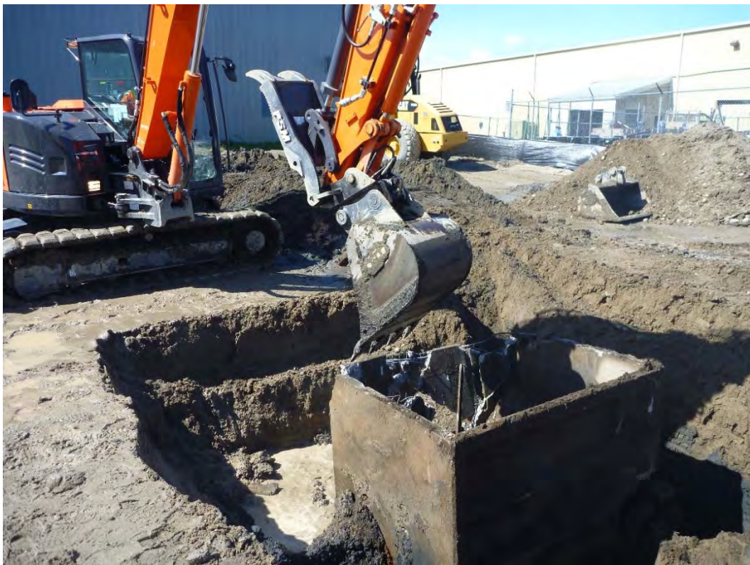
Photograph 12. Excavation For Removal of Former SD8.
