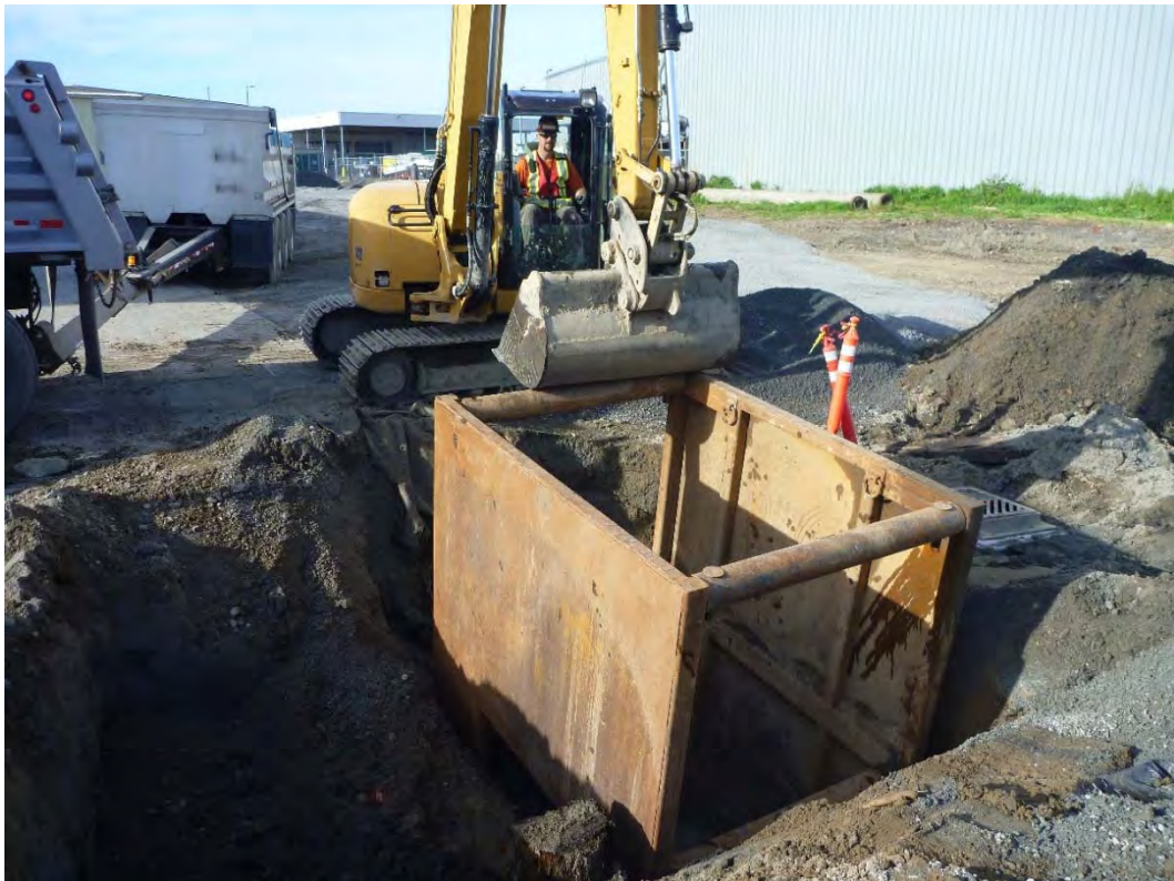
Photograph 19. Connection of Existing Drain to New Storm Drain System.
