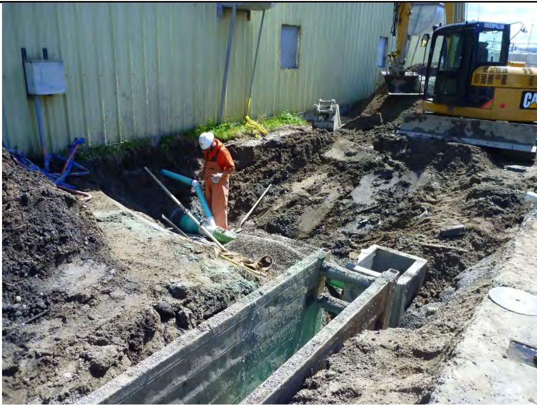
Photograph 19. Connection of Existing Drain to New Storm Drain System.
