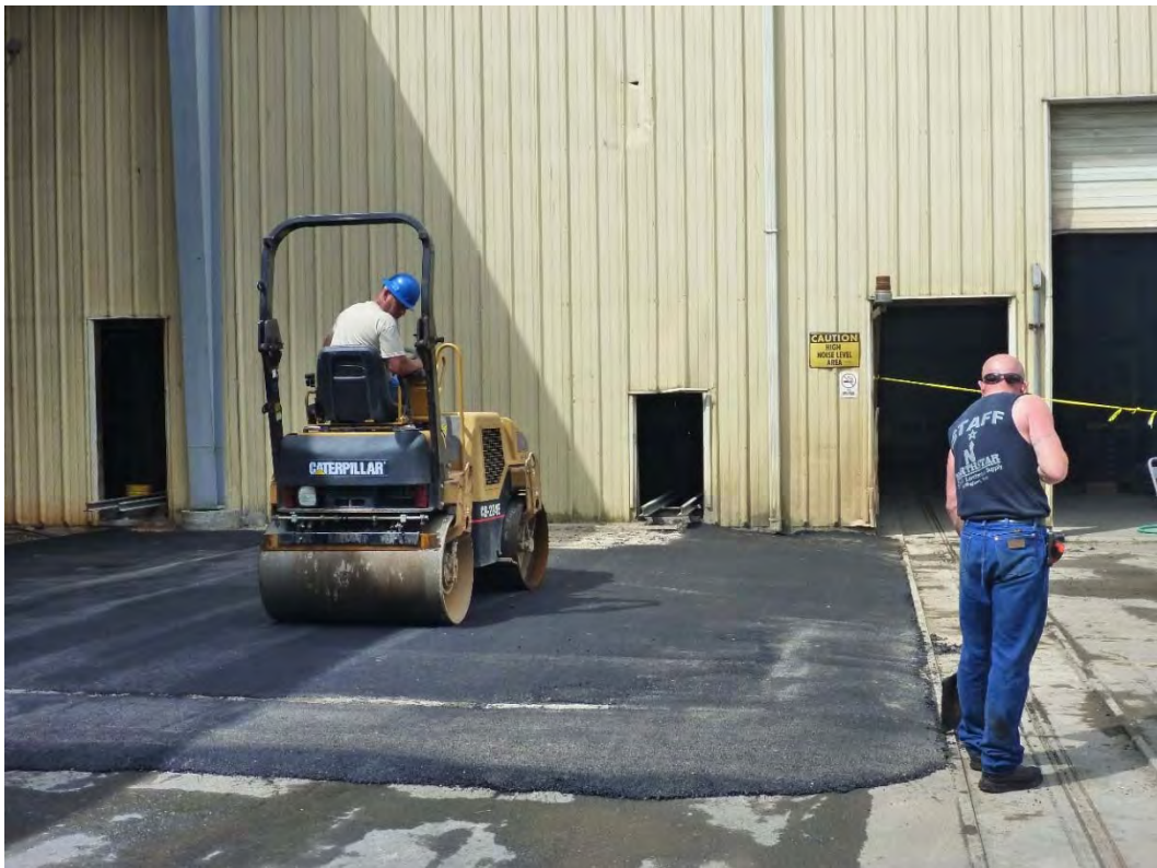
Photograph 22. Paved Finished Surface at Area G-3.
