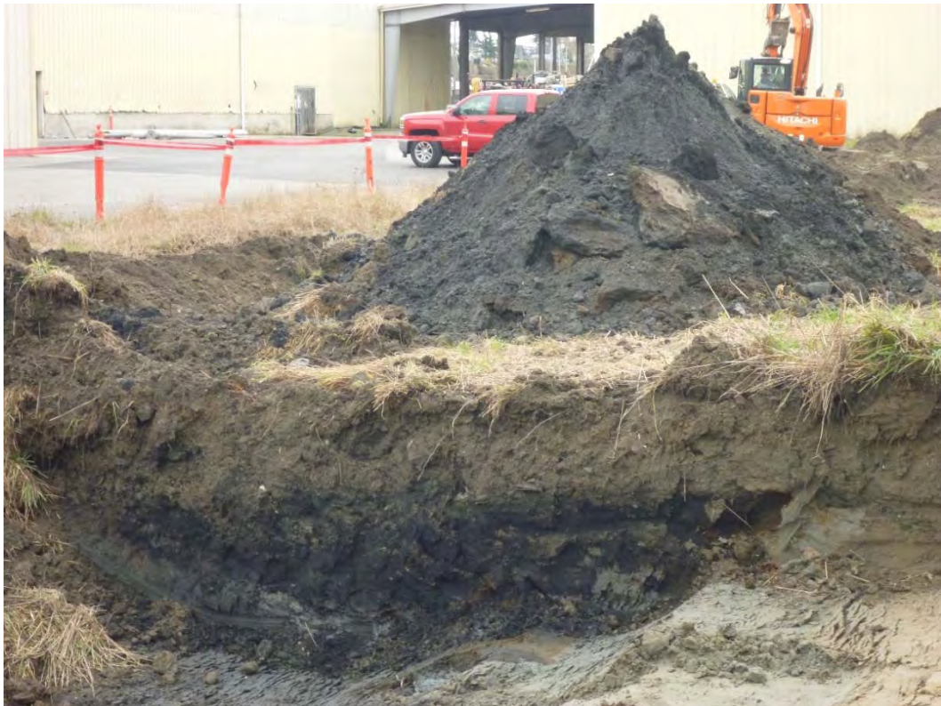
Photograph 2. Sandblast Grit Material in Area G-1B Excavation Sidewall.
