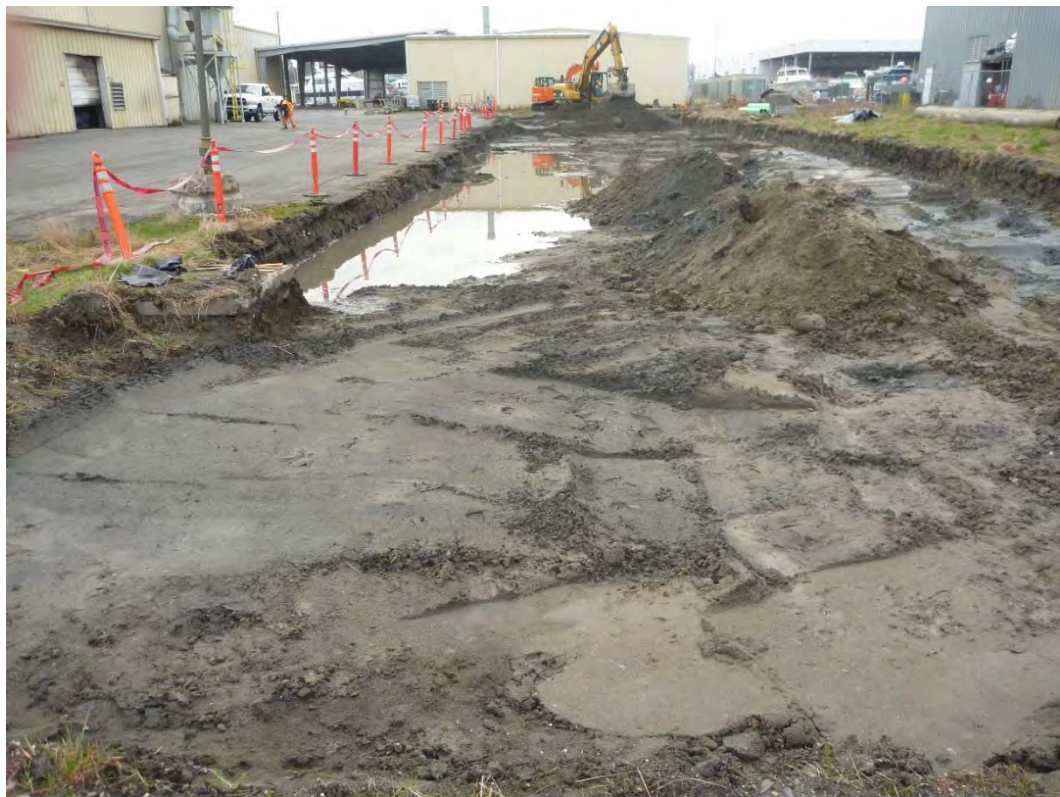
Photograph 4. Finished Extent of Area G-1B Initial Excavation.
