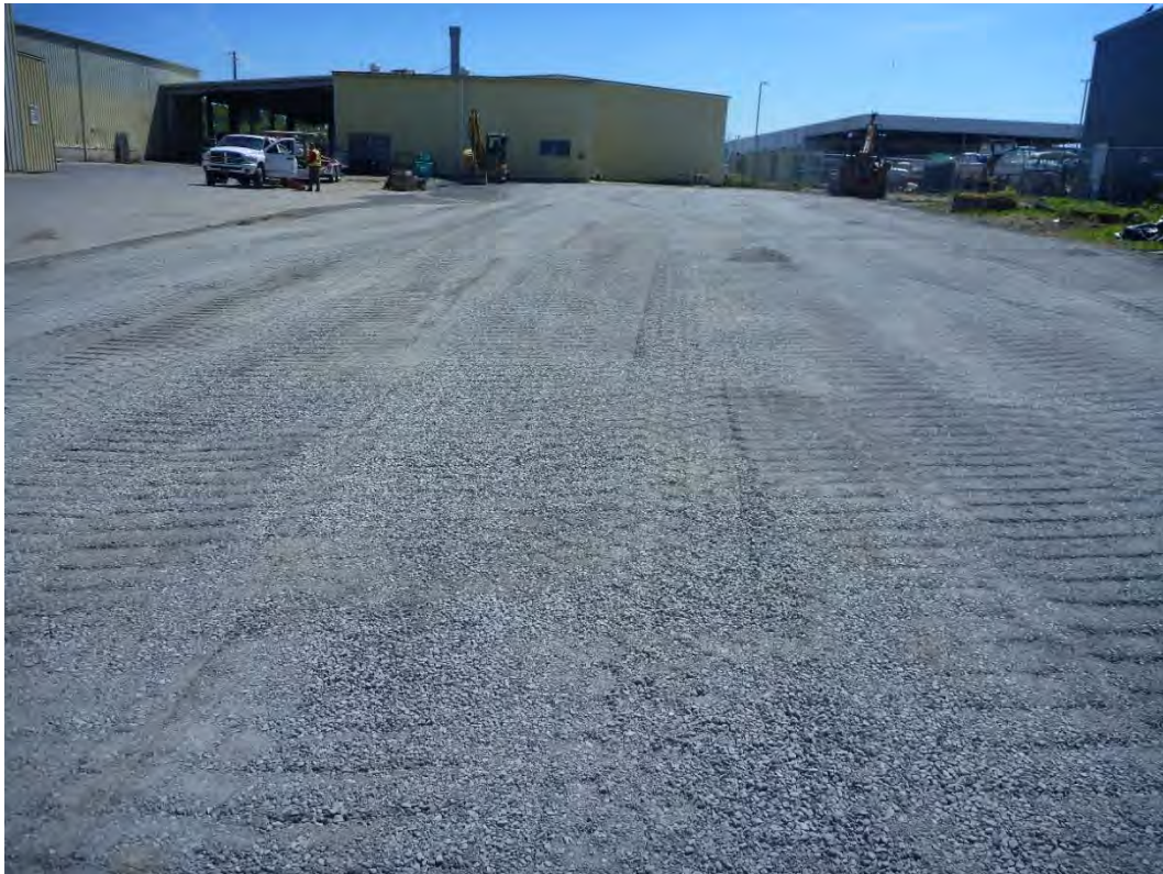
Photograph 21. Graded and Compacted Finished Surface of Area G-1B.
