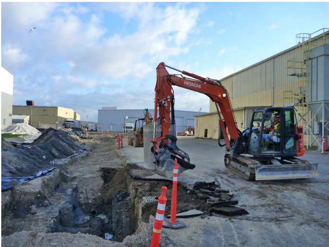
Photograph 16. Beginning Excavation of Former SD9.
