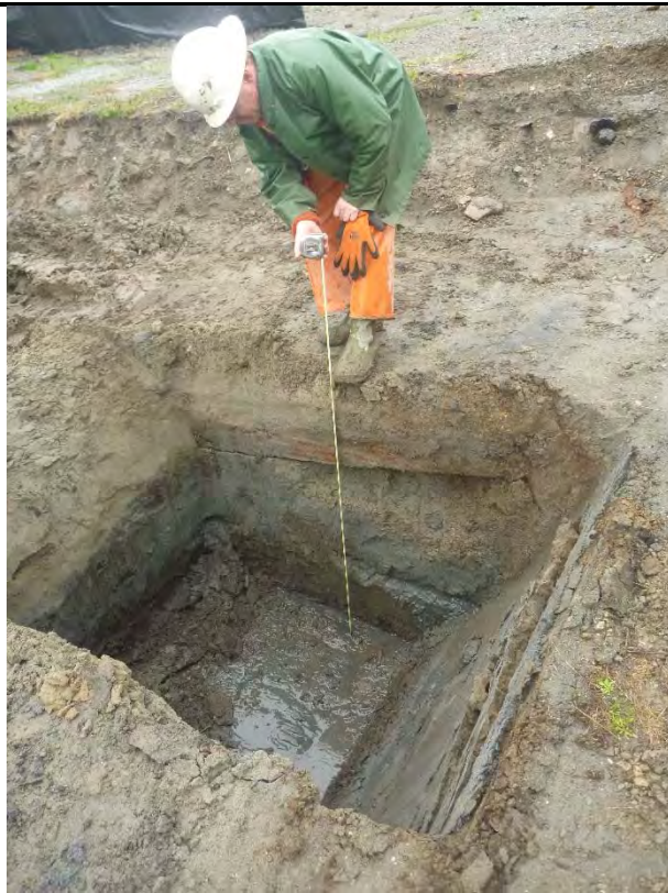
Photograph 3. Typical HA Sample Location Test Pit.
