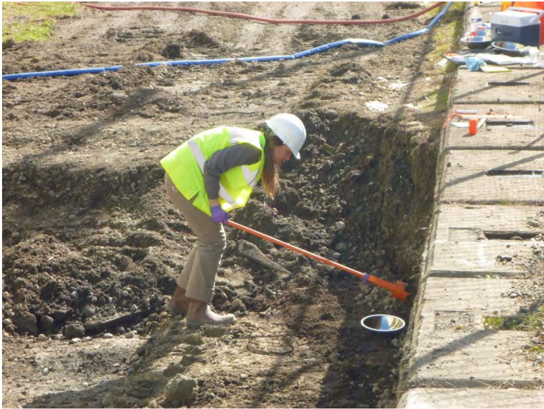
Photograph 5. Typical Sidewall Confirmation Sample Collection Procedure.
