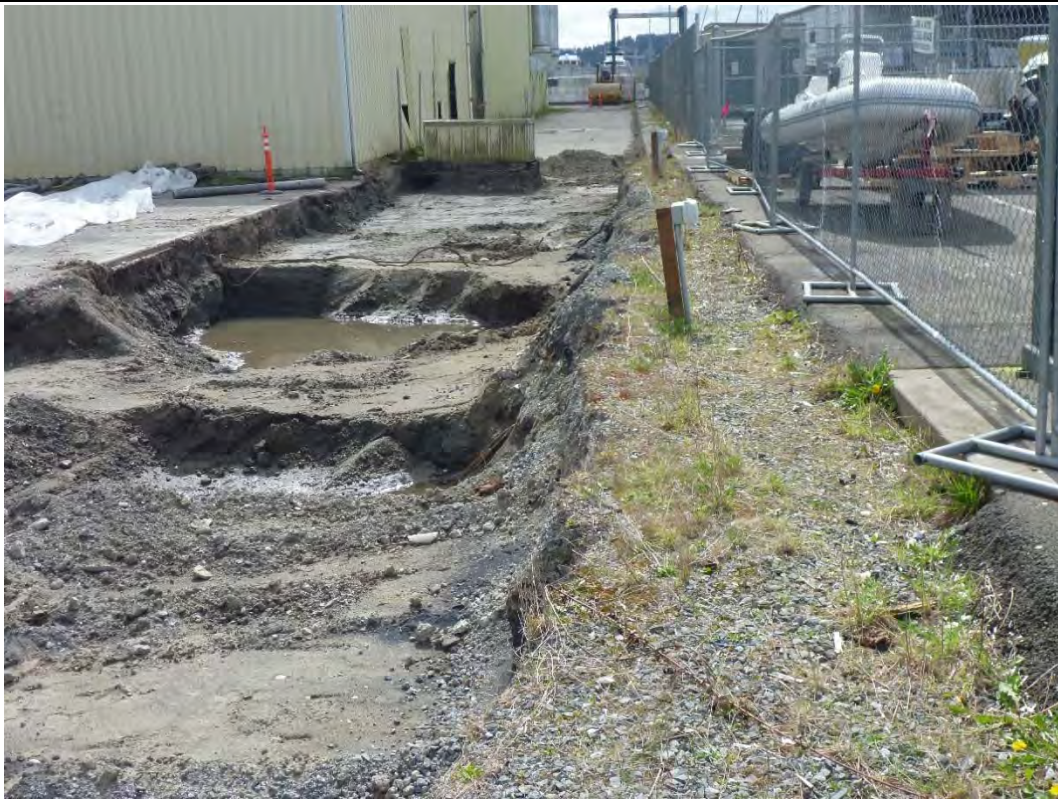
Photograph 9. 'Pothole' Test Pit in Southern Portion of Area G-1B.
