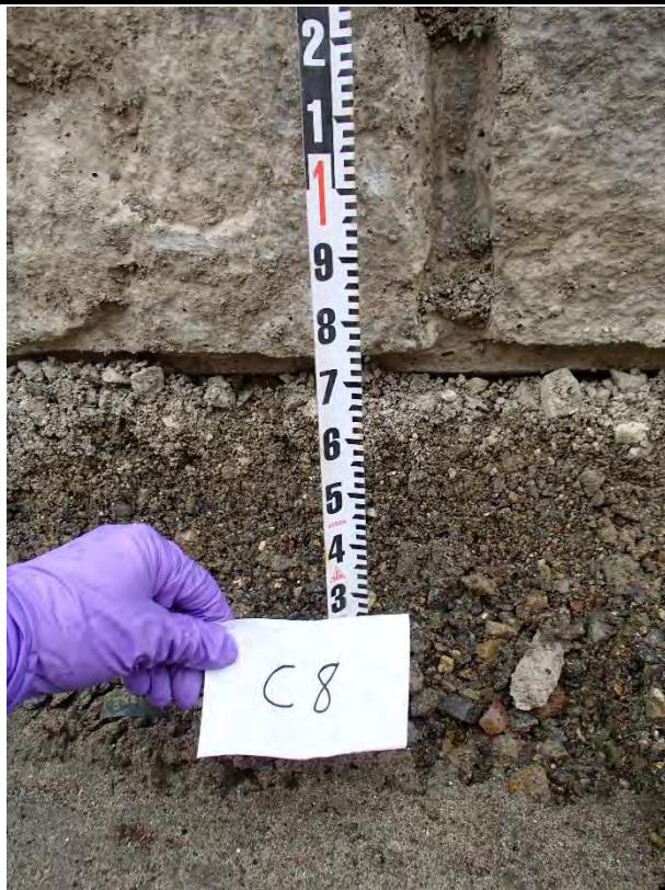
Photograph 7. New Base Course from Area J-3 Interim Action Encountered at G1B-C8.
