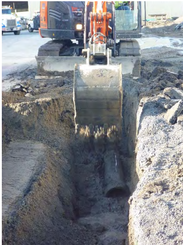
Photograph 18. Removal of Former Storm Drain Pipe South of Former SD8.
