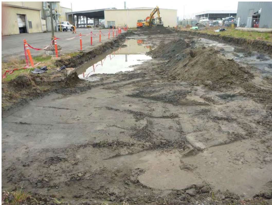
Photograph 4. Finished Extent of Area G-1B Initial Excavation.
