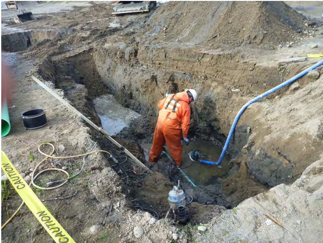
Photograph 13. SD8 Area Pit After Excavation.
