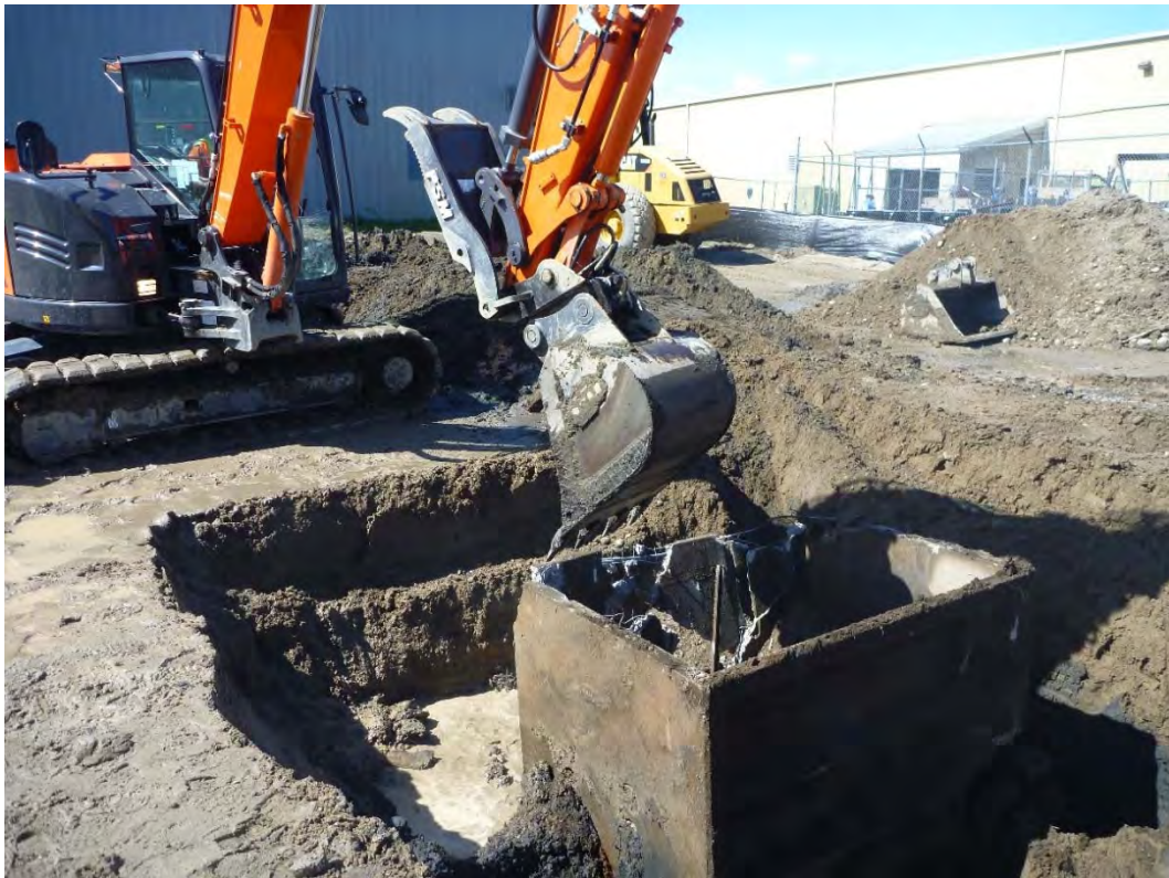
Photograph 12. Excavation For Removal of Former SD8.
