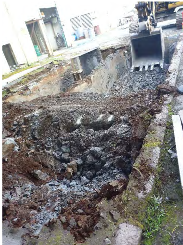
Photograph 10. Excavation of Area G-3 Former Settling Pond.
