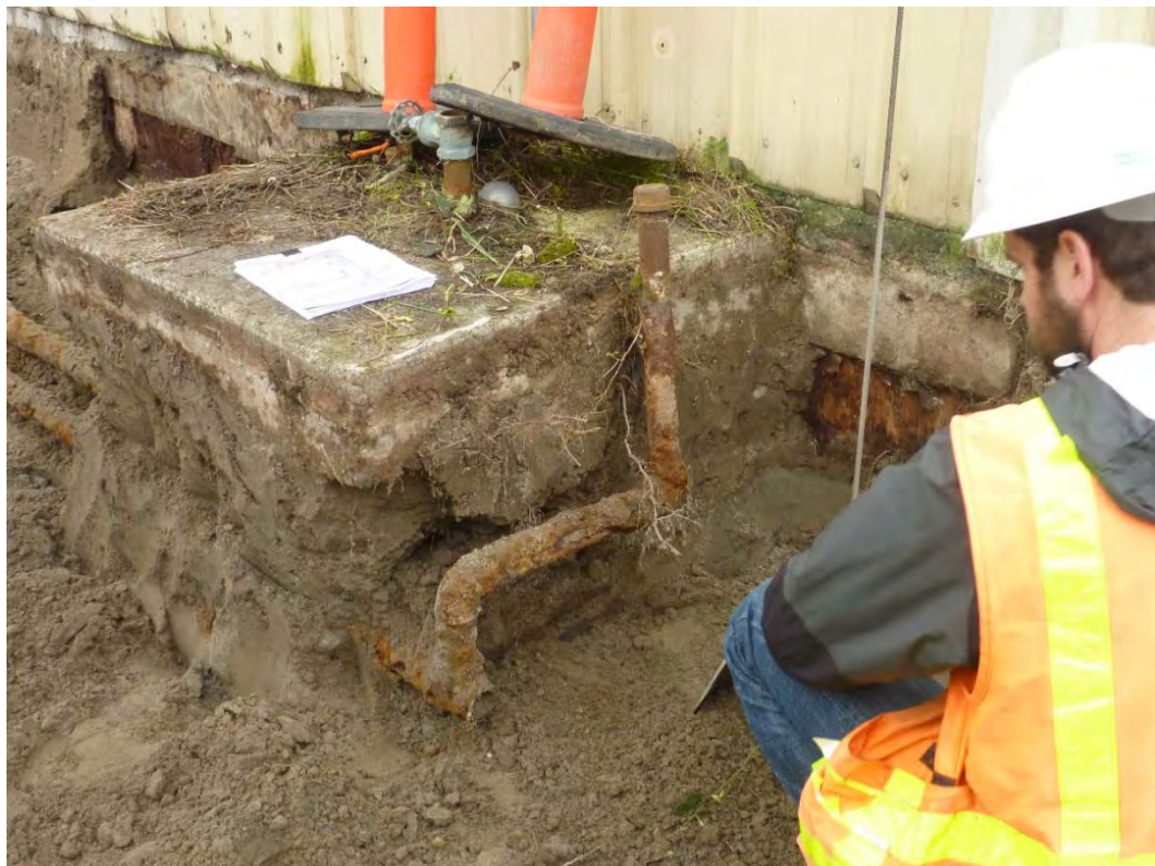
Photograph 8. Former Diesel UST Pad and Piping Near Lab Building.
