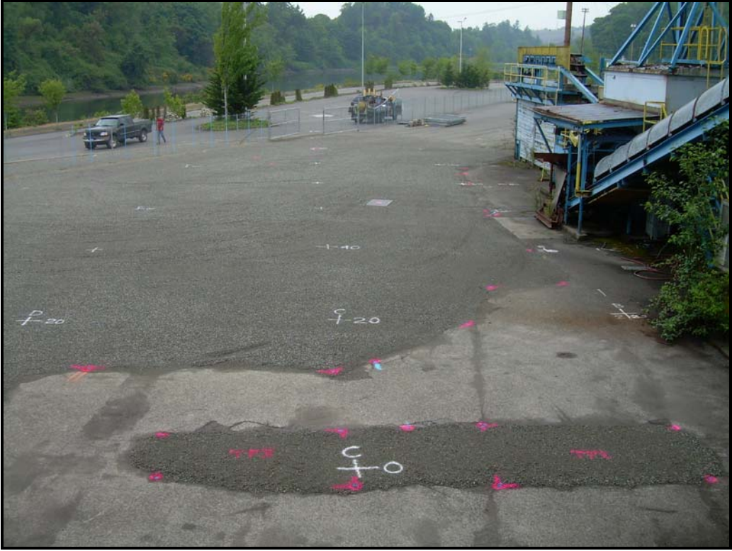
Photo 6B. Site Restoration.
