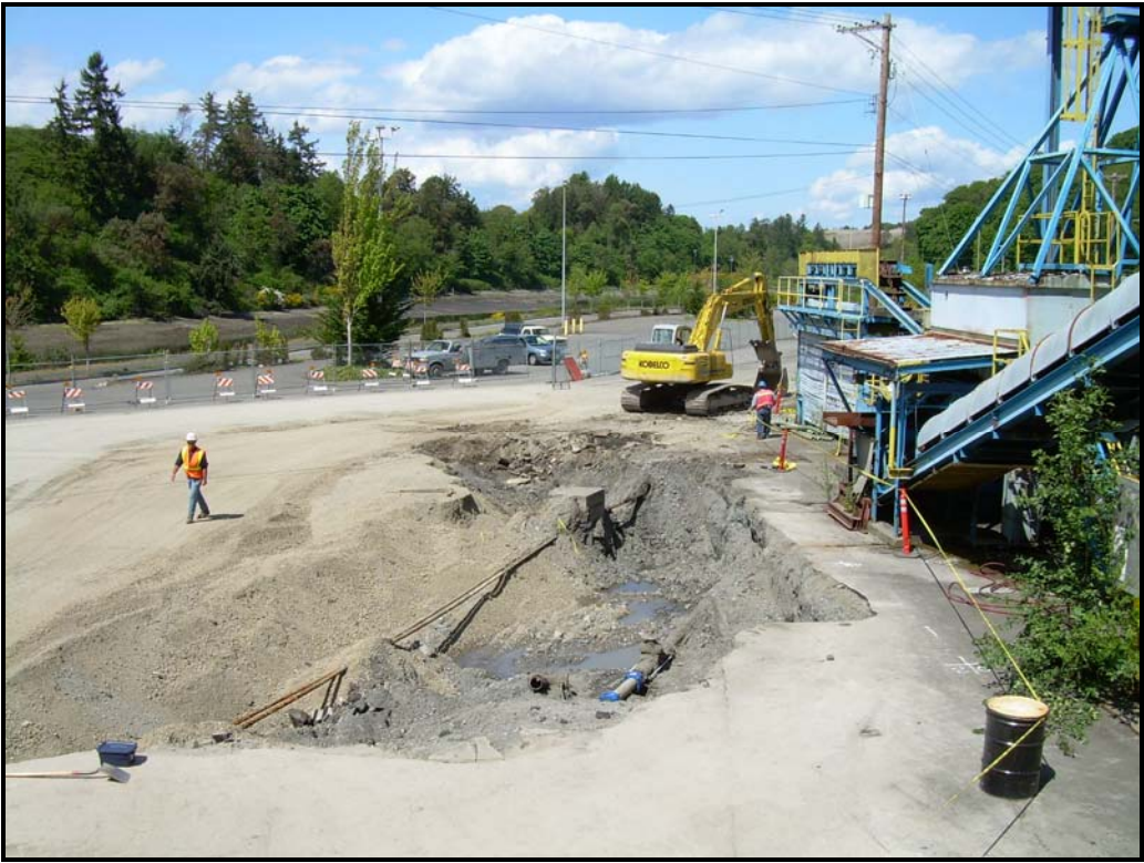
Photo 5. Backfilling.
