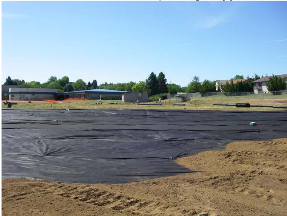
Photo D-1: Robertson Elementary School placing geotextile
