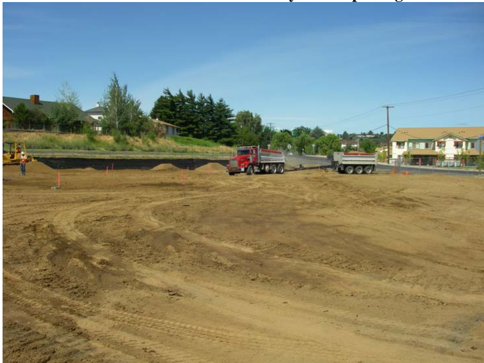
Photo D-2: Robertson Elementary School placing soil
