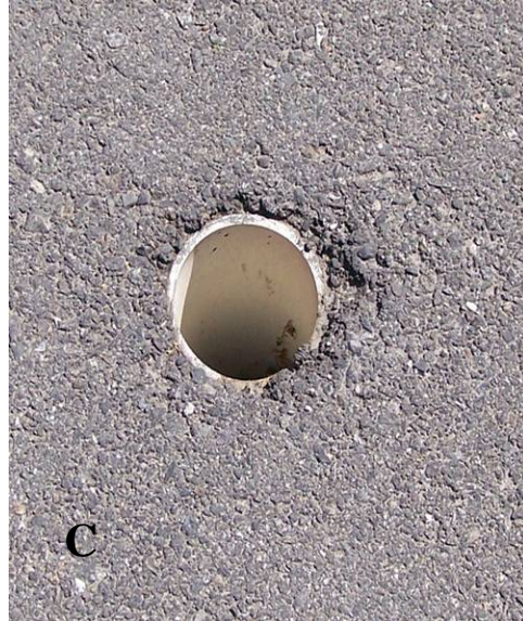
Photos of Leo's Line Up Taken During Site Visit on May 24, 2010. Plate A: Looking South West. Plate B: Ground Water Monitoring Well with Cap. Plate C: Ground Water Monitoring Well without Cap.
