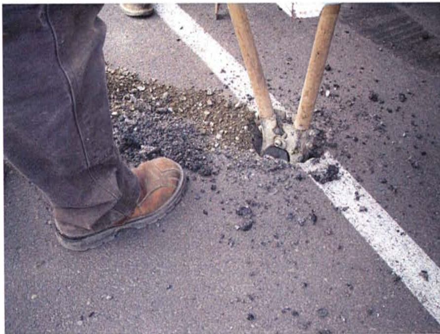
Photograph No. 2: View of hand clearing procedures for soil borings.
