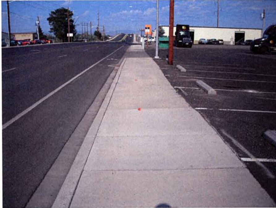
Photograph No. 5: View looking west down West Valley Mall Blvd. Note MW-01 is located in the right center of the photograph. Existing subsurface utilities are marked by paint.
