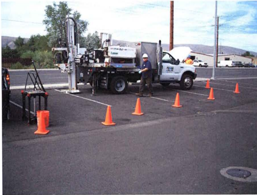
Photograph No. 1: View of the probe rig setting upon SB-01/MW-01 location.
