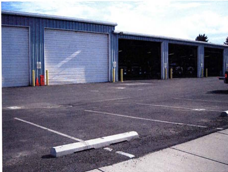
Photograph No. 6: View of the former gasoline underground storage tank (UST) and dispenser area. MW-01 is located to right, MW-02 is located to the left, and MW-03 is located in center background.
