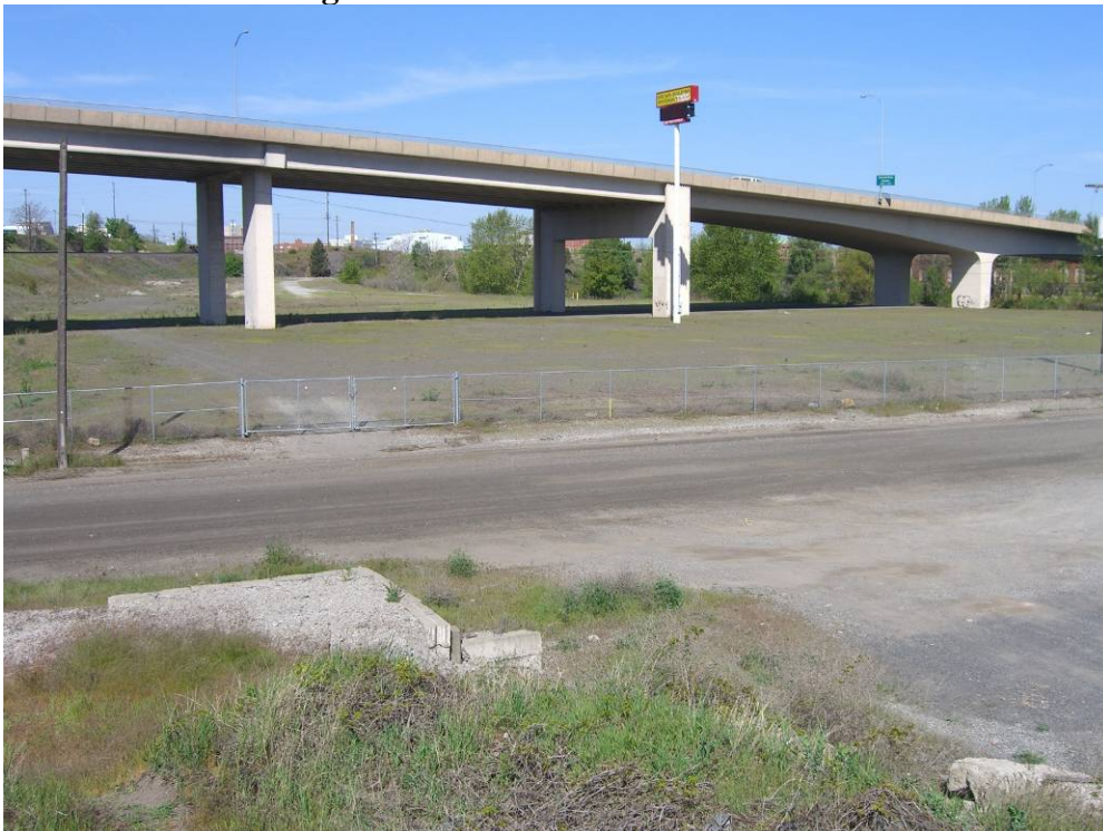
Photo 2: Hamilton Street Bridge Site – from the east
