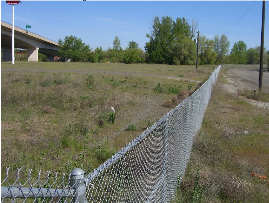
Photo 4: Site Perimeter Fencing - from the south
