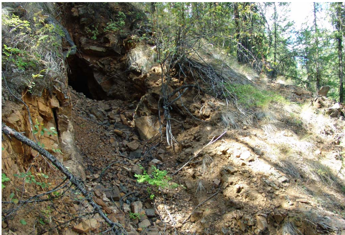
Upper portal is located high on the slope above the creek, and has collapsed.
