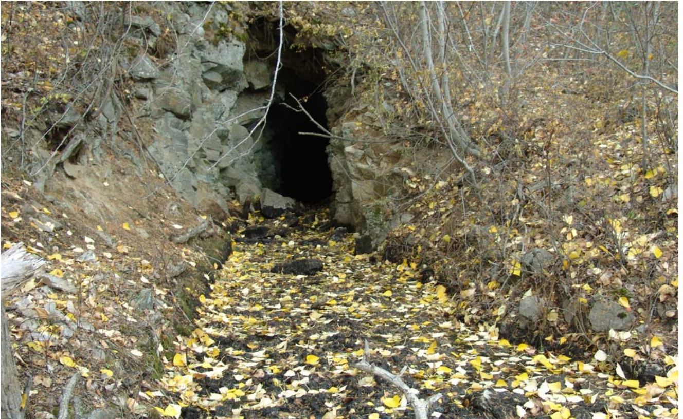
Lower mine portal on the Security claim, with drainage from the adit.
