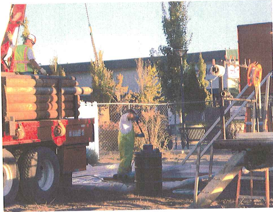
Photo 3: Photograph of drill equipment decontamination process over containment area.
