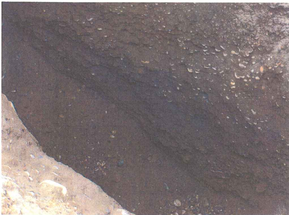
Photo 4: Photograph of northern drywell excavation progress during second cleanup event.
