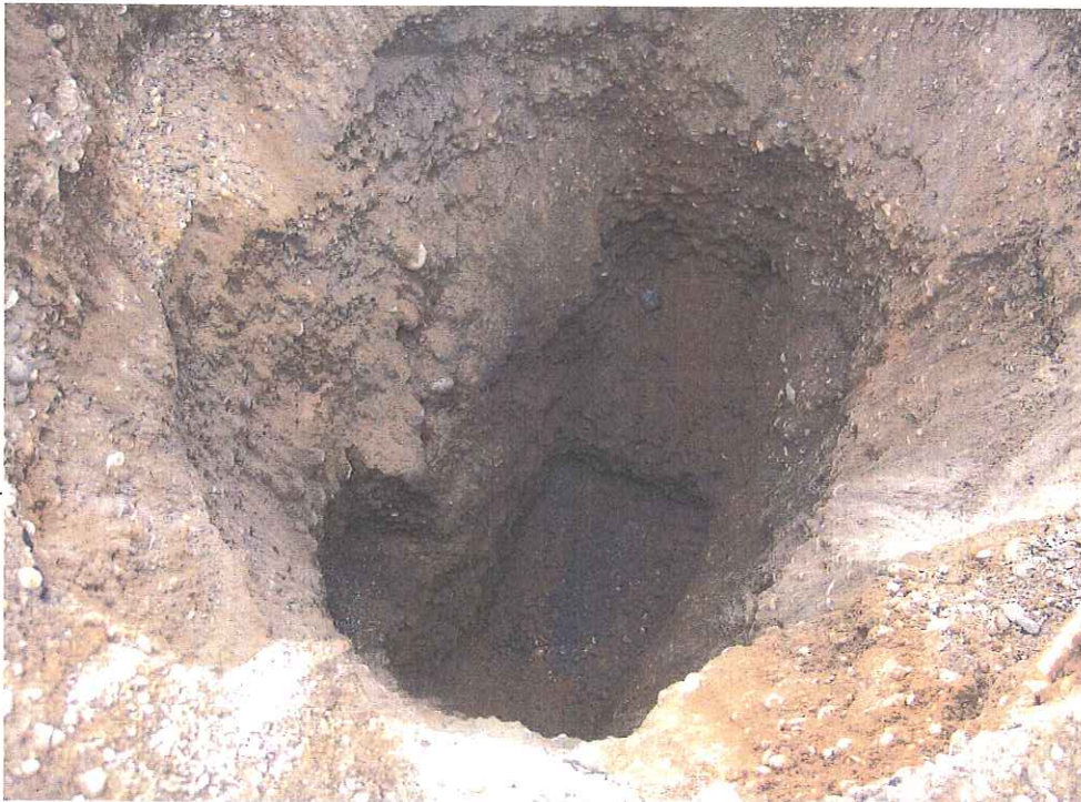
Photo 6: : Photograph of northern drywell excavation progress during second cleanup event.
