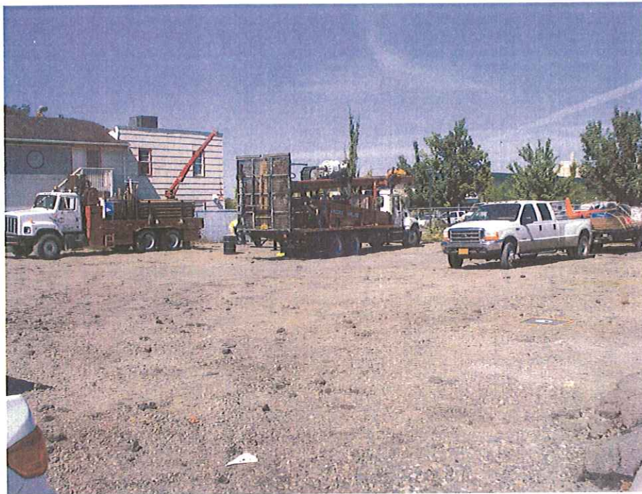
Photo 1: Photograph of northern portion of Site during drilling mobilization.
