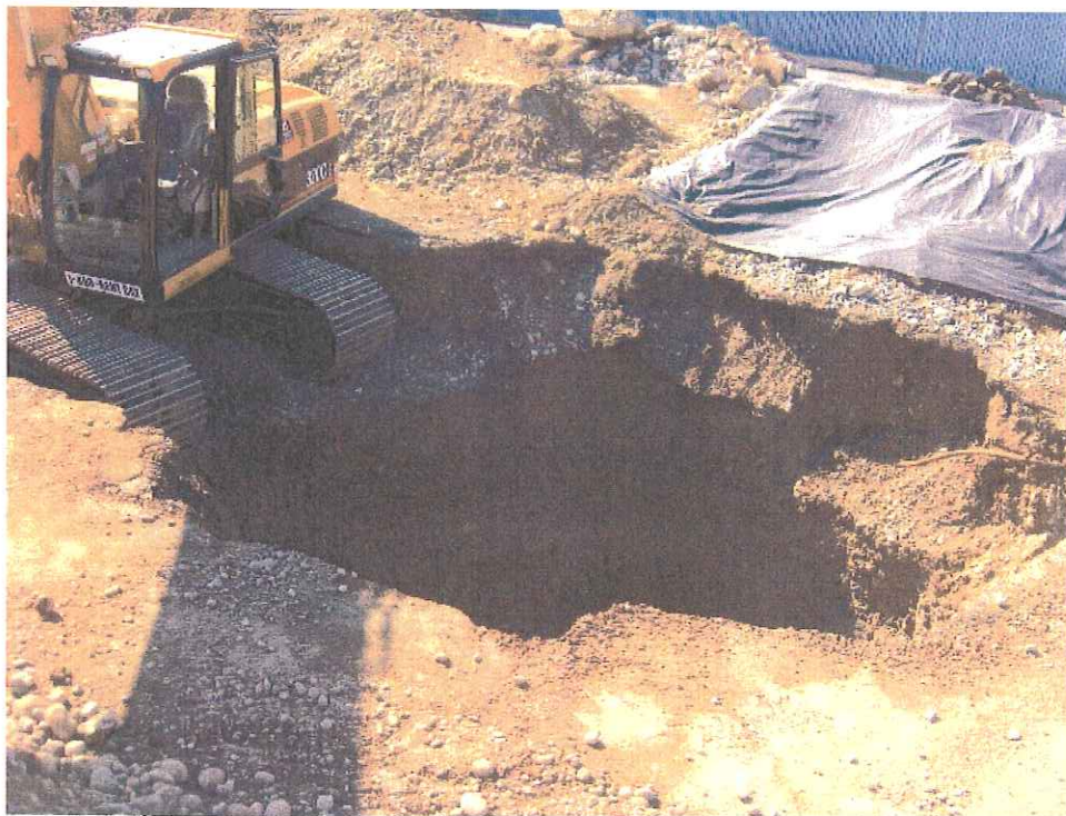
Photo 8: Photograph of northern drywell excavation at final surface dimension and limit.
