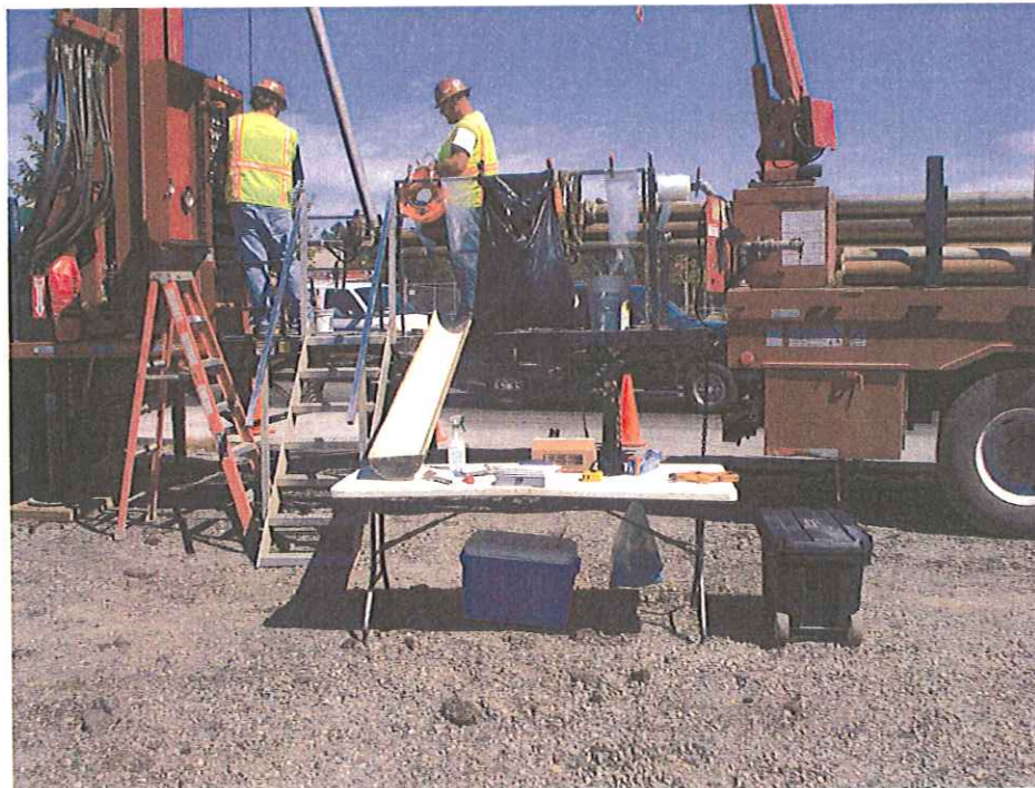
Photo 2: Photograph of drill rig setup.
