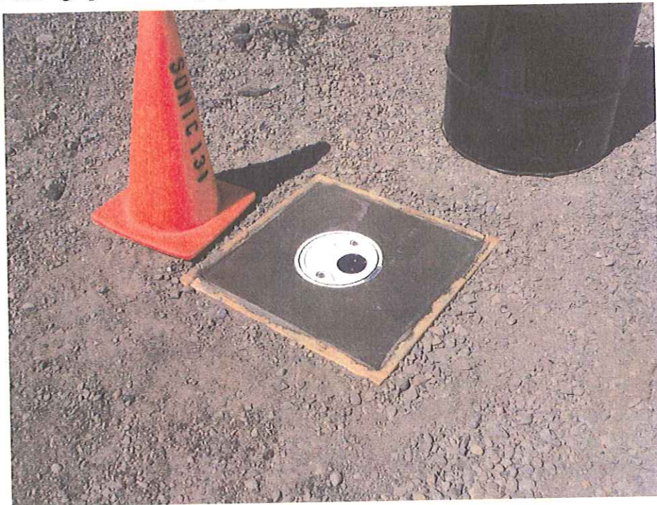
Photo 4: Photograph of typical monitoring well surface construction.
