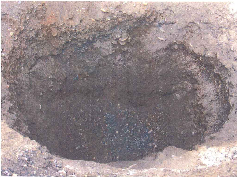
Photo 5: Photograph of northern drywell excavation progress during second cleanup event.
