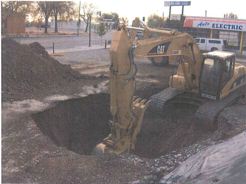
Photo 1: Photograph of northern drywell remedial excavation area.
