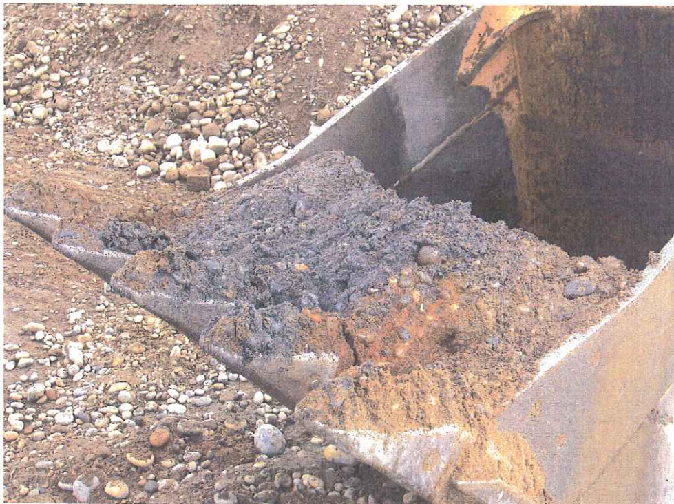
Photo 3: Photograph of obvious discolored (gray) soil removed from remedial excavation.
