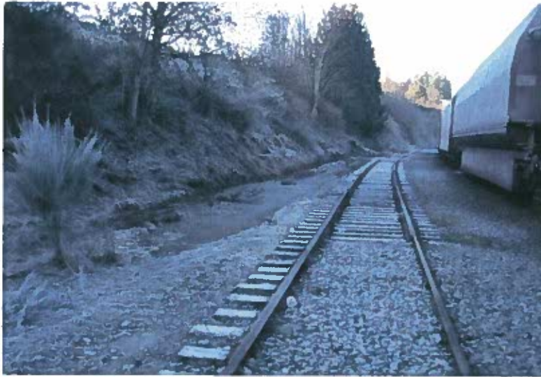
Photo 11. Stormwater drainage ditch along railroad tracks prior to excavation.
