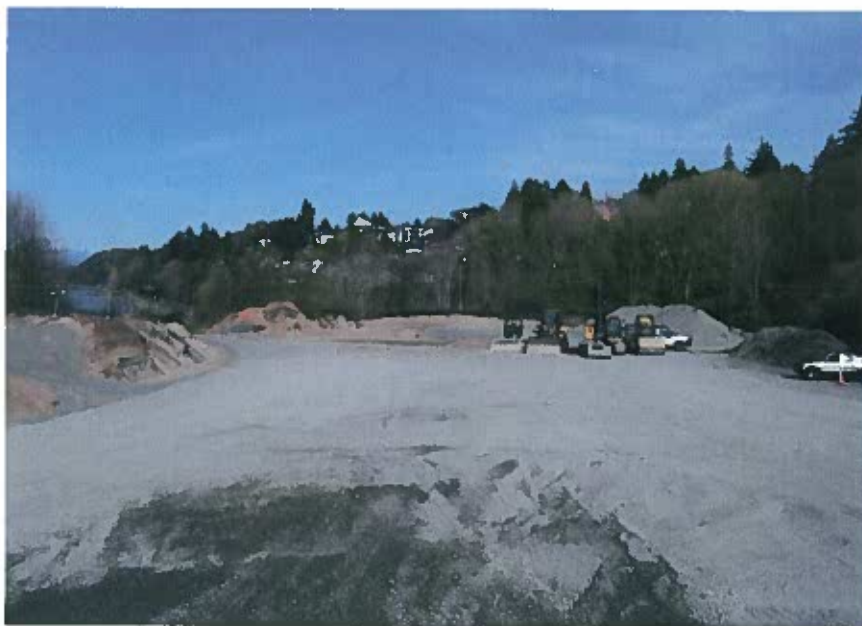
Photo 10. Western to eastern view of site following backfill.
