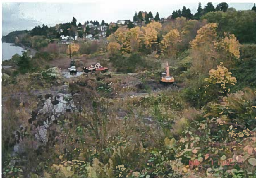
Photo 2. Clearing and grubbing prior to excavation
