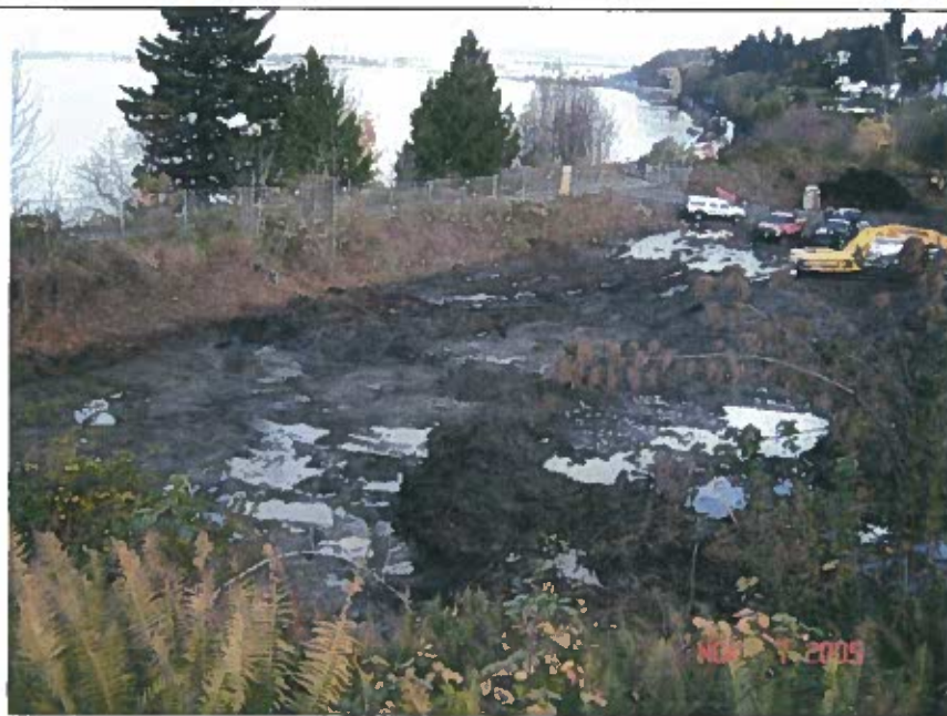
Photo 3. Excavated area in western portion of site.
