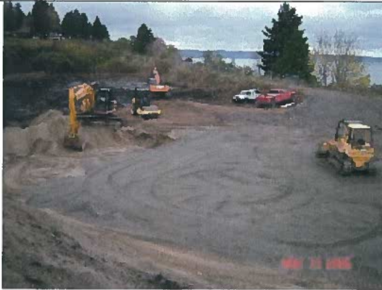
Photo 7. Backfilling area in central portion of site with crushed rock.
