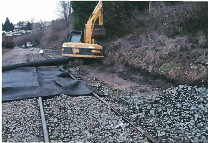
Photo 12. Excavation, geotextile emplacement, and backfilling of stormwater drainage ditch.
