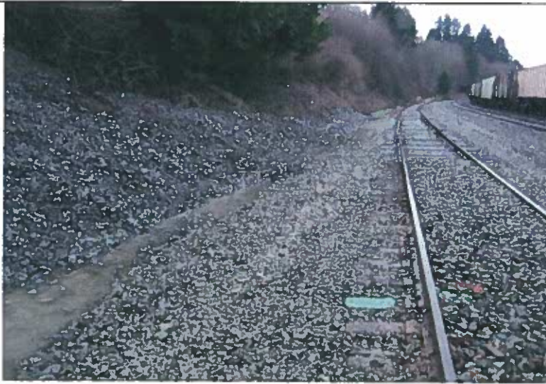
Photo 13. Stormwater drainage ditch after backfill completion
