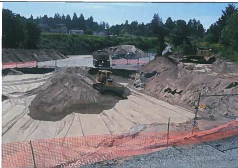
Photo 9. Backfilling of large excavated area in eastern portion of site with native material.
