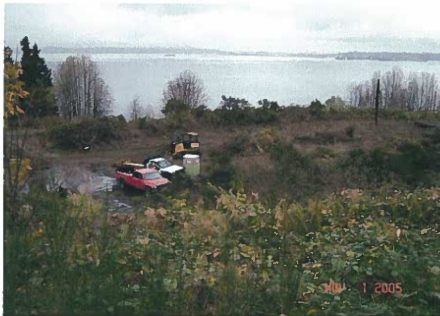
Photo 1. Clearing and grubbing prior to excavation
