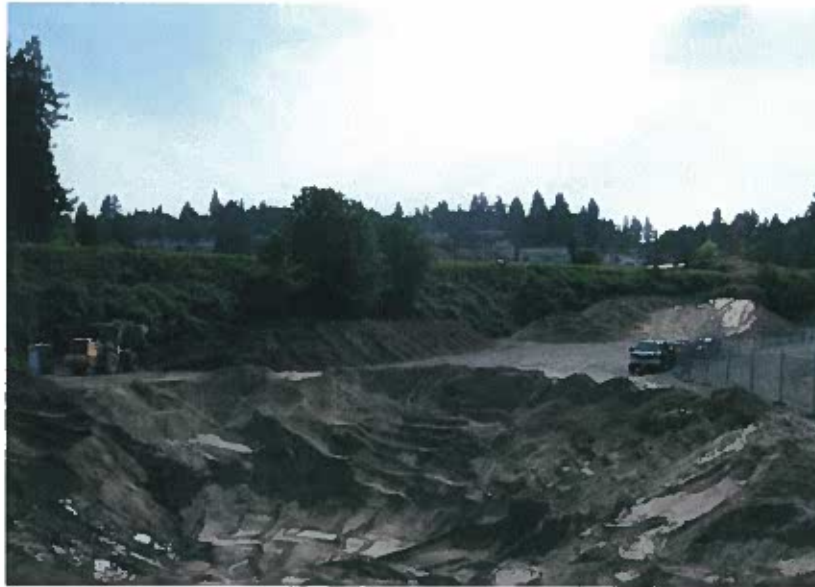
Photo 8. Large excavated area in eastern portion of site.
