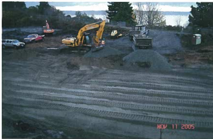
Photo 6. Excavated area in central portion of site.
