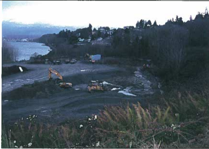
Photo 5. Backfilling with crushed rock in western portion of site.
