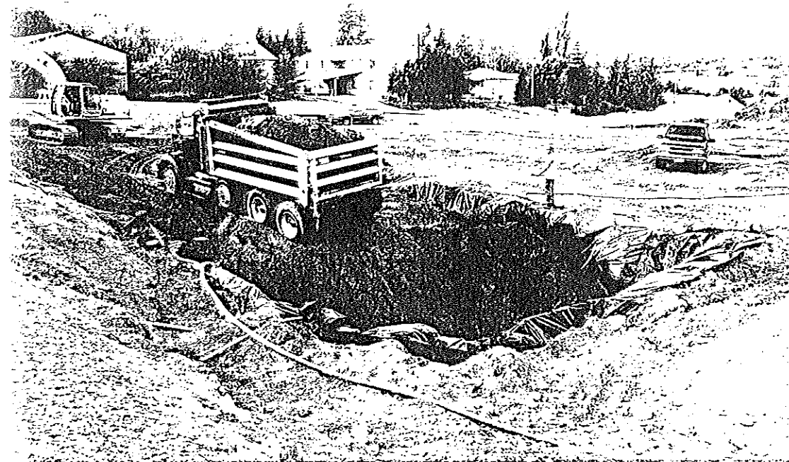
Photograph 9: Completion of northern portion of remediation burial pit.
