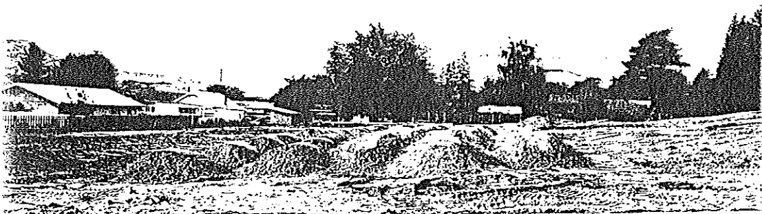
Photograph 14: Western site fill placed on 6 mil visqueen.
