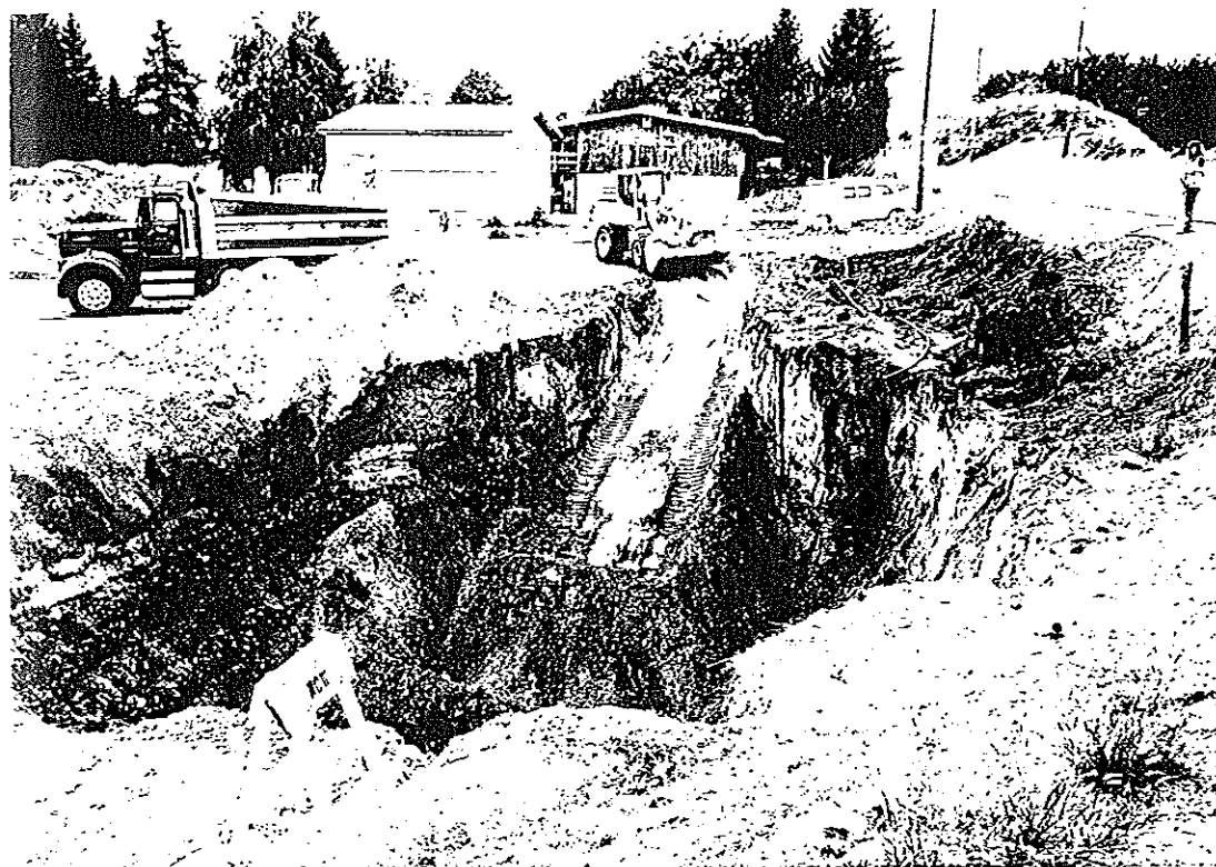
Photograph 5: Excavation of southern section of remediation burial pit.
