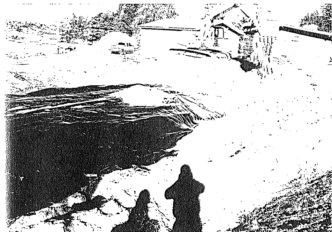
Photograph 10: Covering of remediation burial pit and soil capping.
