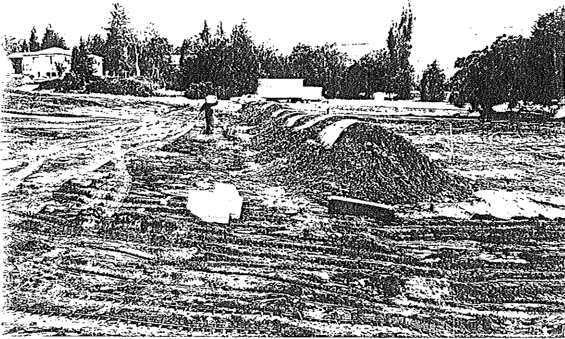
Photograph 13: Western site fill placed on 6 mil visqueen
