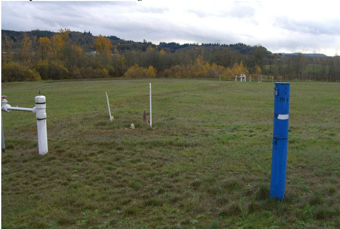
Photo 2: Cap Surface with Monitoring Wells and Gas Collection Points – from the north
