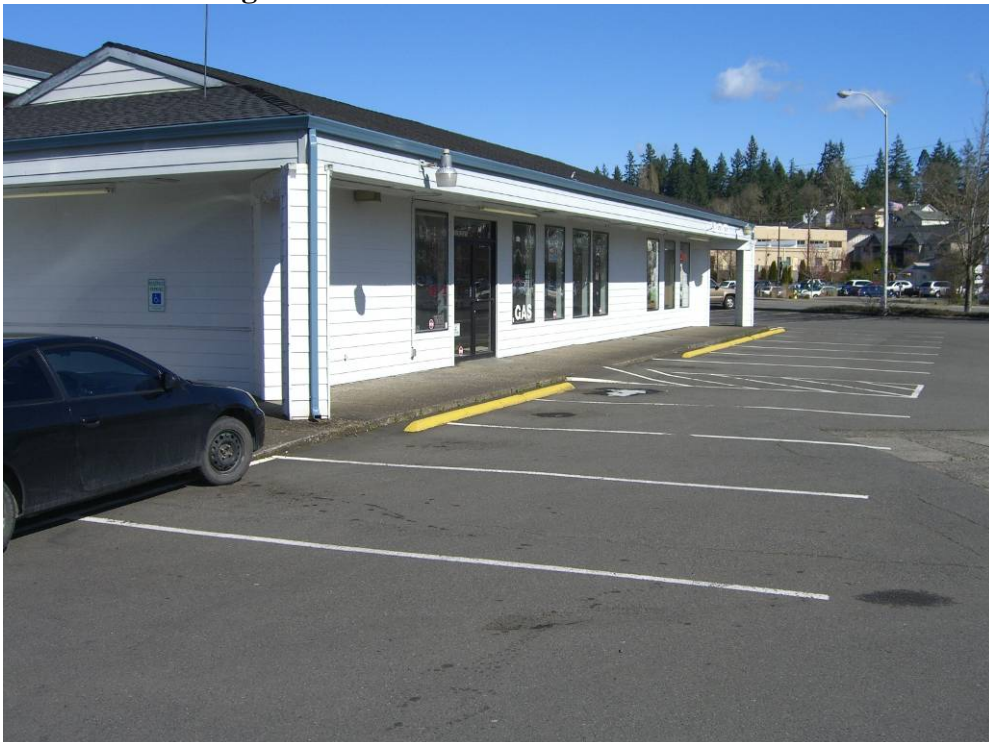
Photo 2: L&C Deli Building – from the west
