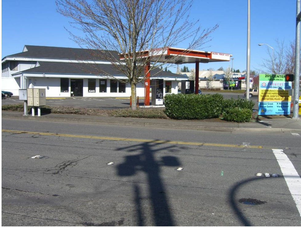
Photo 3: L&C Deli Site - from the west
