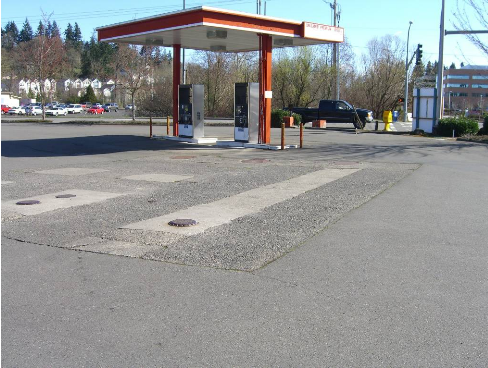
Photo 1: L&C Site Pump Island - from the northeast
