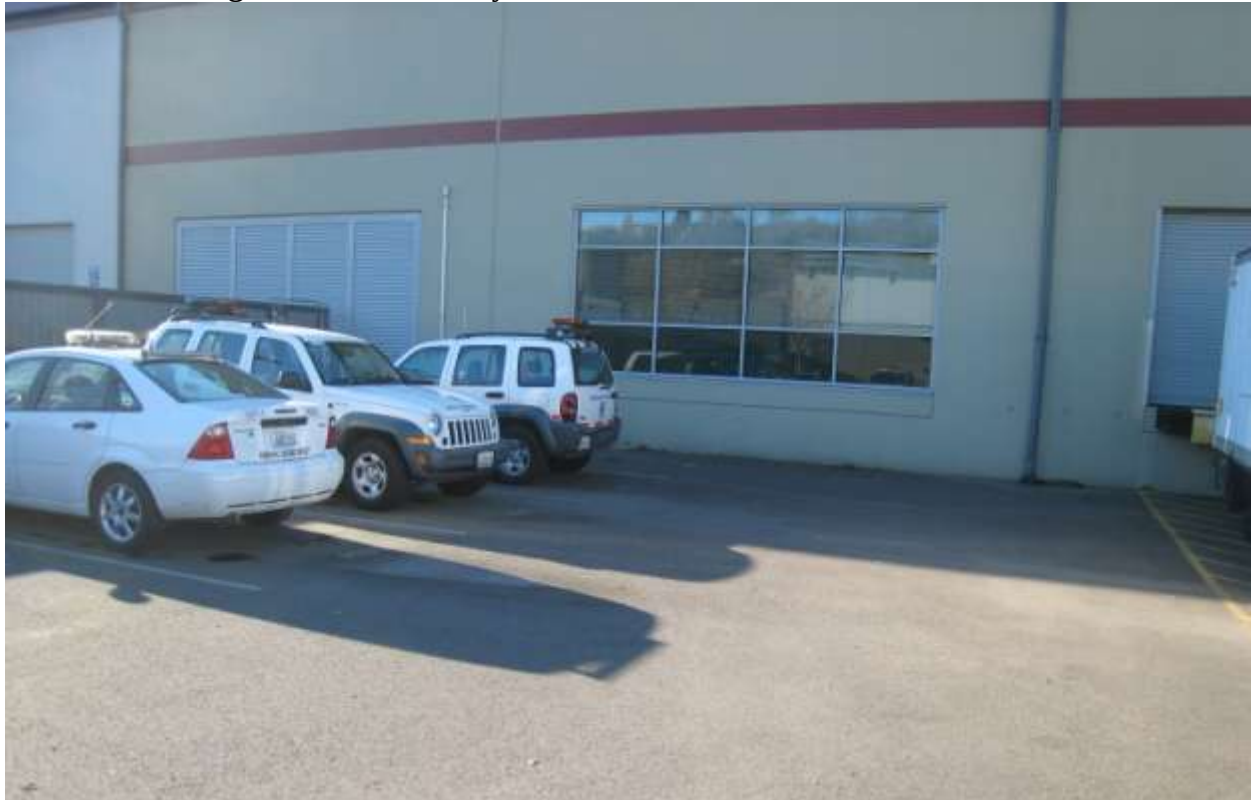
Photo 4: Building C, area covered by covenant – from the east
