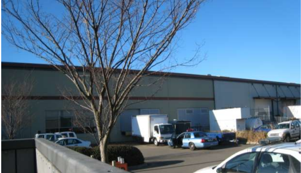
Photo 3: Building C, area covered by covenant - from the southwest corner of Building D
