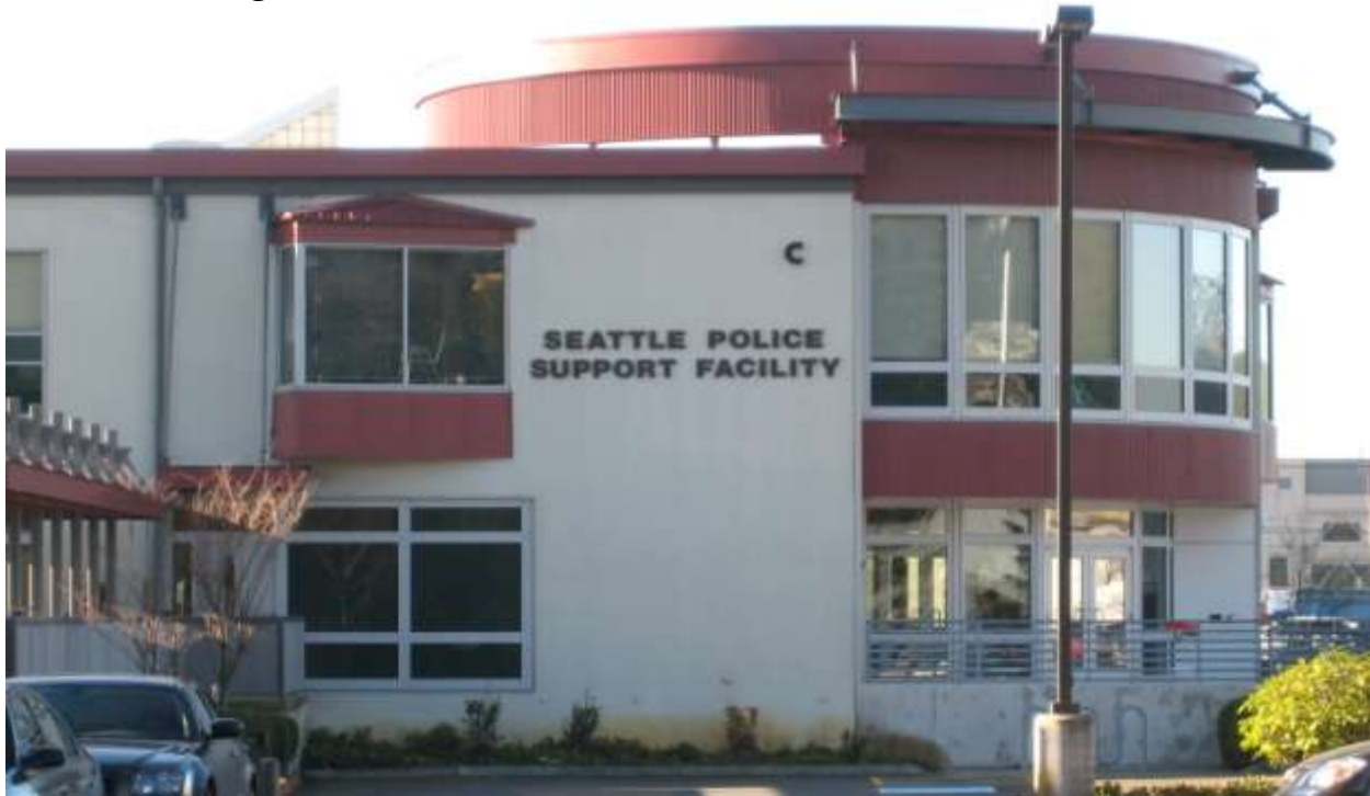
Photo 1: Building C, north end - from the east
