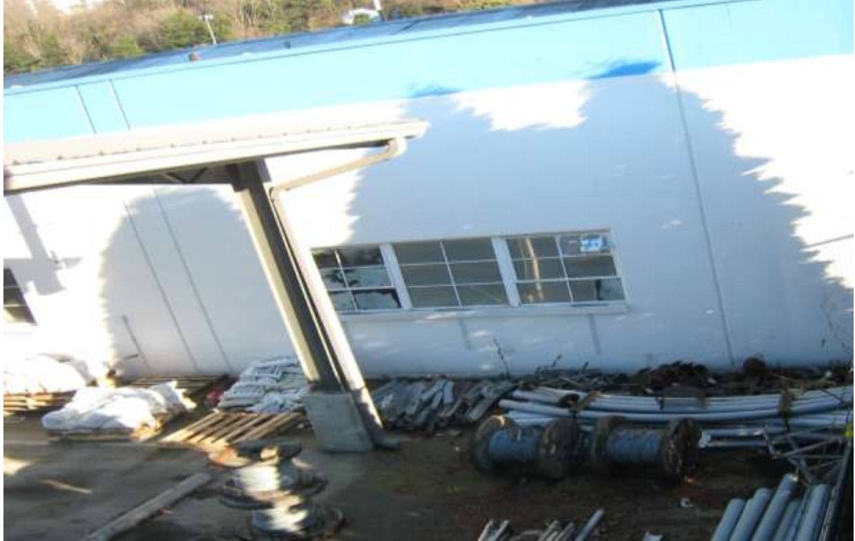
Photo 3: Former waste oil tank location near building at right
