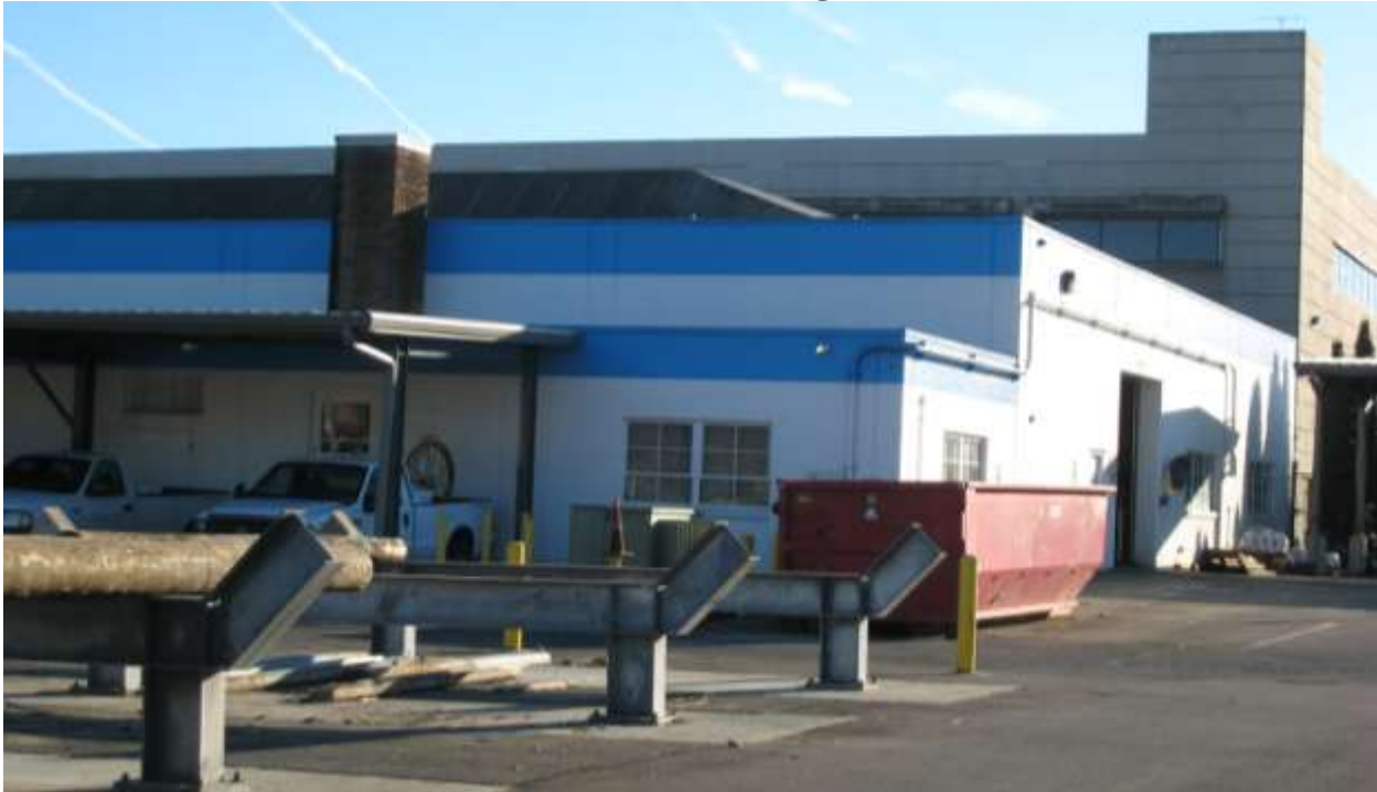
Photo 1: Former tank locations near corner of building - from the north
