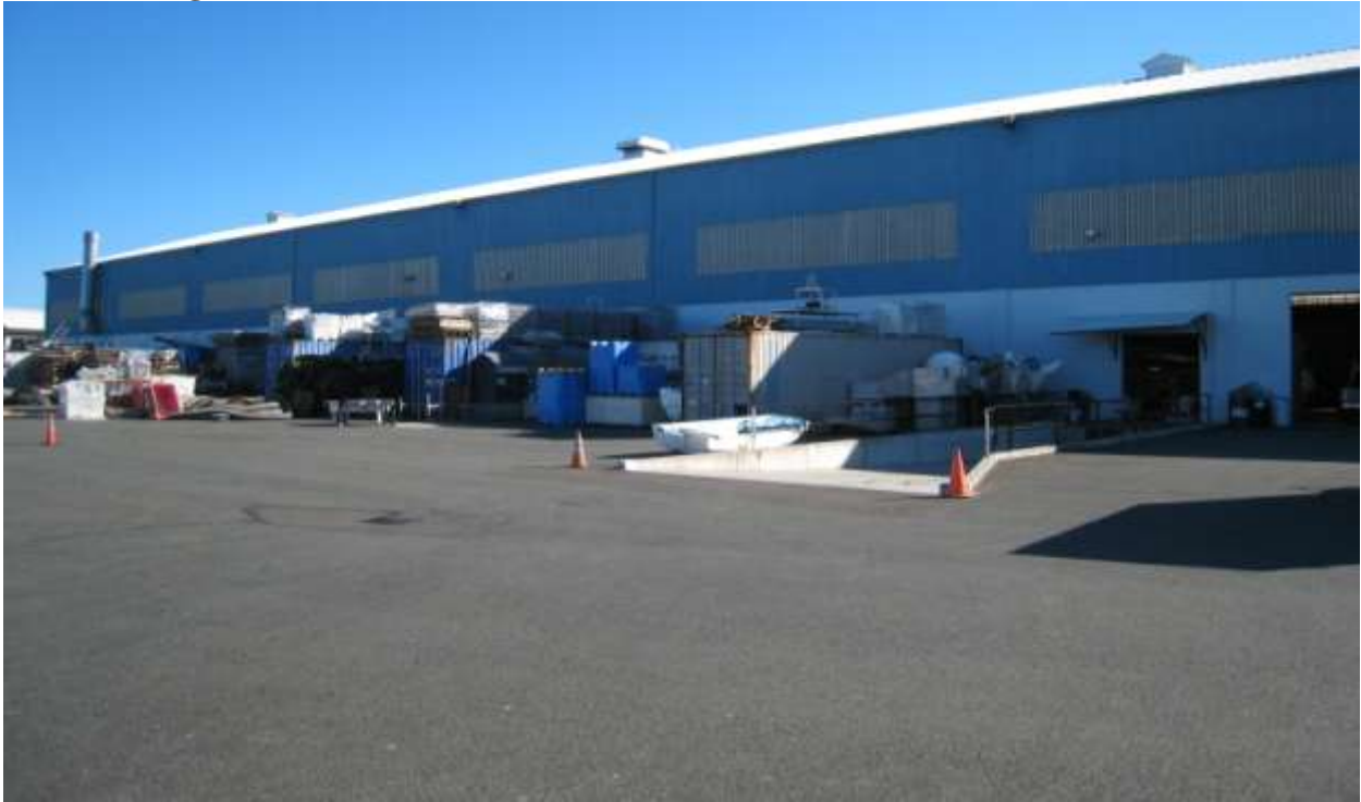
Photo 1: Ferguson Terminal Warehouse - from the south
