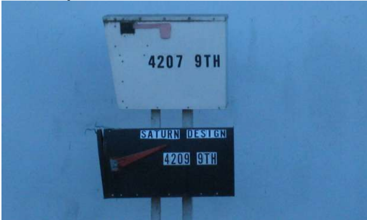
Photo 4: Close-up of the address of record at the northwest end of the warehouse
