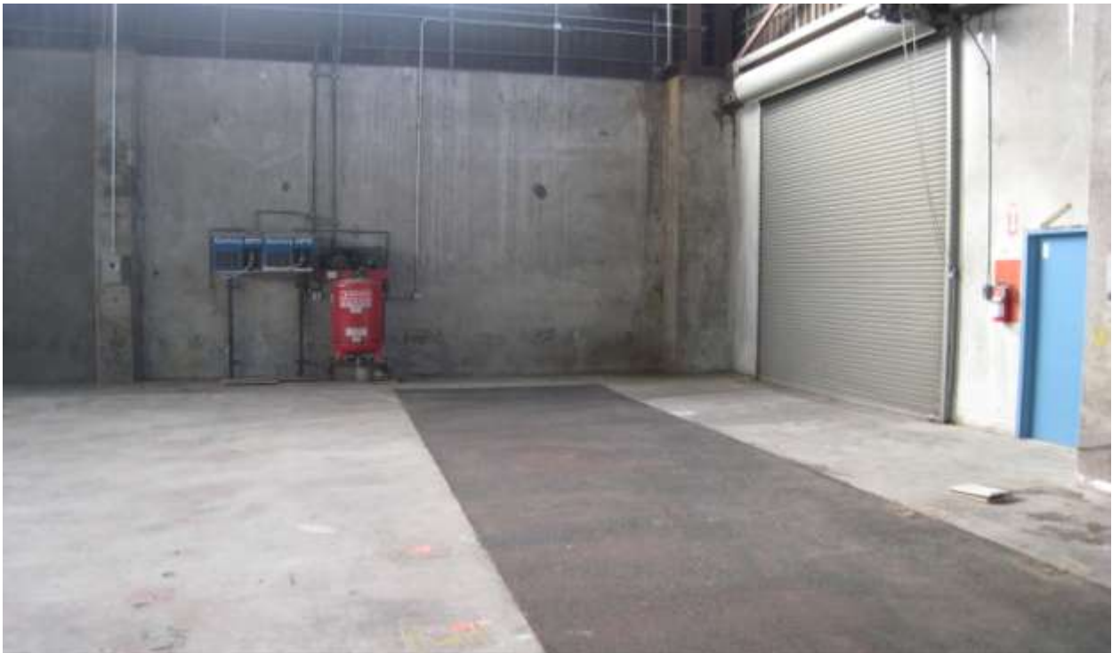
Photo 2: Interior of the warehouse – southeast end
