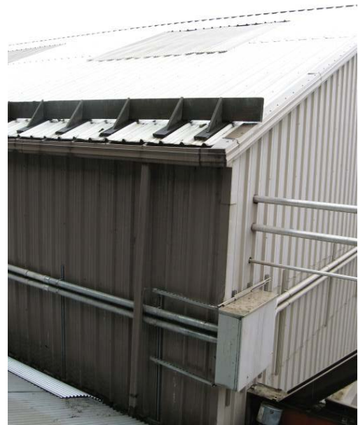
Photo 2 Forge Shop West Roof Surface
