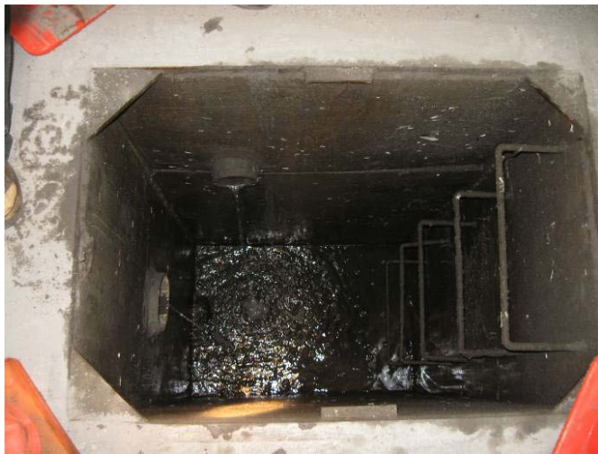
Photo 7 Outfall 002 Upgradient Vault Interior
