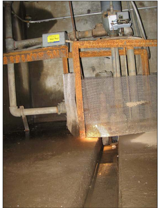
Photo 2 Railroad Scale Vault
