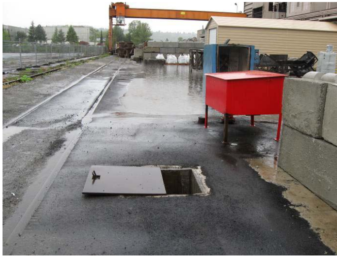
Photo 5 Outfall 001 Upgradient Vault Exterior
