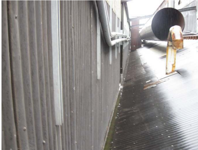
Photo 1 Forge Shop East Roof Surface
