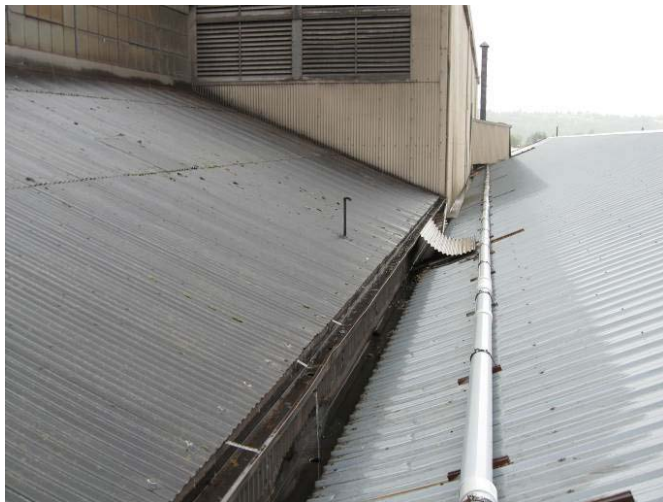
Photo 3 Machine Shop and Heat Treat Area Roof West
