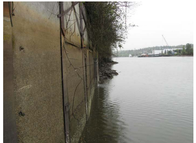
Photo 4 Outfall 001 Along Concrete Panel Wall
