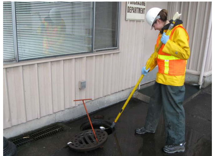
Photo 12 South of Shipping Area
