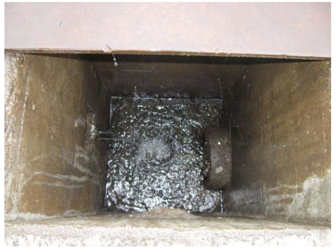
Photo 6 Outfall 001 Upgradient Vault Interior
