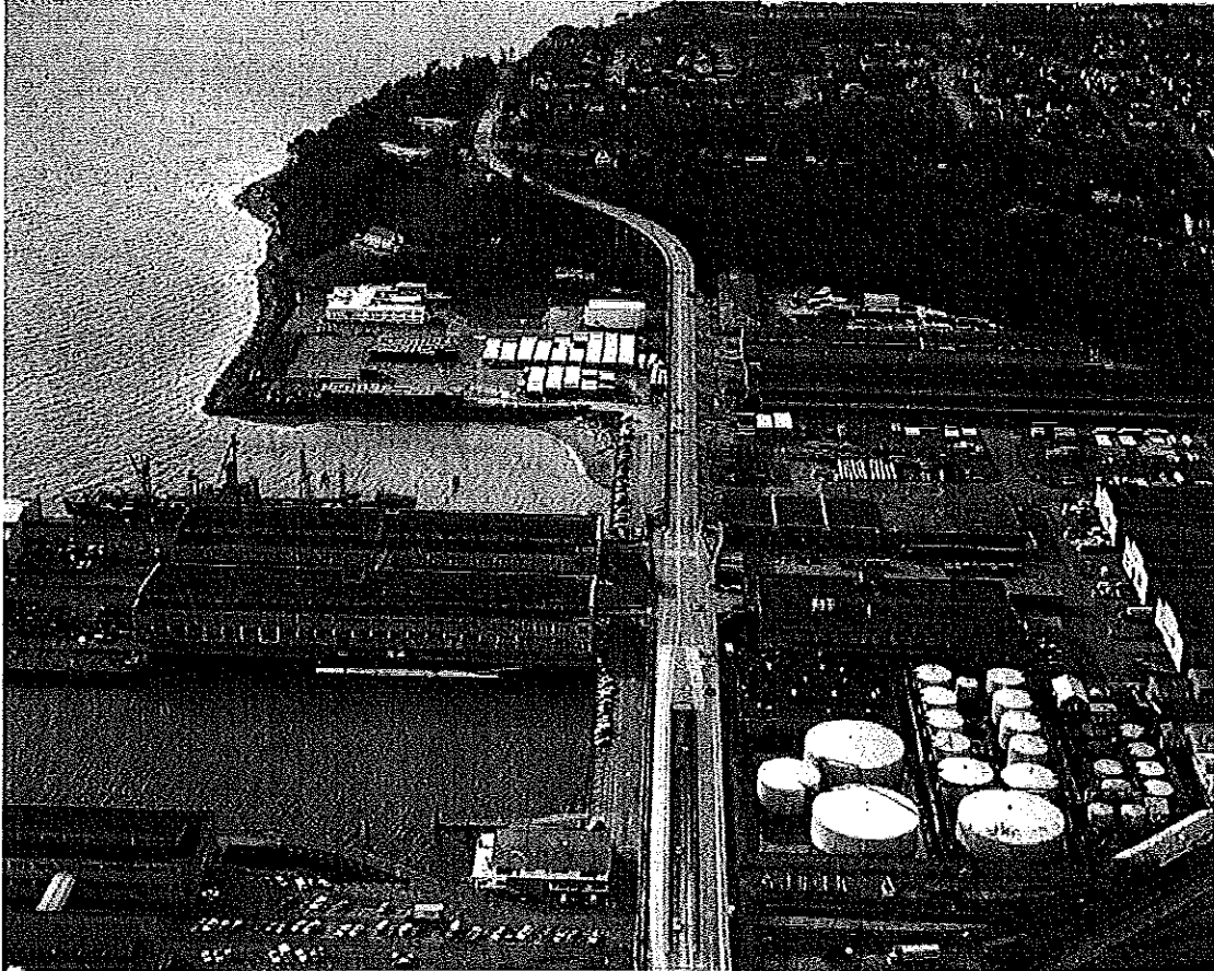
Historical photo from 1975, prior to Tank Farm Demolition
