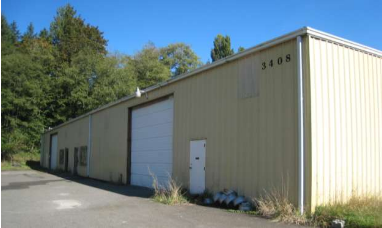
Photo 1: Warehouse building – UST area at left
