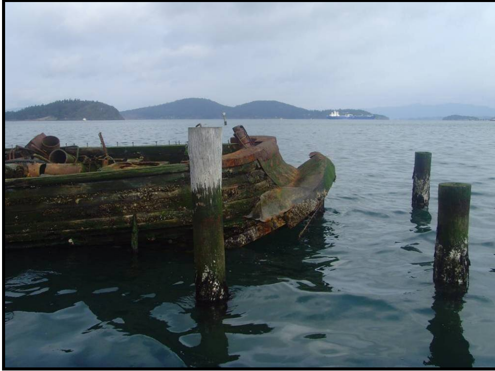
Figure 6. Stern of Enchantress caught on piling (view west).
