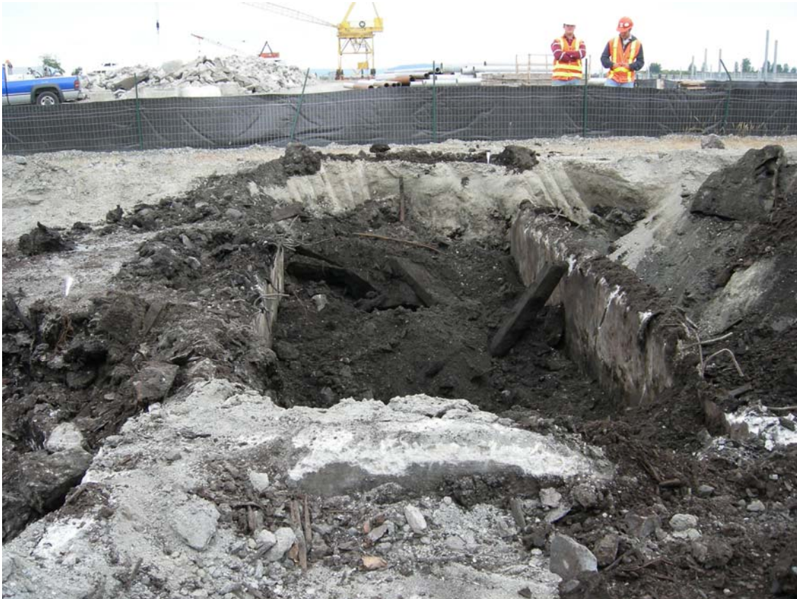
Concrete vault in Area J-1, looking west
