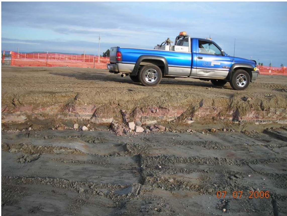
Colored concrete-like material layer visible in I-3a, looking west.
