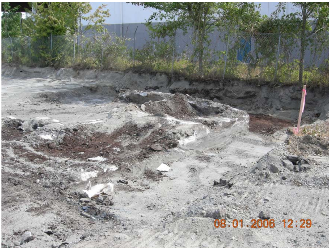
South end of J-1 excavation with edge of vault exposed.
