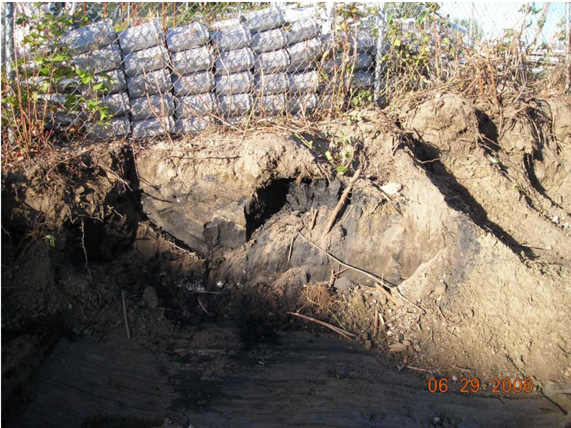
Black sand material on south sidewall of G-1, looking south.
