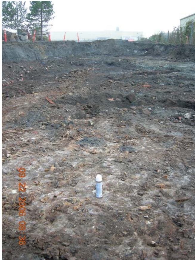
J-3, looking north along excavation bottom.
