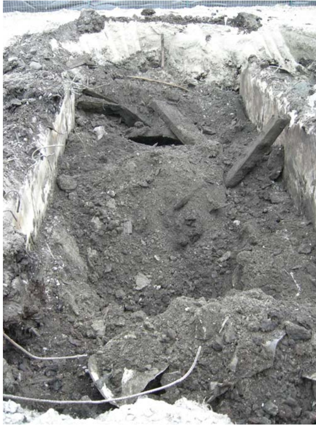
J-1 concrete vault, looking west.
