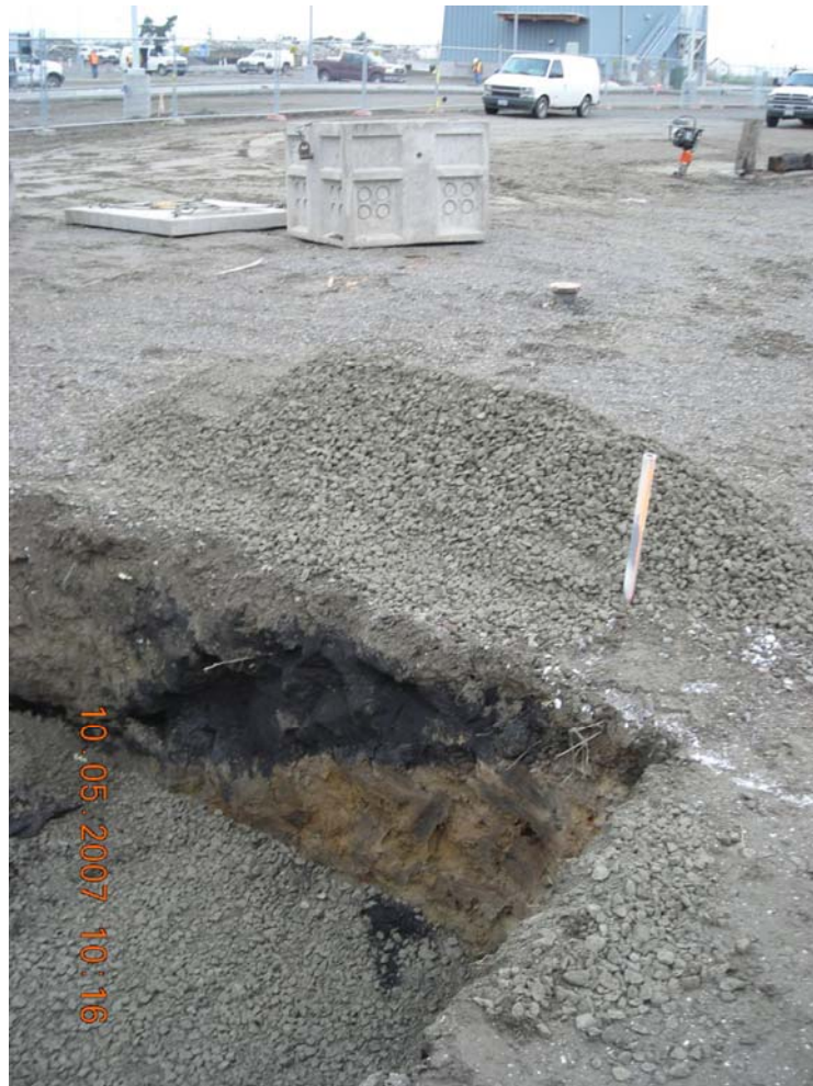
G-1a, looking west-southwest before start of excavation. Note black sand material.
