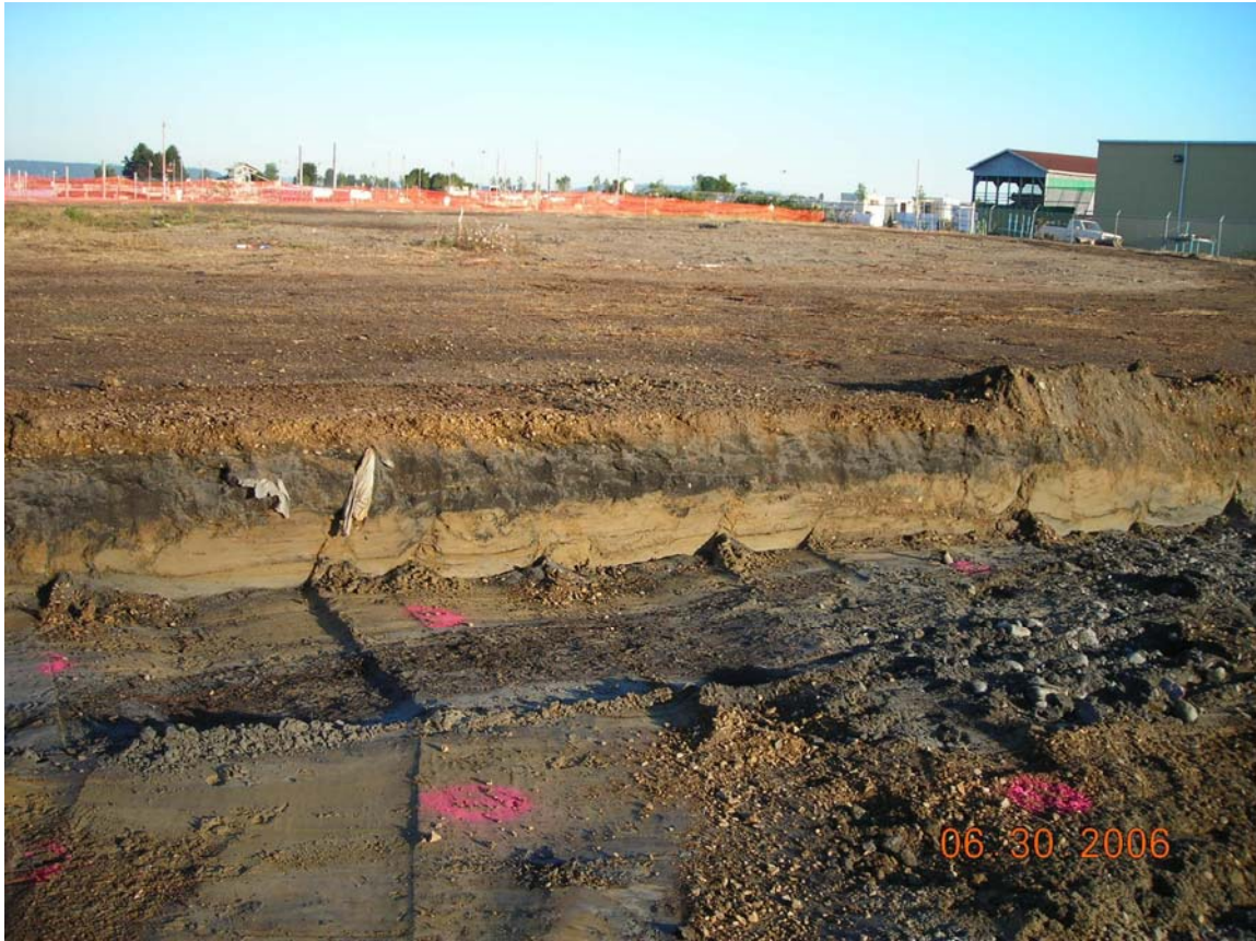
Excavating I-3a, notice thick black sand material layer looking west northwest.
