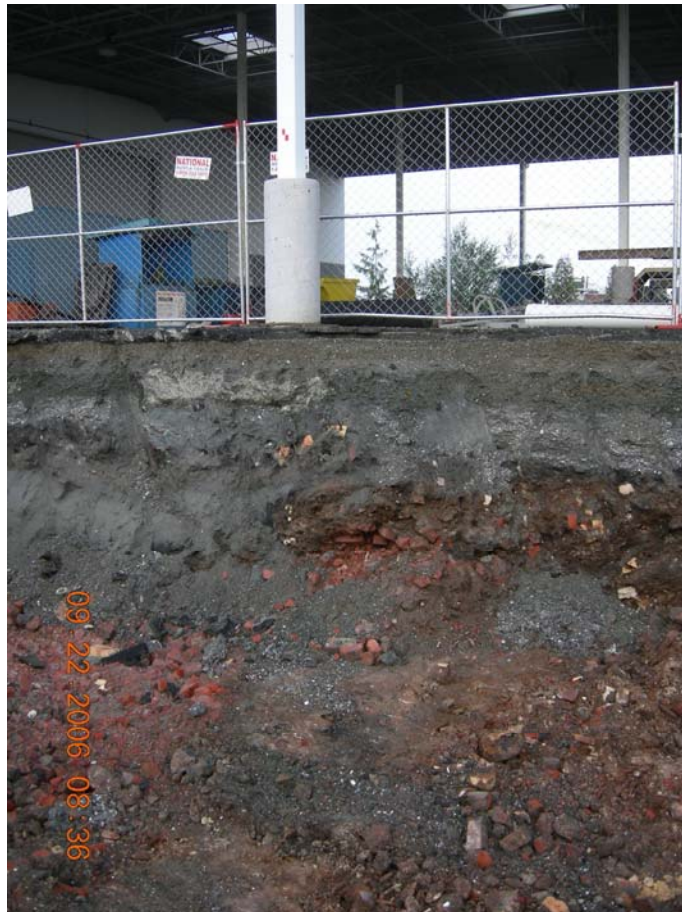
J-3, Construction debris looking west-northwest.
