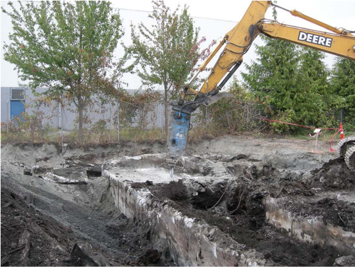
J-1, ICI jacking open chamber 1, looking east.
