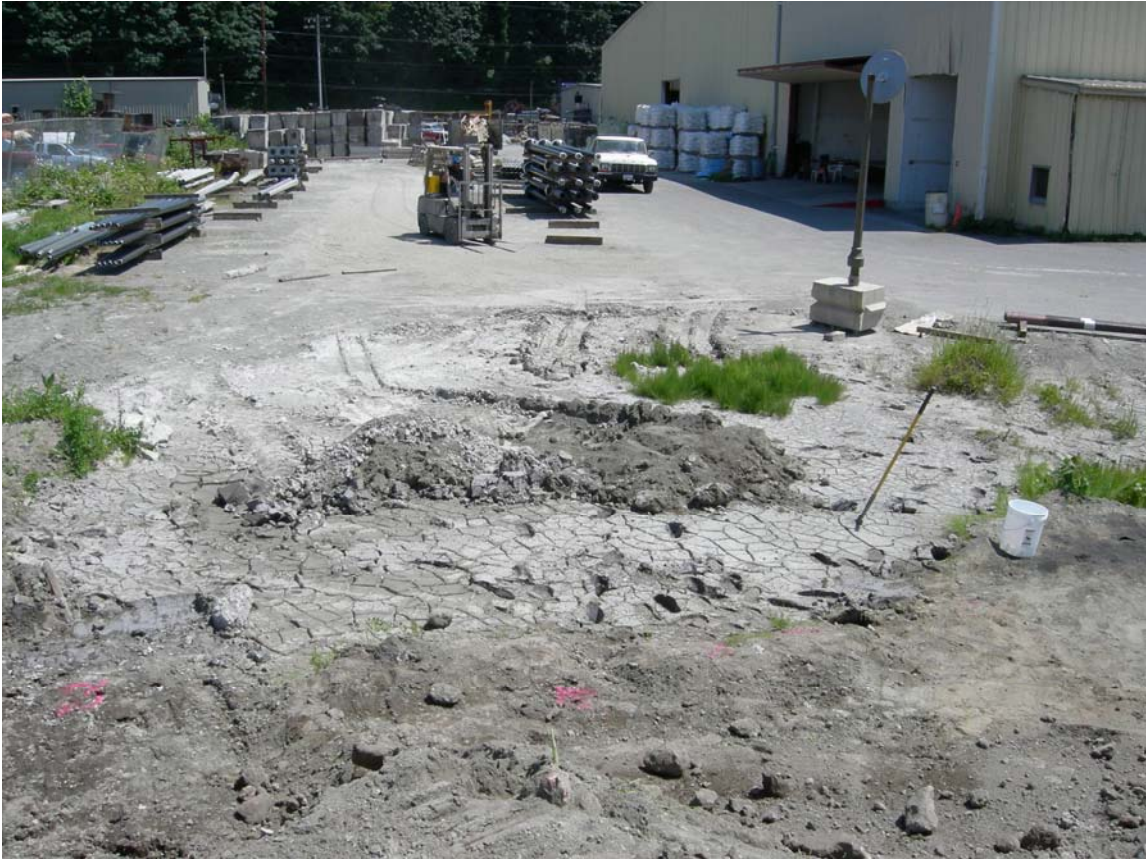
G-1 looking east at freshly placed material overlying area with desiccation cracks.
