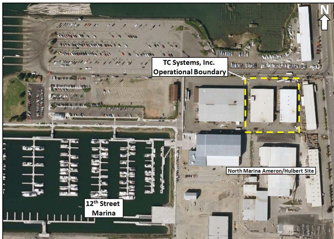
Figure 2: A current view of the TC Systems, Inc. Site. (Photo Source: 2010 Google Imagery)
