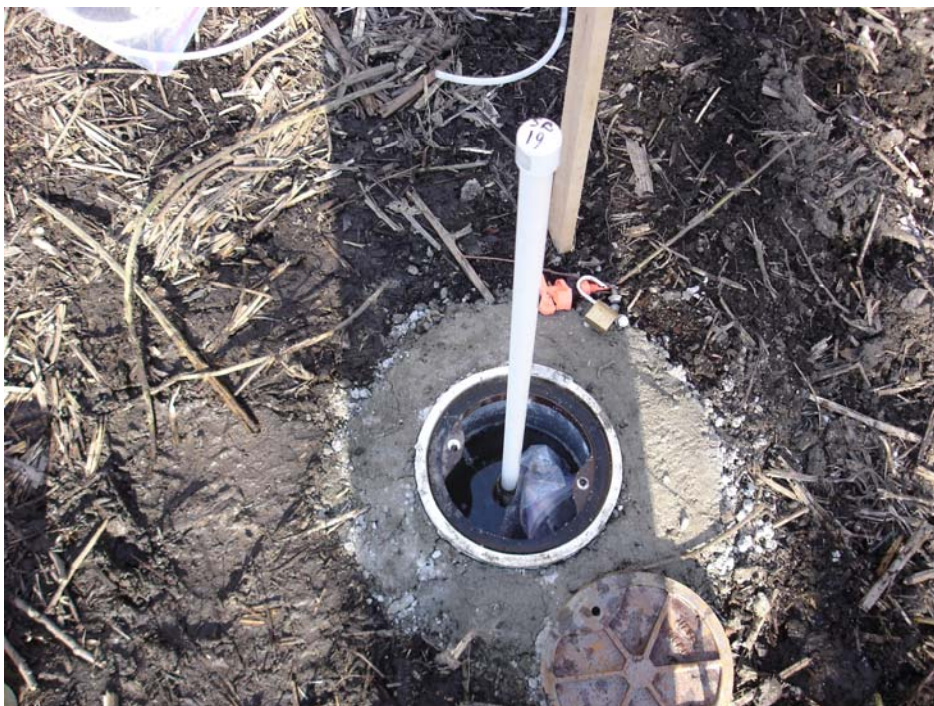
Photo 10. PVC surge block used to develop piezometers that produced little water.
