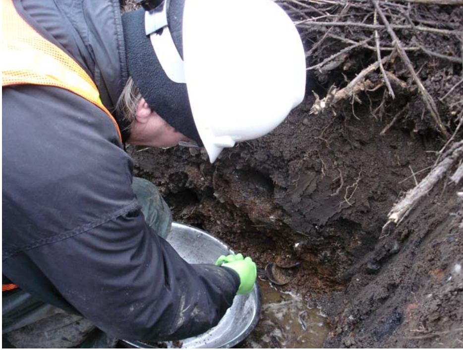
Photo 13. Soil sample collection from 1.7 to 2.2 ft below ground surface at test pit TP-22.
