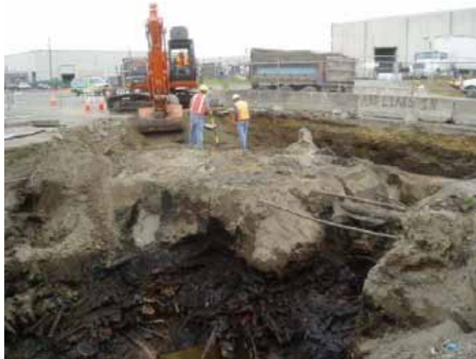
Photo 2 Site conditions, note thickness of soil fill overlying wood fill
