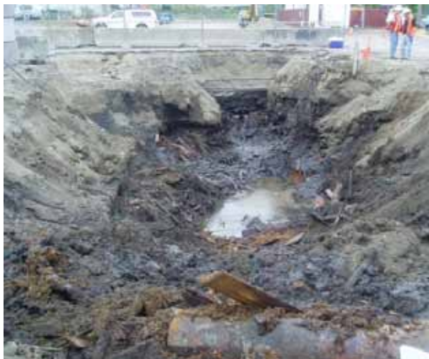
Photo 1 Site conditions, note size of wood debris in wood fill, large log in foreground
