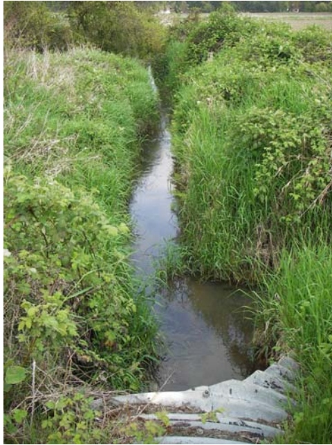
Photo 15: Culvert facing eastward
