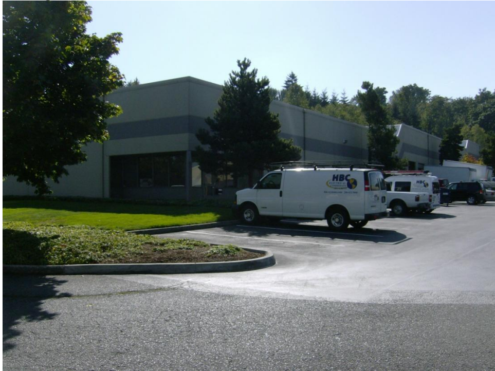
Photo 1: Building A – eastern end over contaminated soil
