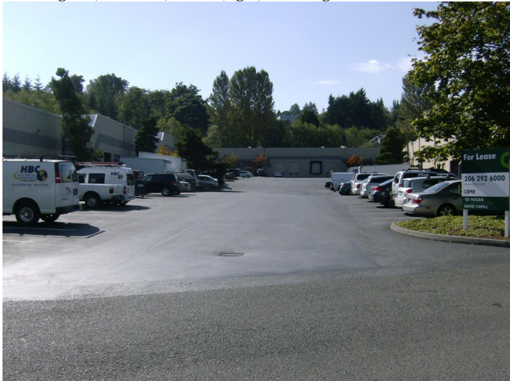
Photo 4: Buildings A (on the left) and C (right) – looking west
