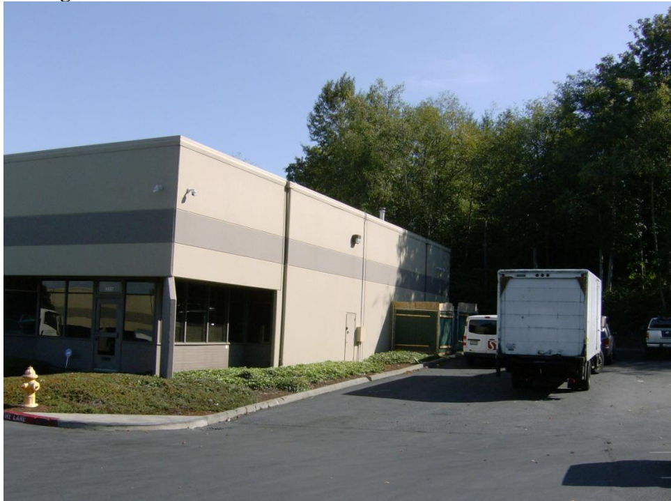
Photo 2: Building C – eastern end over contaminated soil
