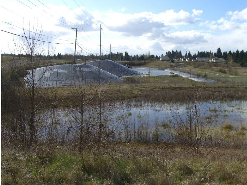
Photo 3: Stormwater Collection Area - from the east
