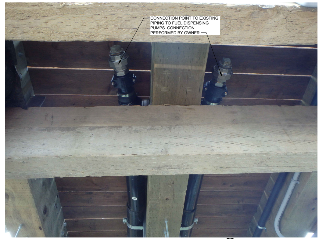
FUEL LINE CONNECTION AT DOCK DETAIL 4
