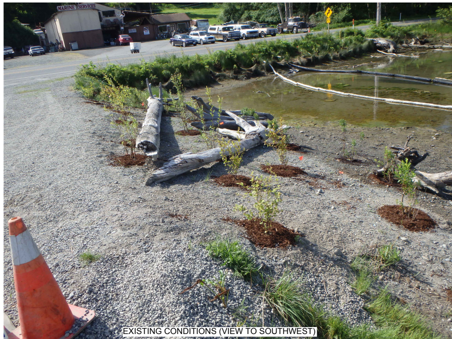
EXISTING CONDITIONS (VIEW TO SOUTHWEST)
