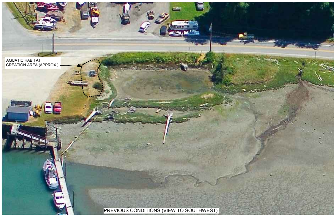
PREVIOUS CONDITIONS (VIEW TO SOUTHWEST)
