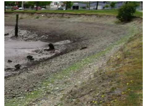
Gravel from the post-1975 fill forms the shoreline adjacent to Budd Inlet.
