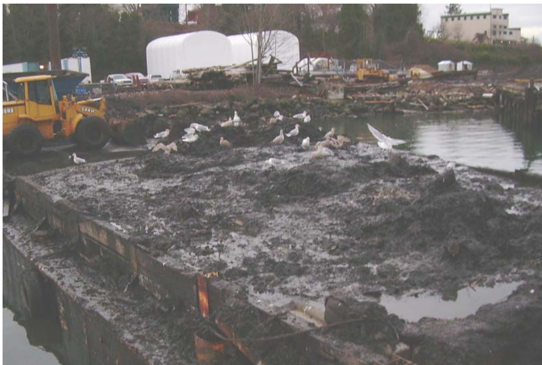
Photograph 7 - Wet silty, heterogeneous sediment/woodwaste dewatering/decanting on barge.
