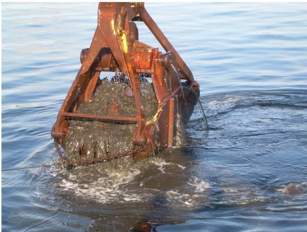
Photograph 3 - Dredge bucket full of sediment at water surface.
