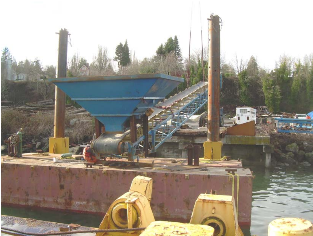
Photograph 15 - Dredge sediment offloading area hopper and conveyor setup.
