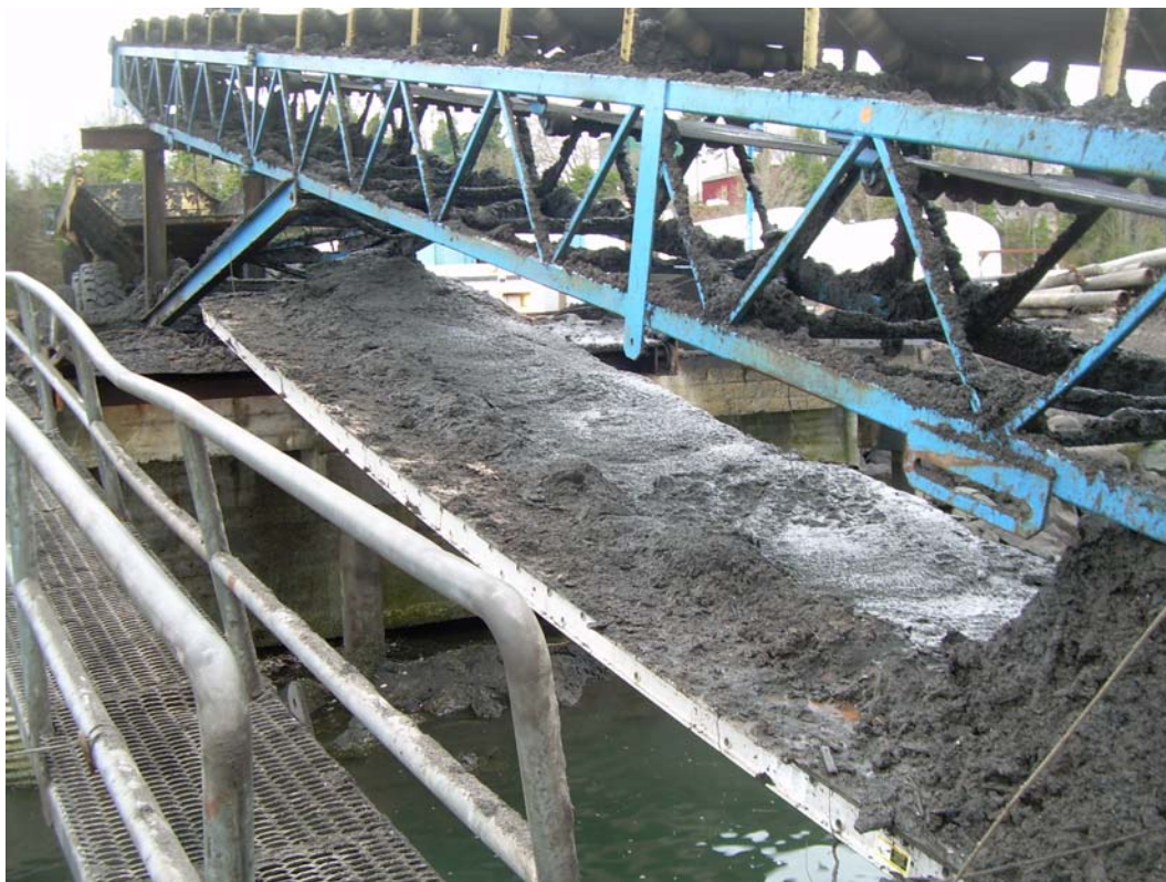
Photograph 20 - Close up of planking under offloading conveyor.
