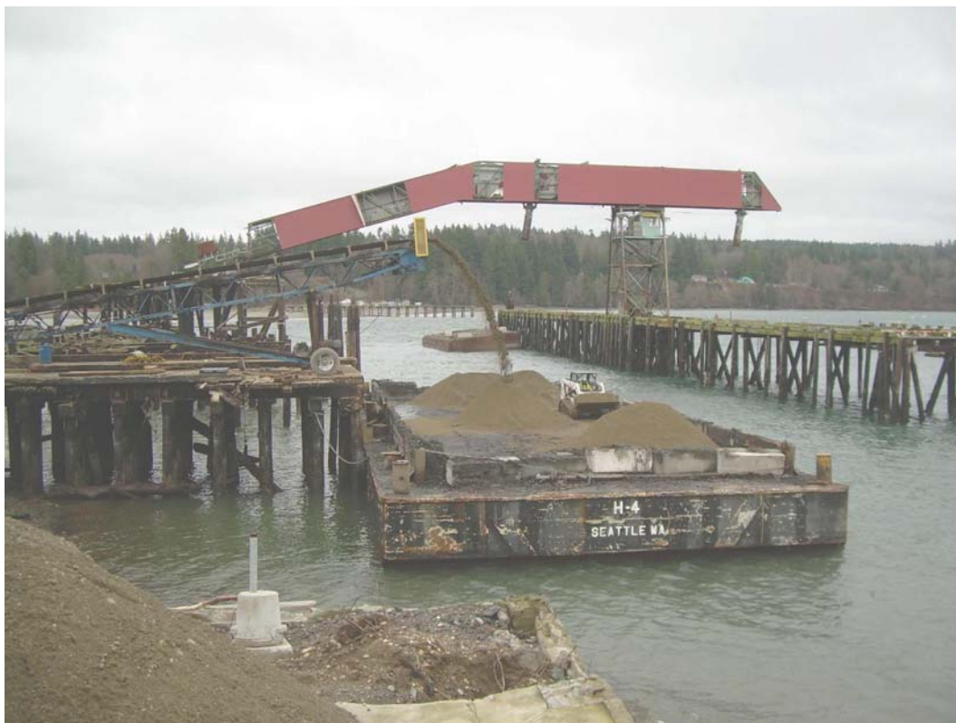
Photograph 18 - Loading of barge with cover sand material.
