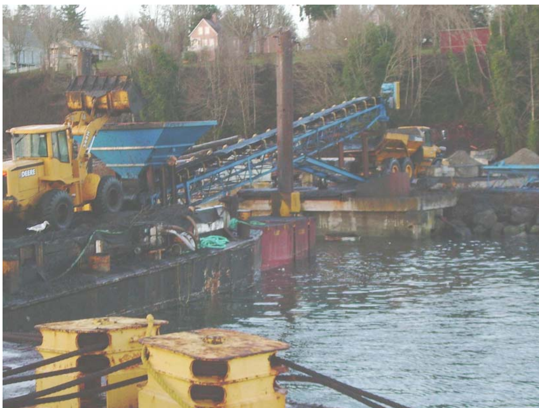
Photograph 14 - Loader and off-road truck offloading dredge sediment.
