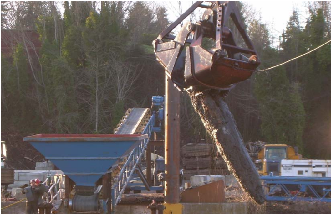
Photograph 9 - Large wood debris being loaded onto barge.
