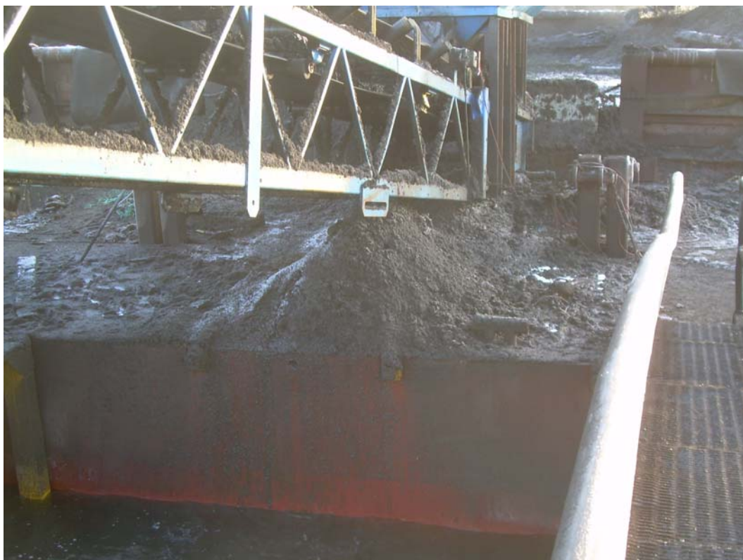
Photograph 19 - Spilling of wet sediment off of offloading conveyor prior to installation of planking to catch sediment.
