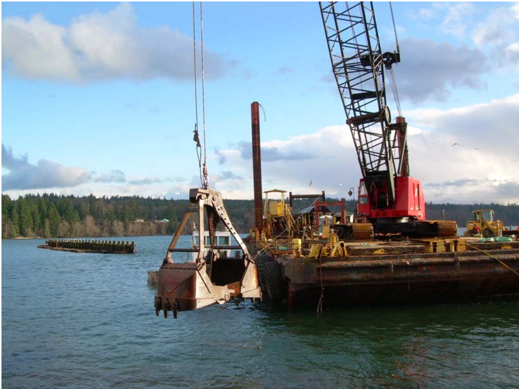
Photograph 1 - Dredging barge, crane, and bucket about to excavate sediment.
