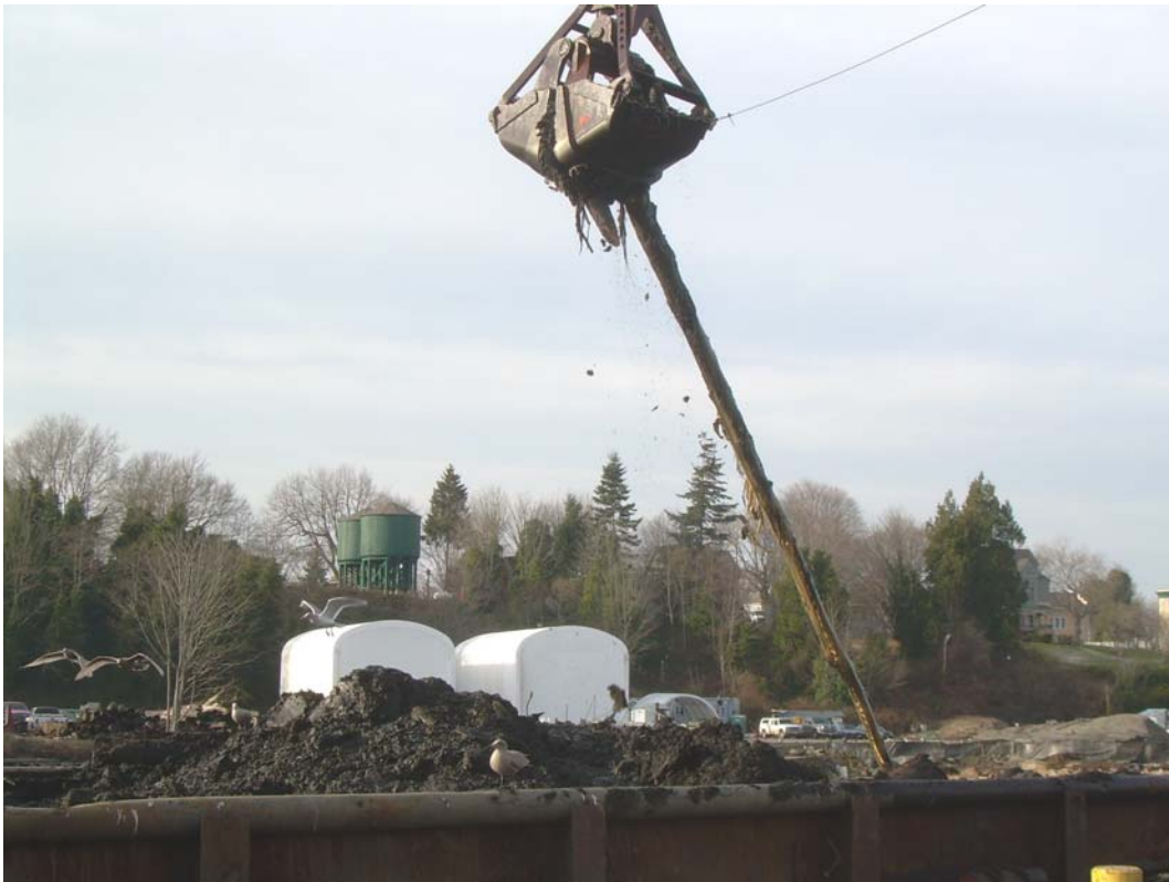
Photograph 10 - Timber pile being loaded on barge.
