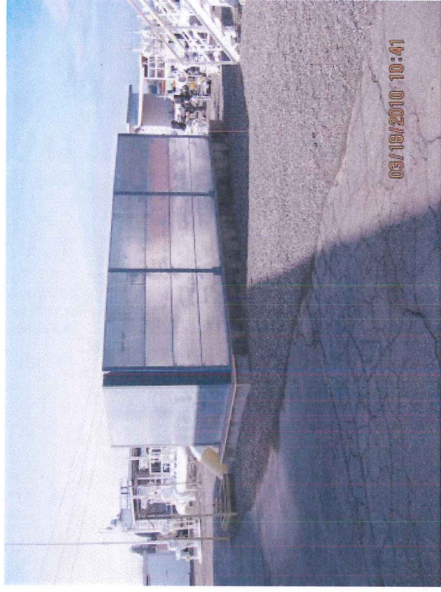
Sound barrier around pumps
