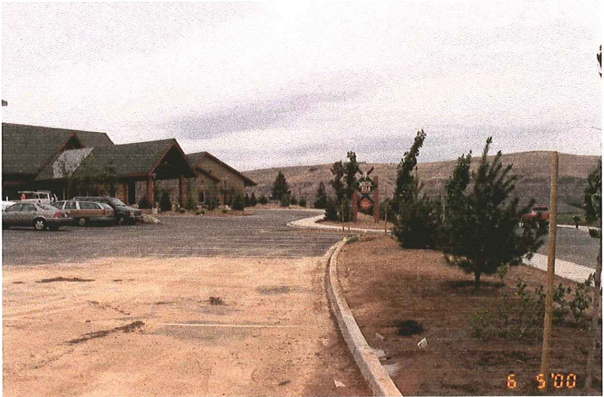
Picture 9: View from the south looking north. Initial site landscaping.
