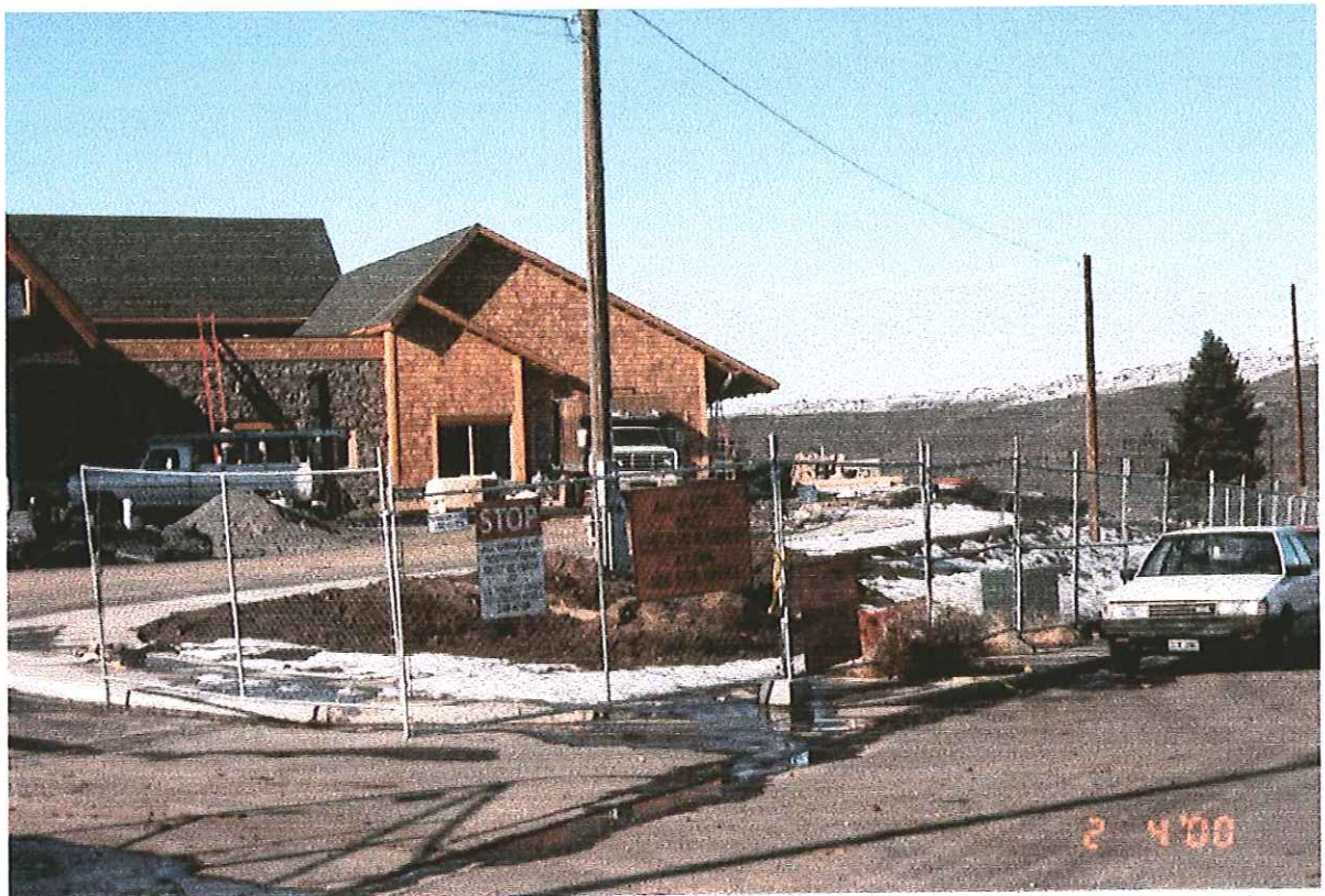
Picture 7: View from the east looking northwest. North Star Lodging nearing the end of the construction phase.
