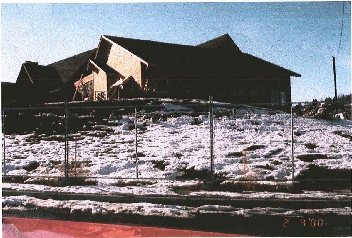
Picture 8: View from the northeast looking southwest. North Star Lodging nearing the end of the construction phase.
