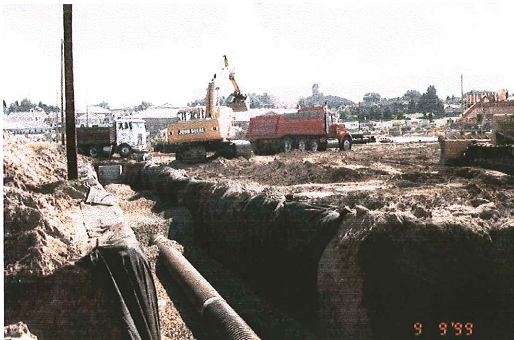
Picture 6: View to the southeast. Trench closure over water main installation.
