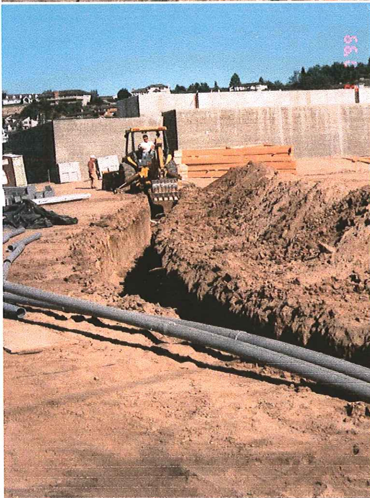
Pictures 3&4: View from the west looking east. Water main installation.
