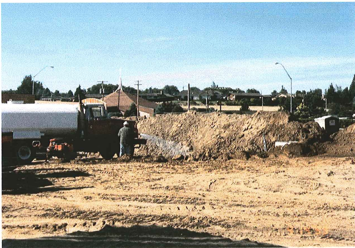
Picture 2: View from the east looking west. Dust suppression activities.
