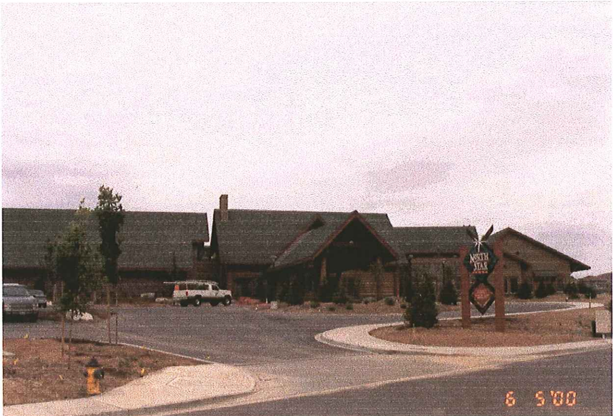
Picture 10: View from the west looking east. Initial site landscaping.
