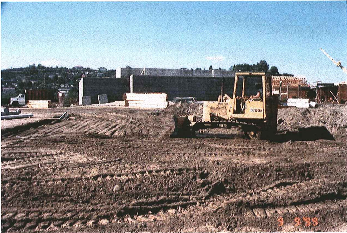
Picture 1: View from west looking east. Completion of vegetation removal.
