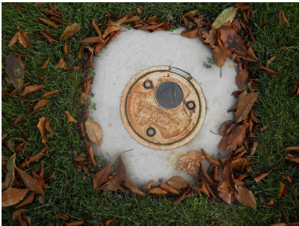
Photo 4: Photo of access port to monitoring well 6, typical of all MW on site.
