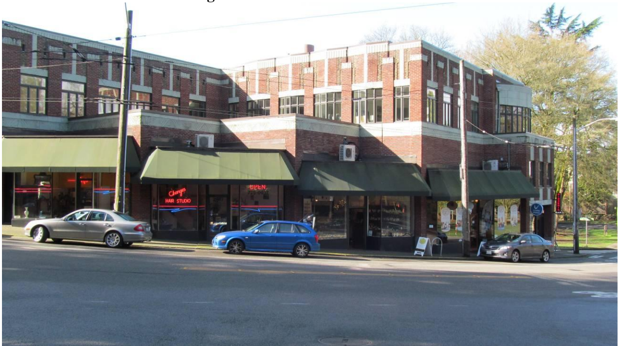
Photo 4: North Side of Building – from the north
