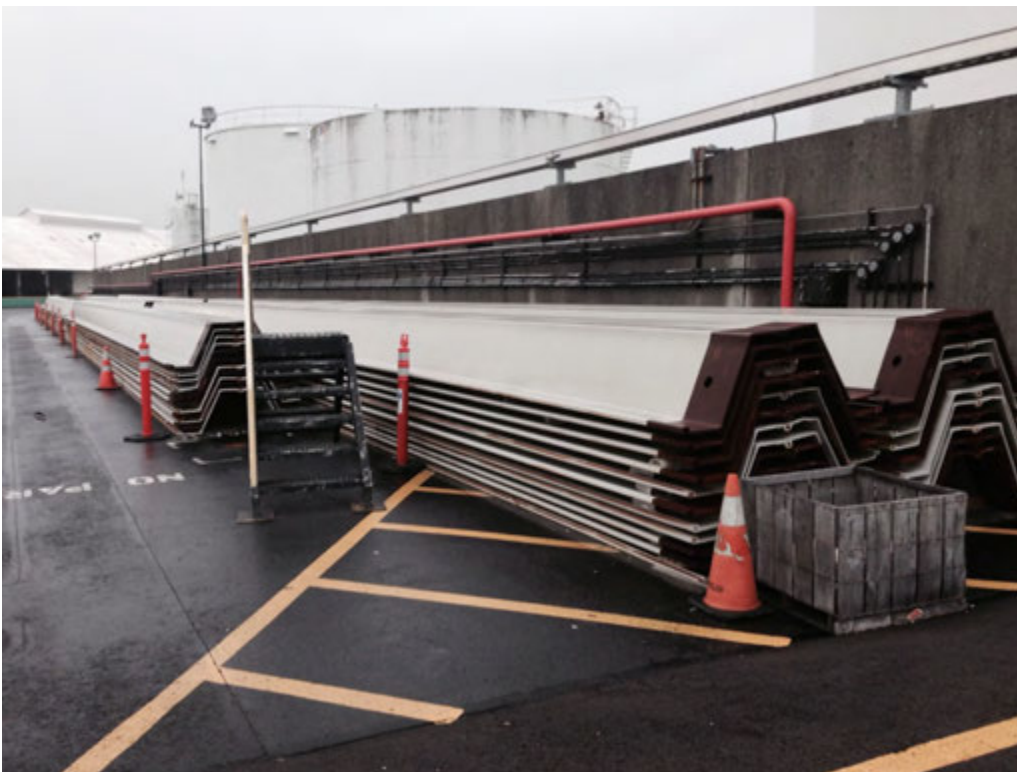
Photo 10. BP Terminal outside south wall for Plant 1 where new materials for new seawall are temporarily stored and waiting permit approval to replace West Waterway seawall and AST No. 9 and 13 in background.
