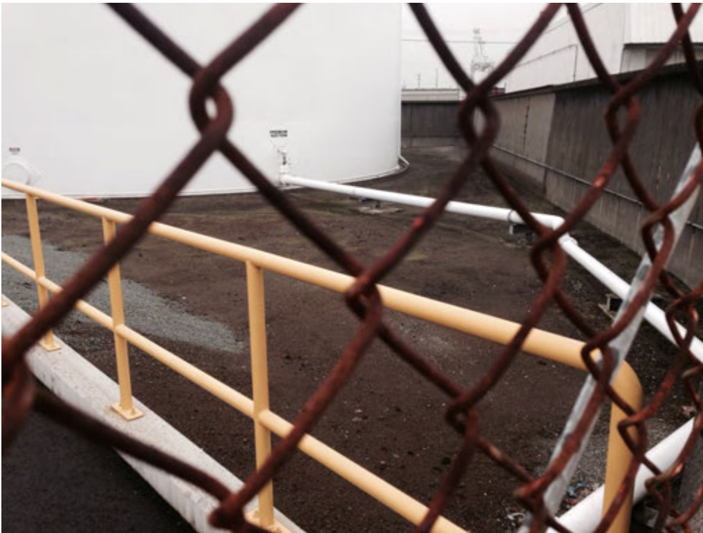
Photo 9. BP Terminal Plant 1 at south wall looking east where above ground storage tank (AST) No. 8 with monitoring well GM-16S is located in distance at the southeast corner of Plant 1.
