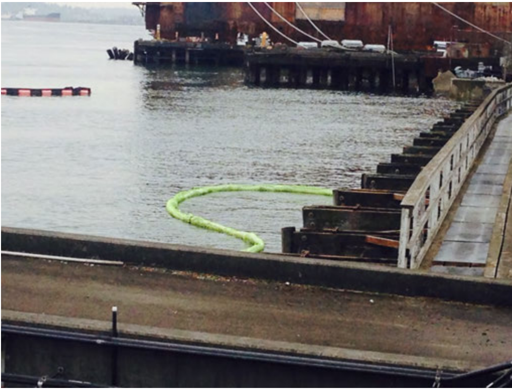
Photo 3. BP Terminal seawall and green boom to capture any sheen or floating product on West Waterway as a safety measure, and photo looking NNW at West Waterway and Elliott Bay in the background.
