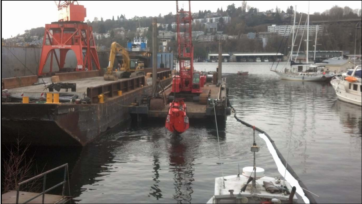
Photograph 7 – Dredging operations begin (December 5, 2013).
