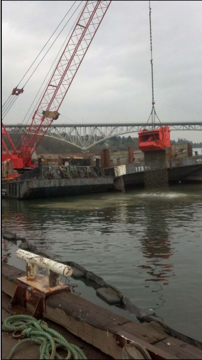
Photograph 30 – Final day of thin-layer placement (March 25, 2014).
