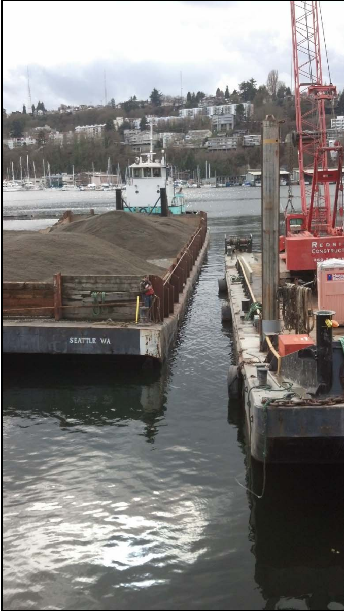
Photograph 28 – Contractor receiving a barge full of thin-layer capping material (March 10, 2014).
