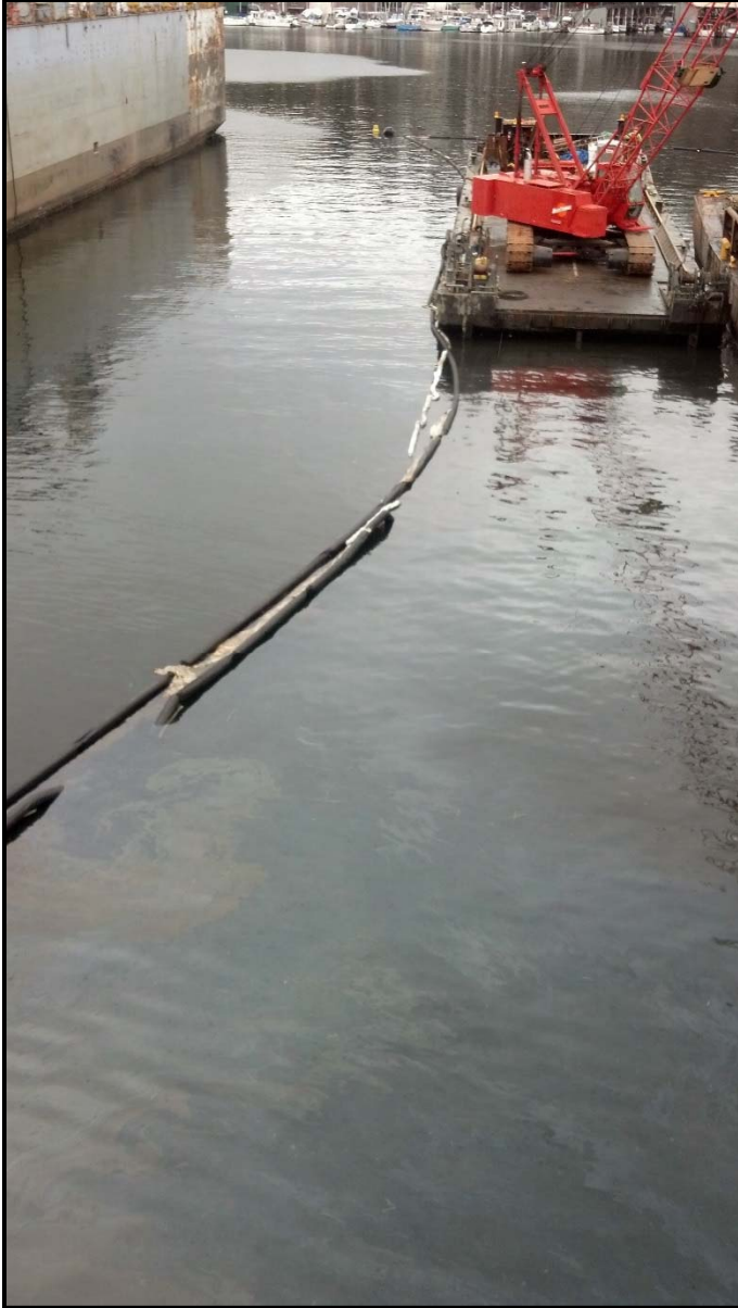
Photograph 23 – Water quality controls during Phase II dredging operations (January 31, 2014).
