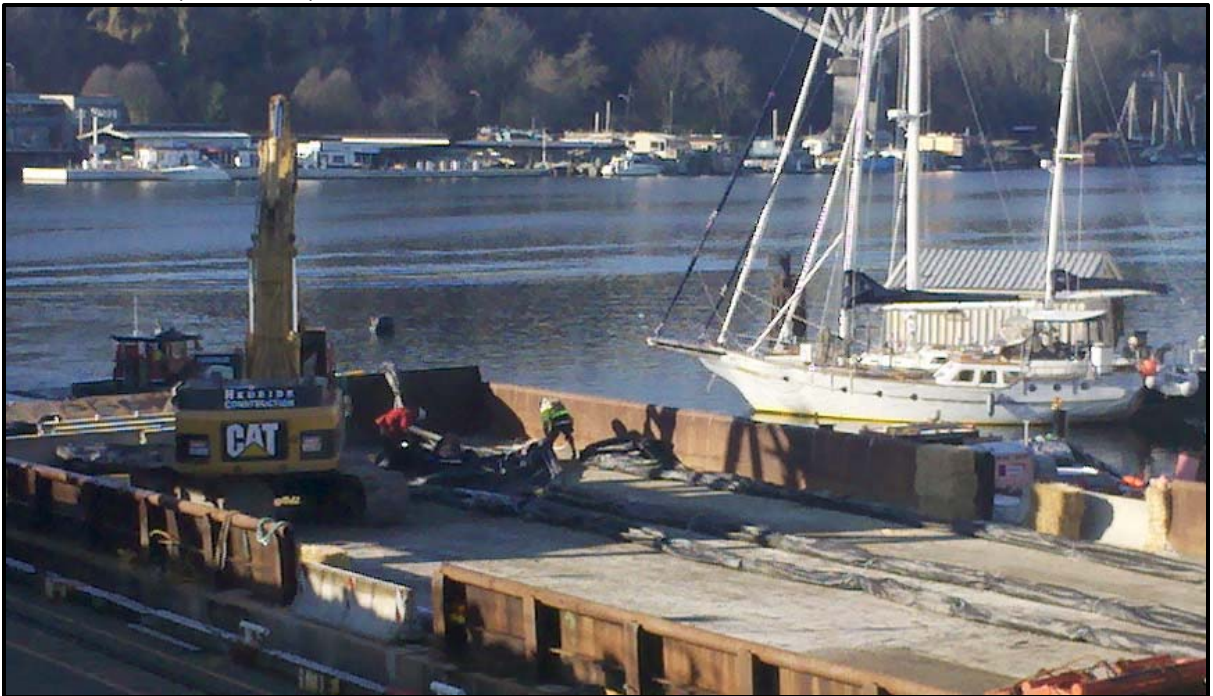
Photograph 2 – Preparing deployment water quality controls at the beginning of construction (Dec 4, 2013).
