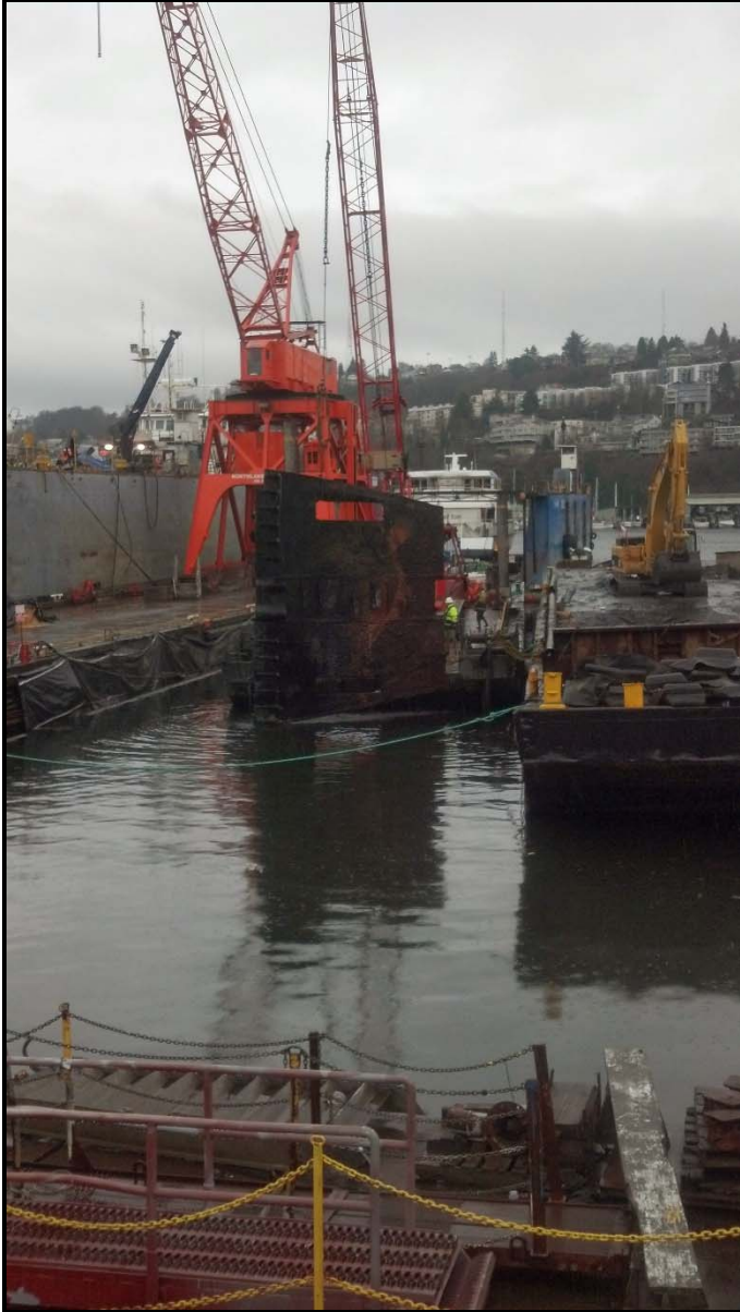
Photograph 14 – Large piece of steel recovered during dredging operations (December 27, 2013).
