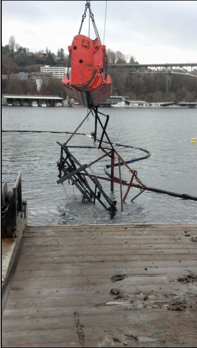
Photograph 15 – Example of scrap steel recovered during dredging operations (January 13, 2014).
