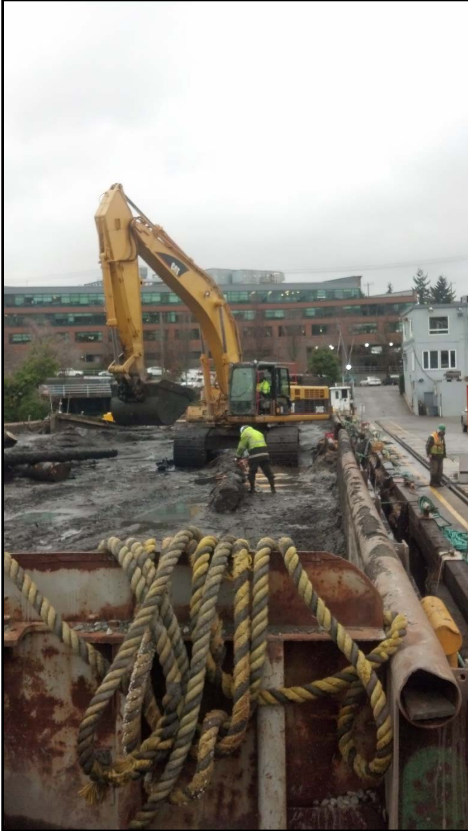
Photograph 19 – Contractor processing recovered timber piles for off-site disposal (January 10, 2014).
