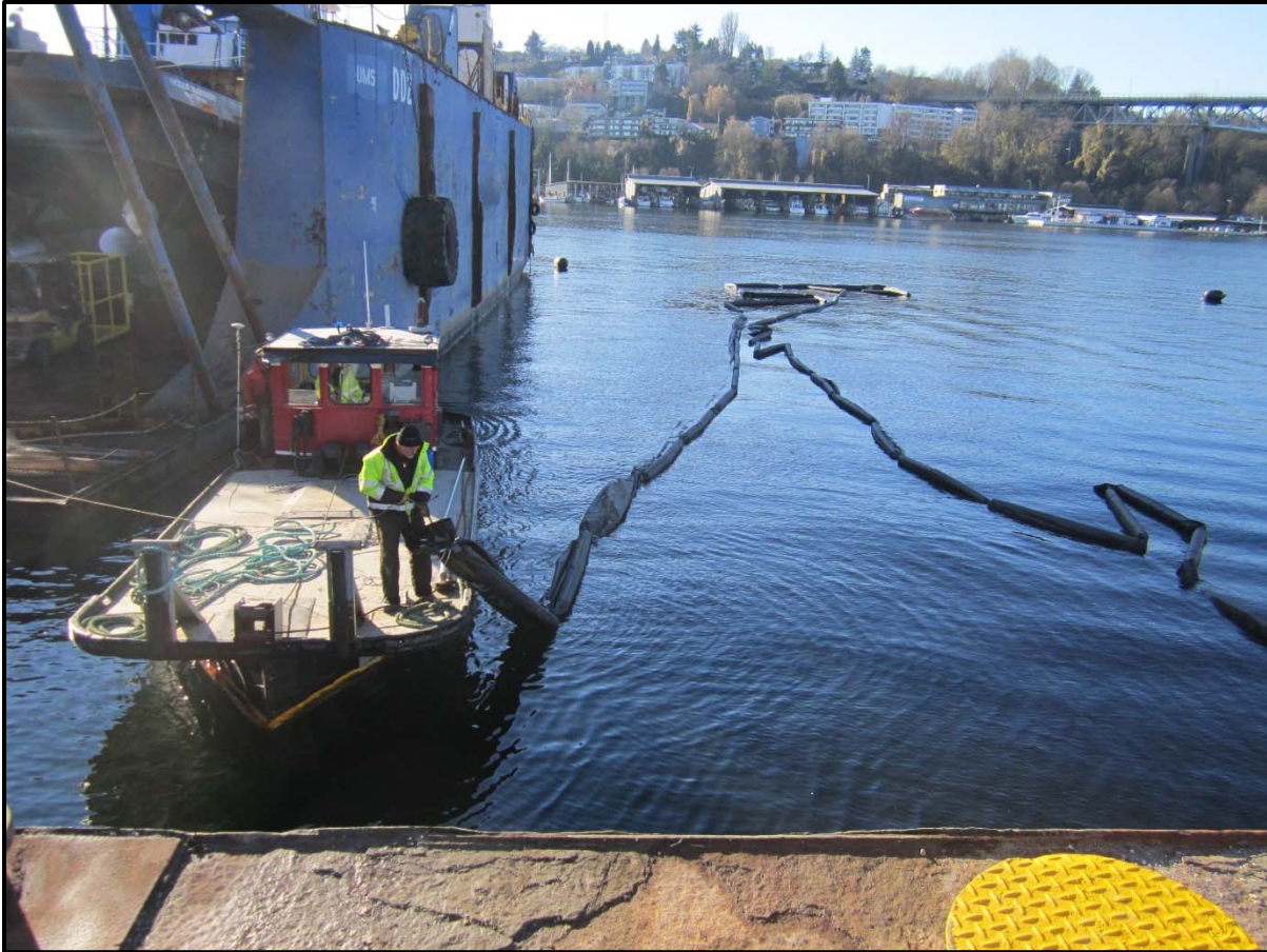
Photograph 3 – Deploying water quality controls at the beginning of construction (Dec 4, 2013).
