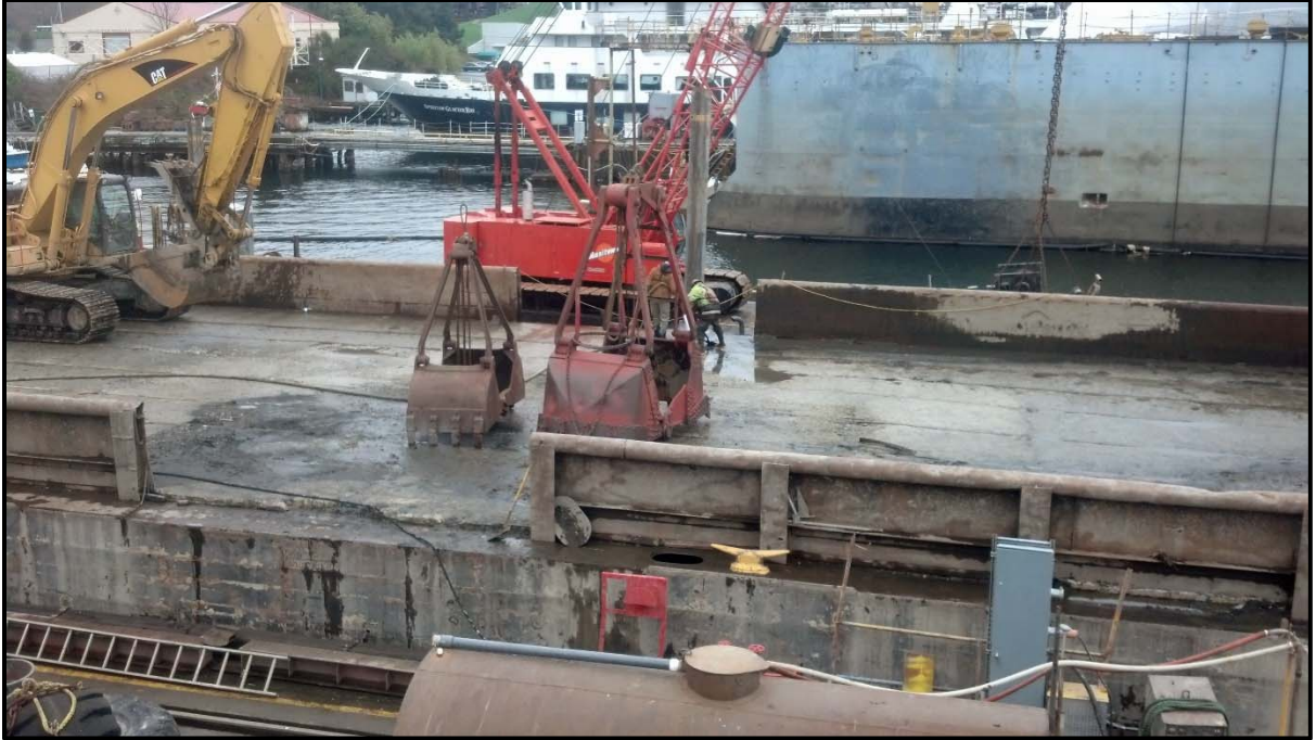
Photograph 27 – Cleaning the barge in preparation for thin-layer cap placement (March 6, 2014).
