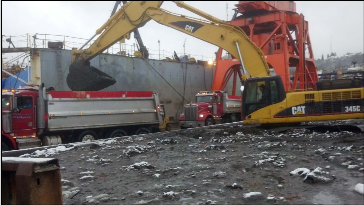
Photograph 20 – Transloading material for off-site disposal (December 20, 2014).
