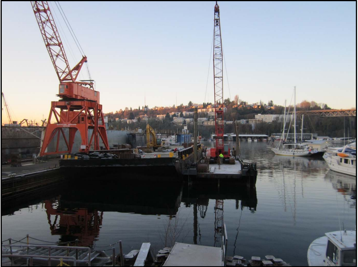
Photograph 1 – Pre-construction conditions and contractor mobilization at the Northlake Shipyard Site (Dec 4, 2013).
