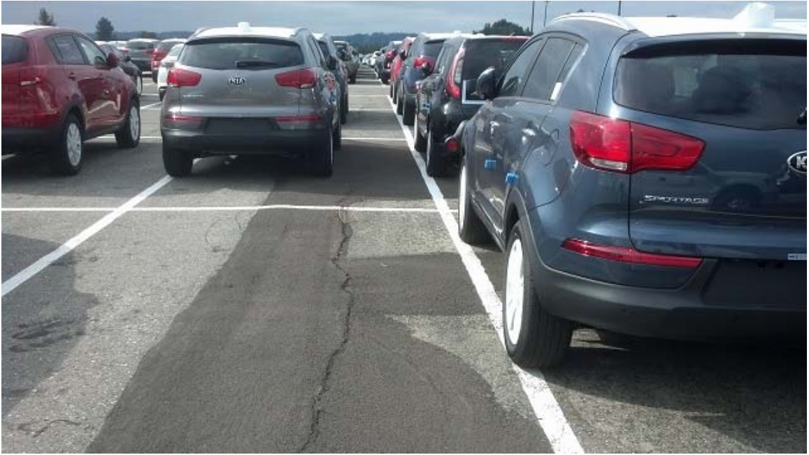
Photograph 1 – Observed cracks in cap.
