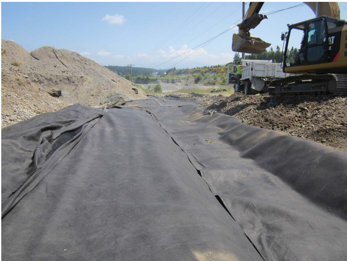
2014, June 2. Placement of geotextile filter over drain rock.
