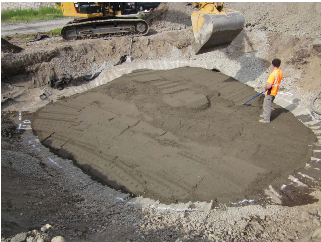
2014, May 15. Backfill placement at east sinkhole.
