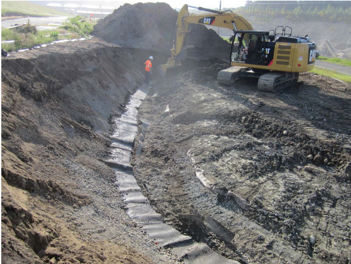
2014, May 14. Excavation at west sinkhole; viewing east.
