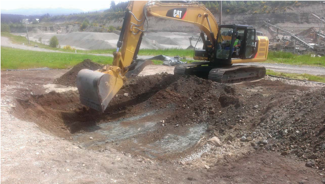
2014, May 12. Initial removal of cover soils, east sinkhole.
