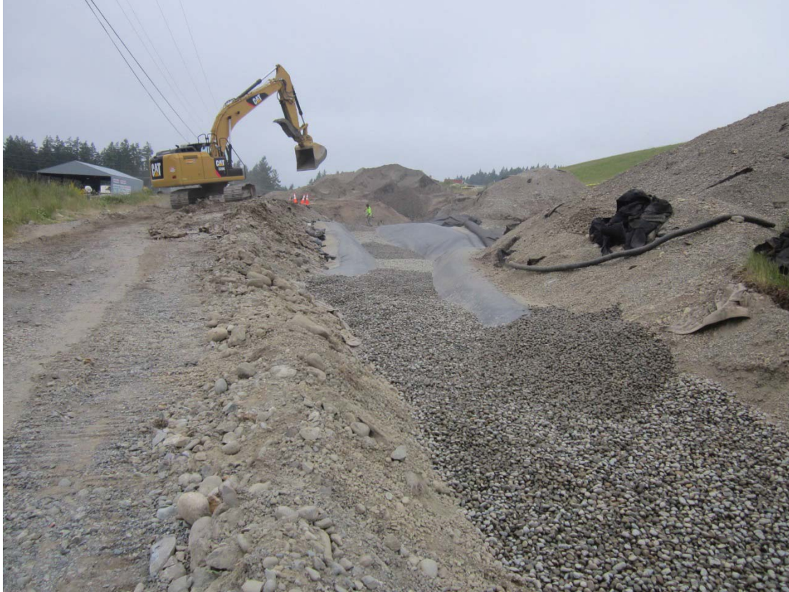
2014, June 2. Placement of drain rock within surface drainage feature.
