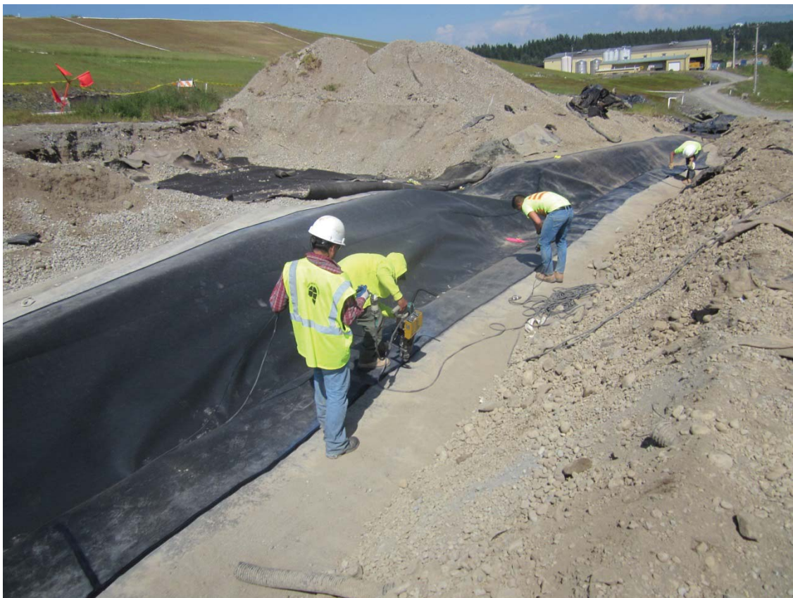
2014, May 30. Geomembrane installation.
