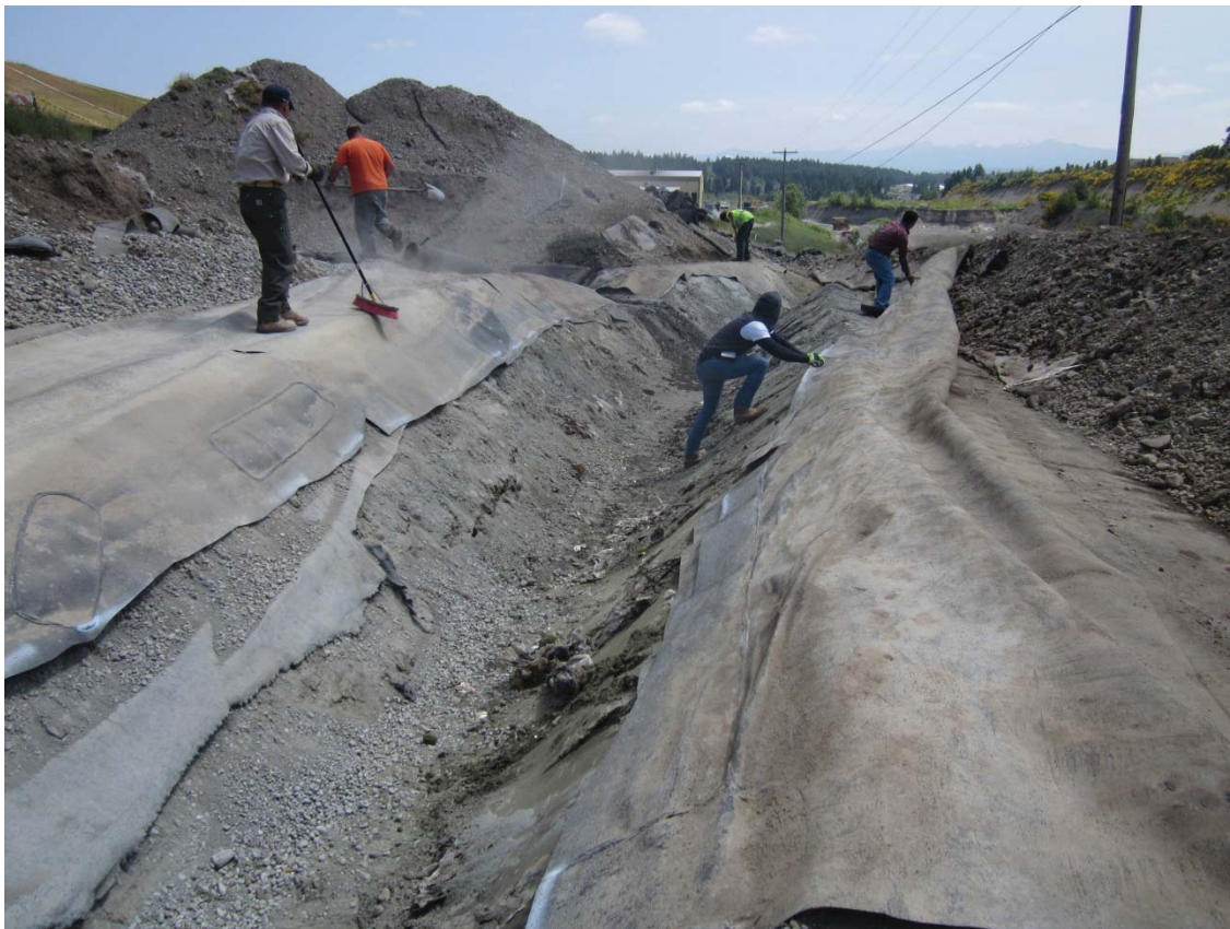
2014, May 30. Preparing subgrade for geomembrane placement.
