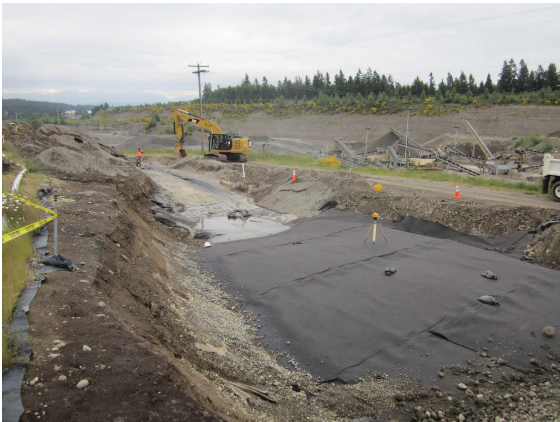
2014, May 29. Additional excavation to re-establish drainage.
