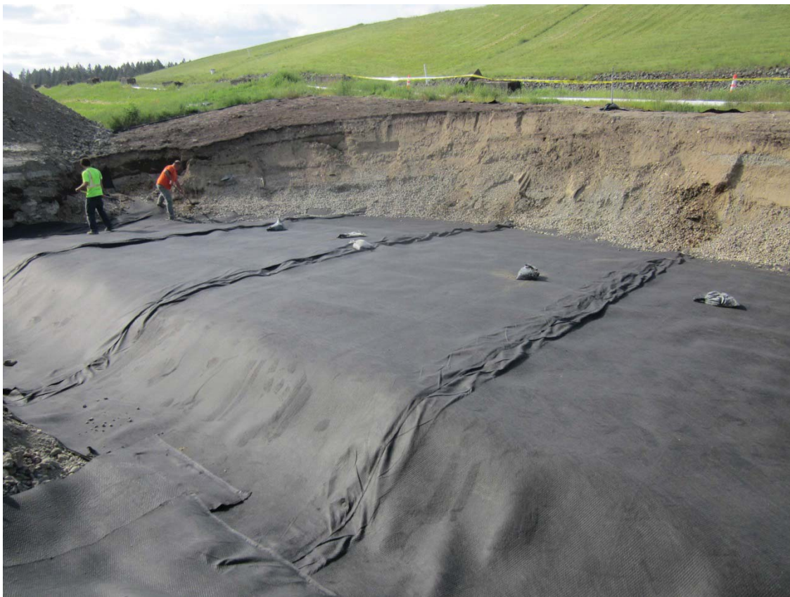
2014, May 16. Geonet composite installation; west sinkhole
