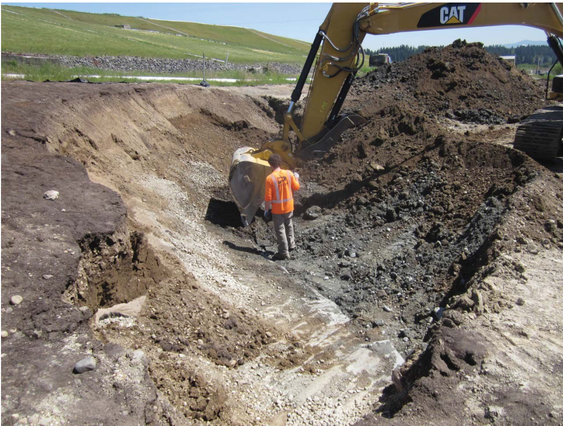
2014, May 13. Continuing removal of cover soils, east sinkhole.
