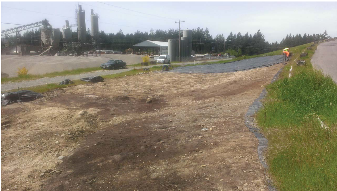
2014, May 12, viewing west. Removal of temporary plastic cover.
