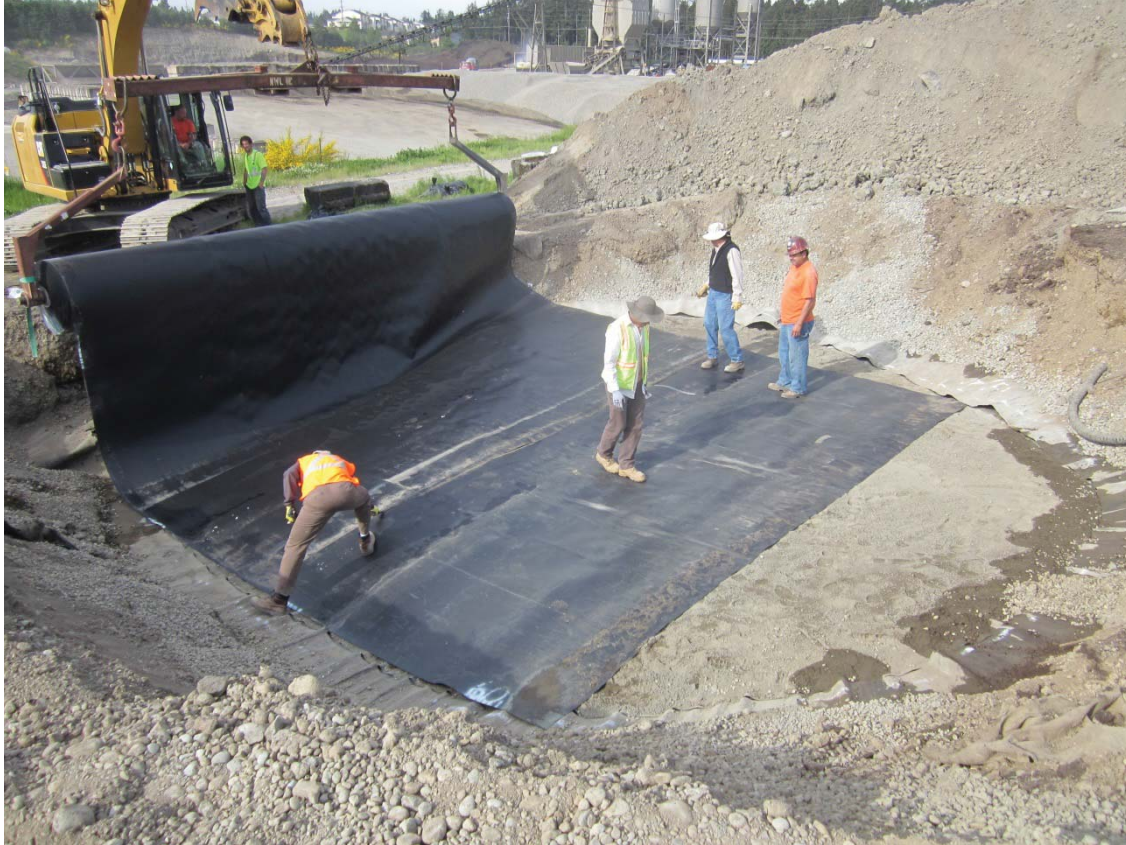
2014, May 16. Geomembrane placement; east sinkhole
