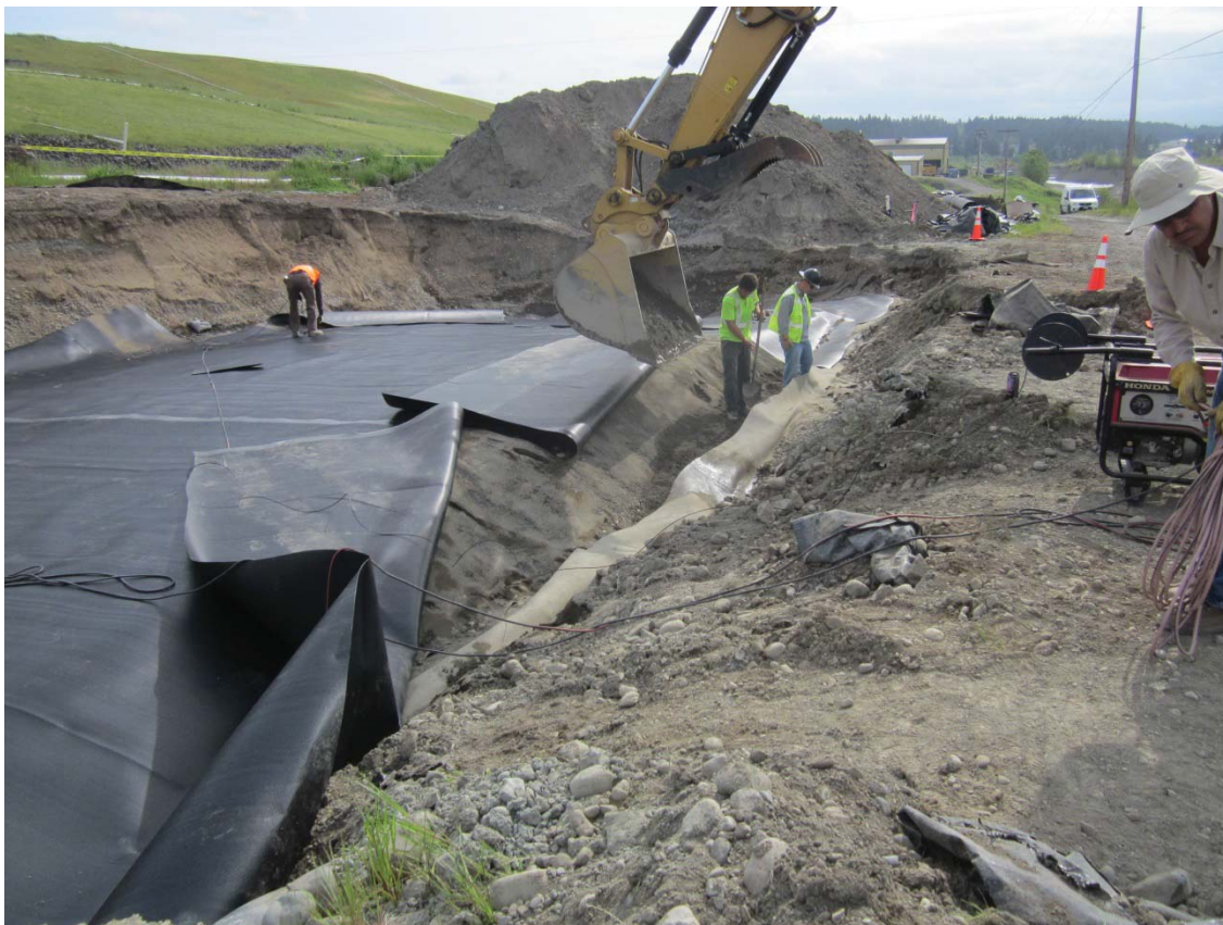
2014, May 16. Geomembrane placement; west sinkhole
