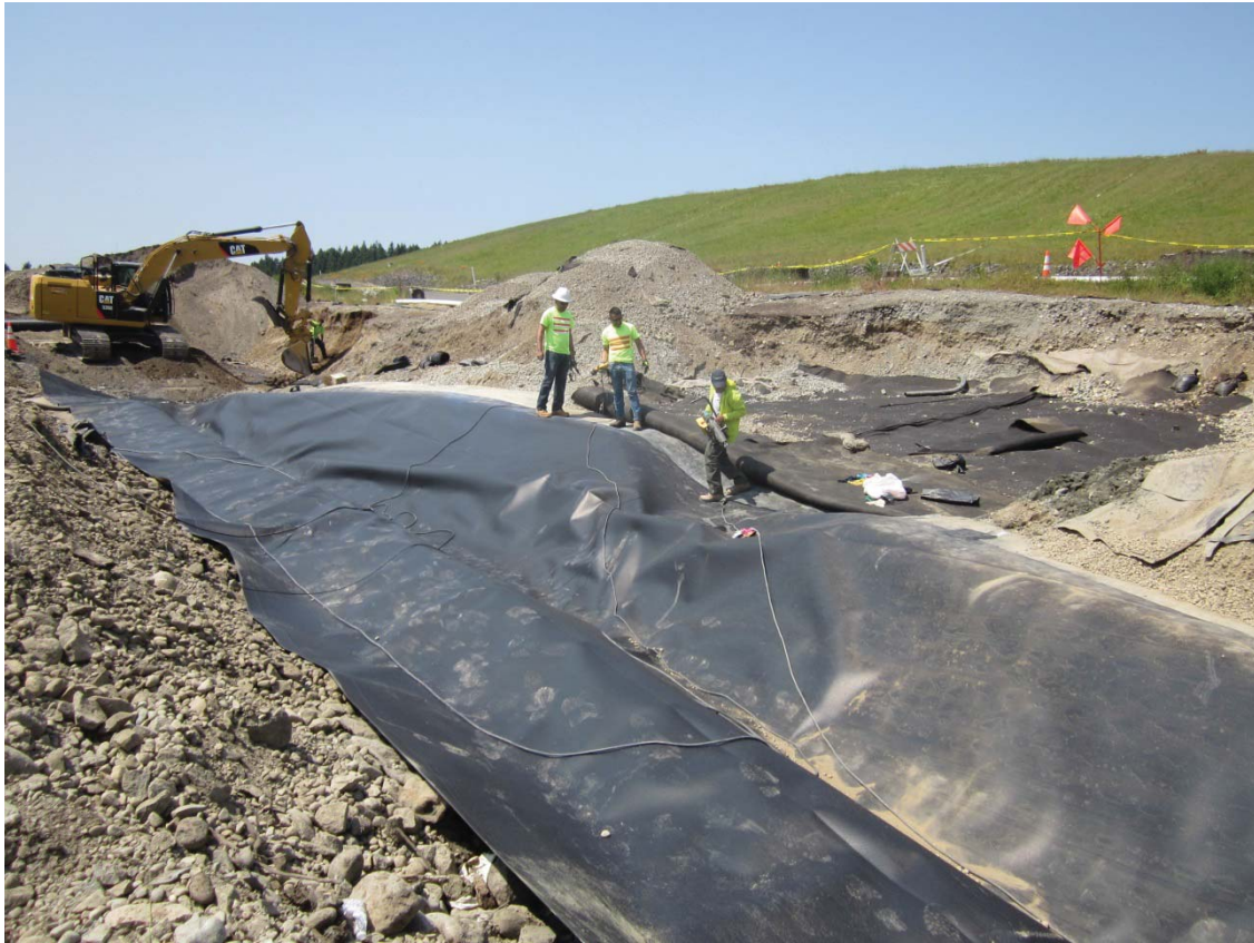
2014, May 30. Geomembrane installation.
