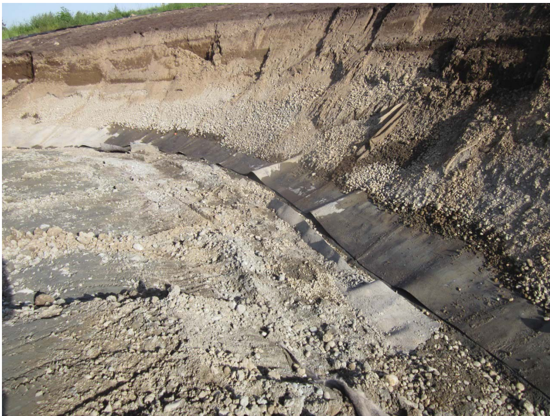
2014, May 14. Excavation at west sinkhole; viewing west.
