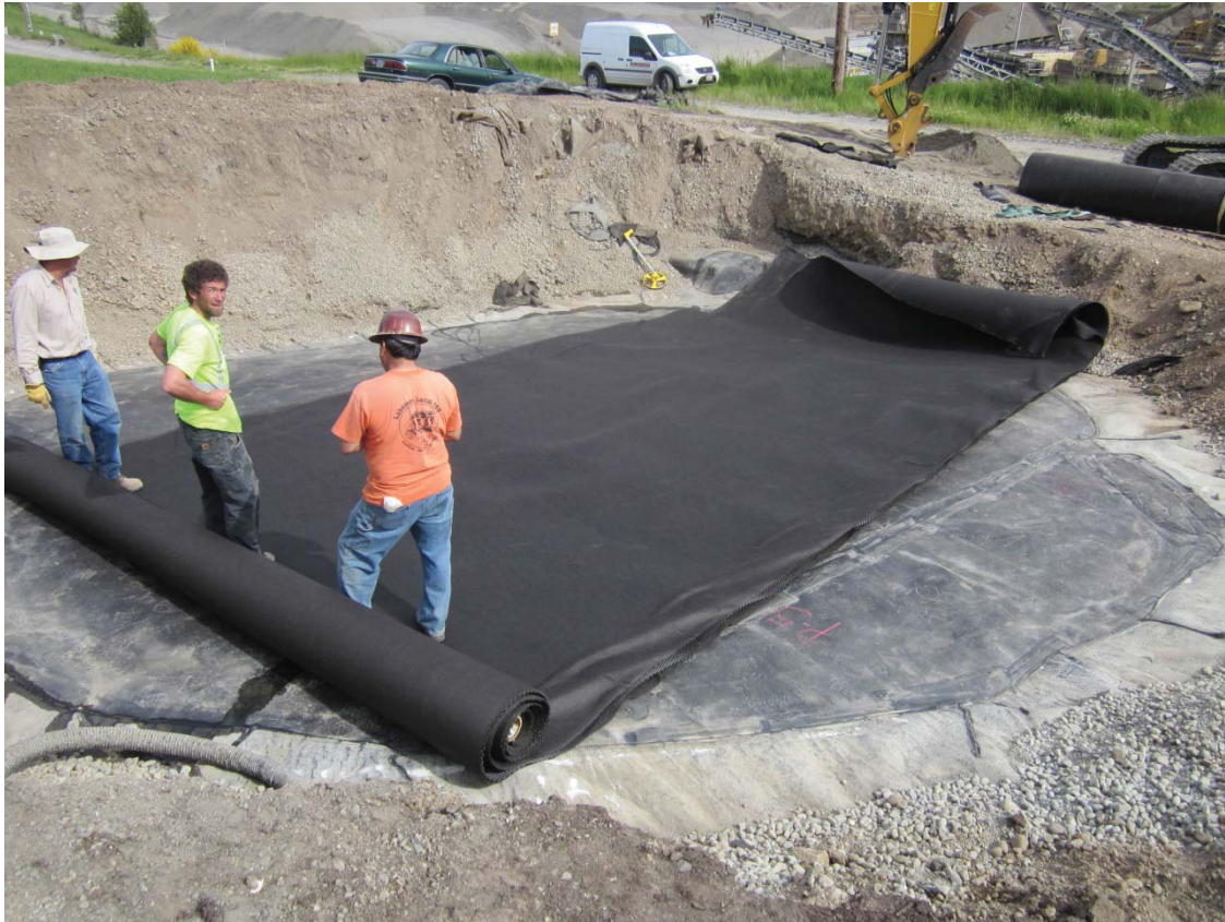
2014, May 16. Geonet composite installation; east sinkhole
