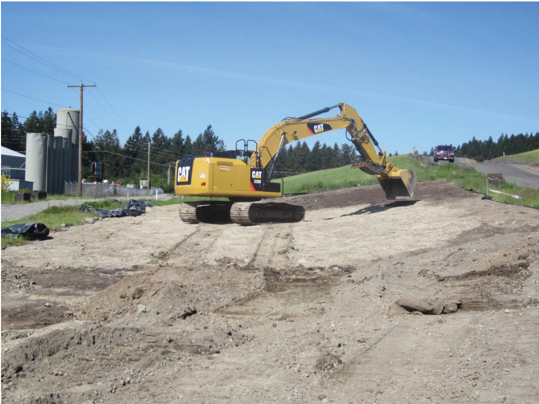
2014, May 13. Initial excavation at west sinkhole.
