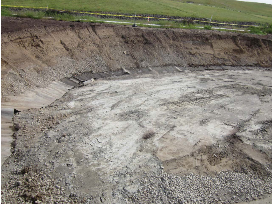
2014, May 15. Excavation at west sinkhole.
