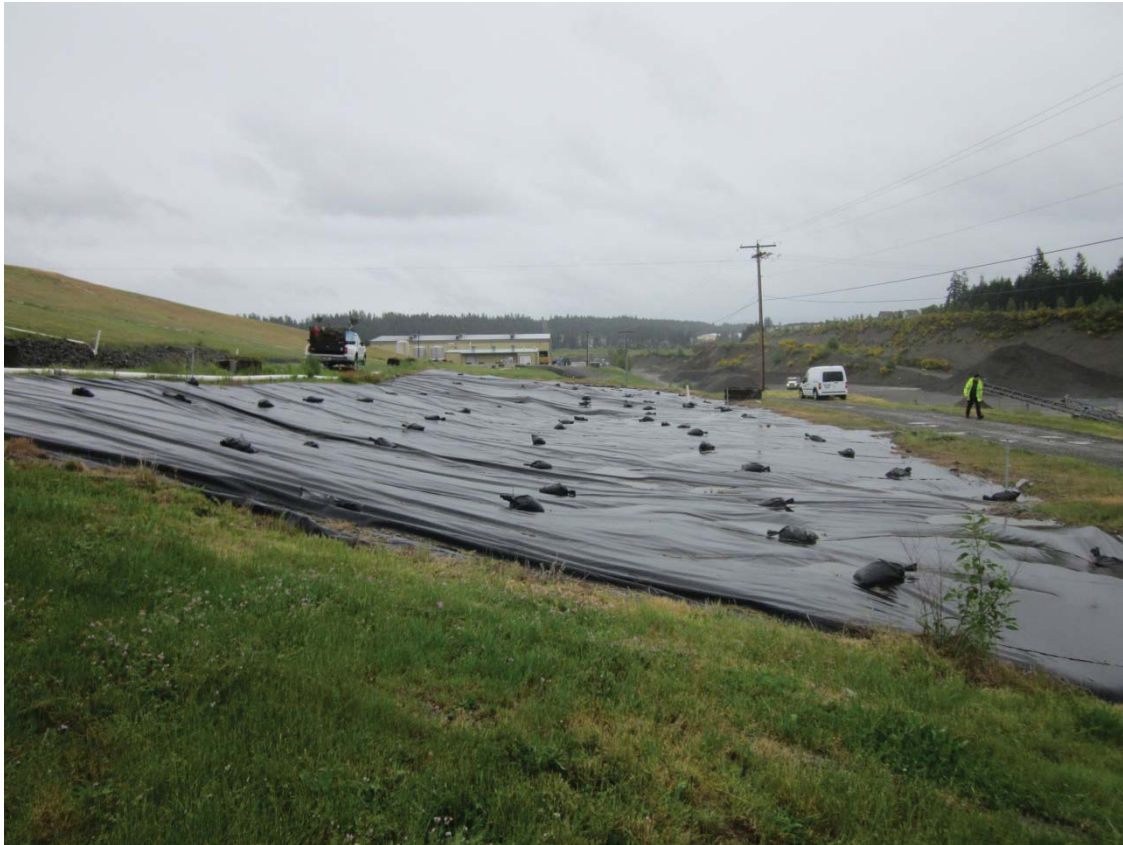
2012, May 23, viewing east.
