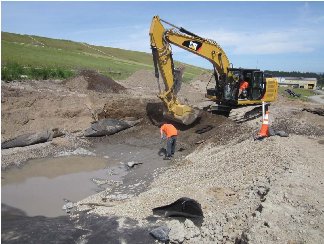
2014, May 22. Additional excavation to re-establish drainage.
