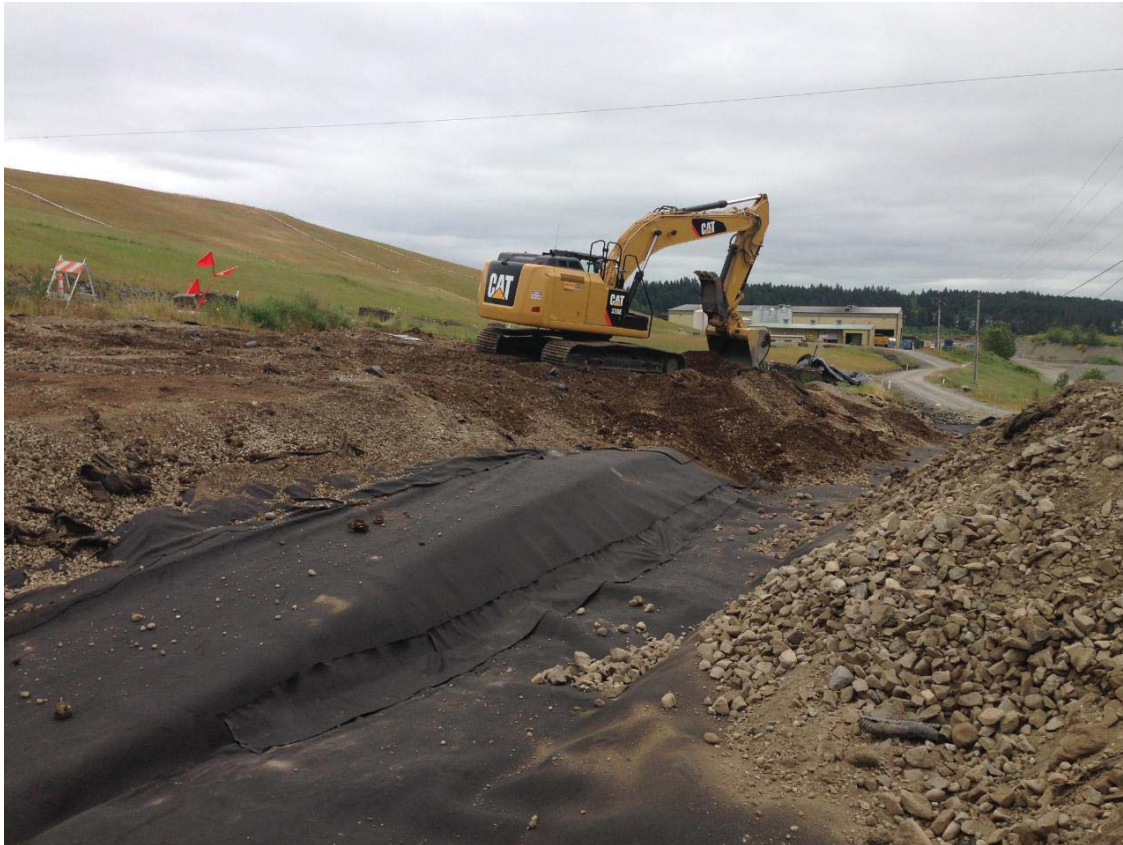
2014, June 3. Placement of cover soil.
