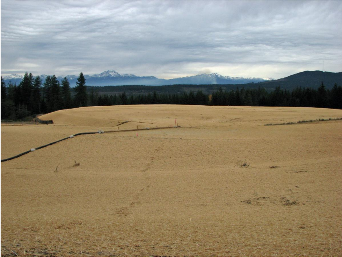
Figure 5a: Norseland, November 14, 2007. This photo was taken just after a minimum of four feet of fill was added on top of the required permeable cover. Straw has been placed to control erosion until vegetation can be established.
