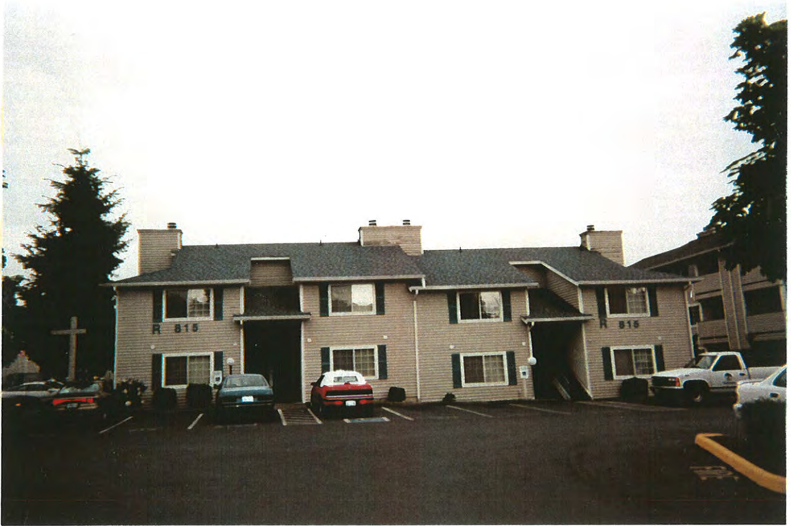
Lora Lake Apartments typical 2-story building.
