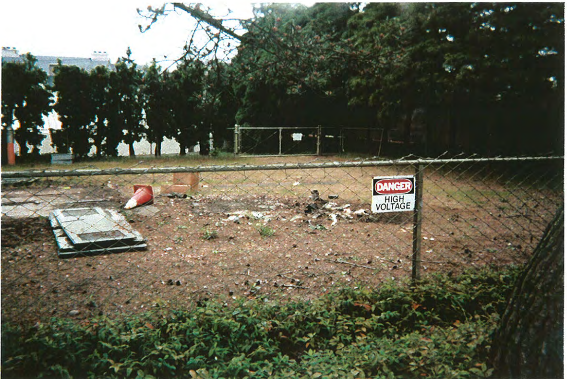
Looking north at the east end of the former transformer station.
