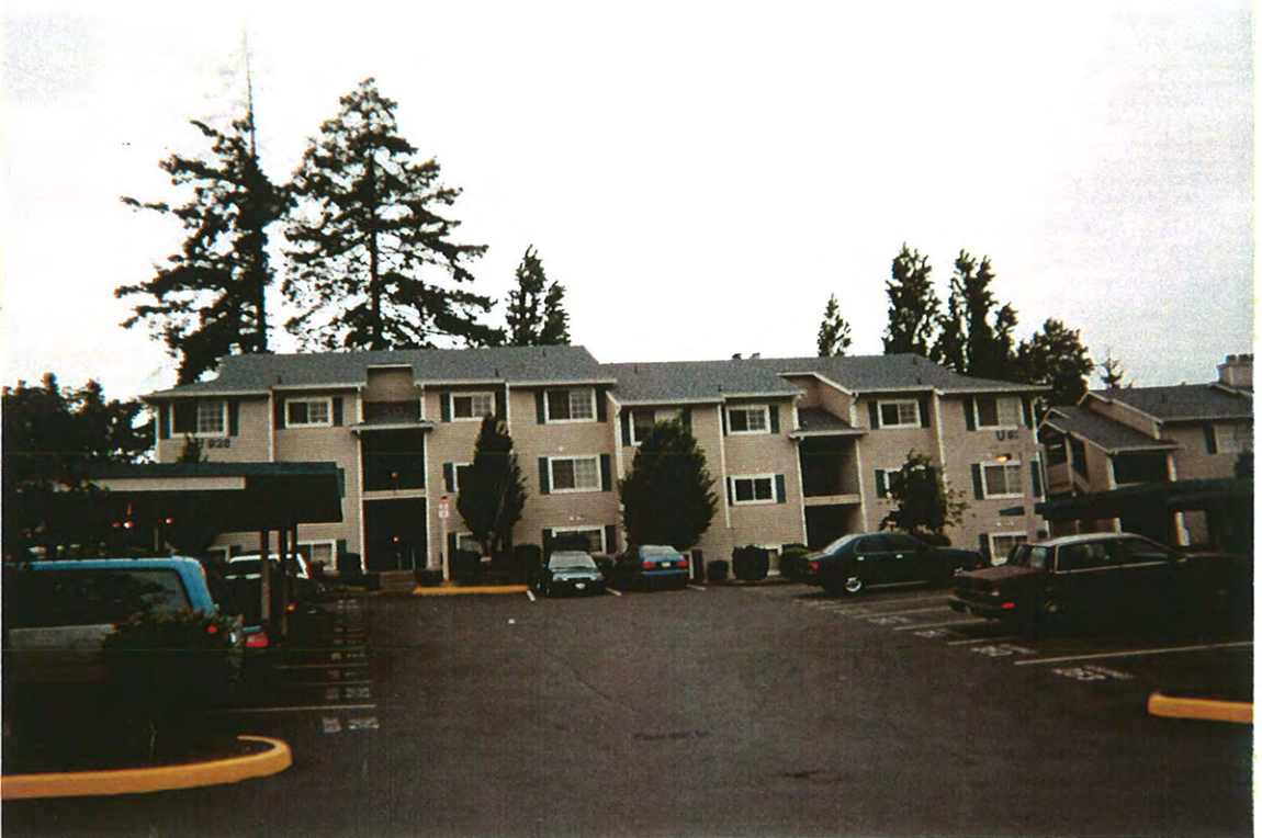
Lora Lake Apartments typical 3-story building.
