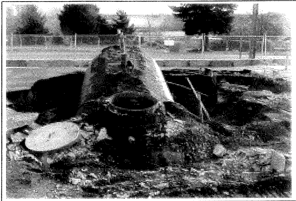
Photo 7. 15,000-gallon USTs floated to surface due to high water table after hold-down straps were cut. Second UST is still in ground to right of photograph.
