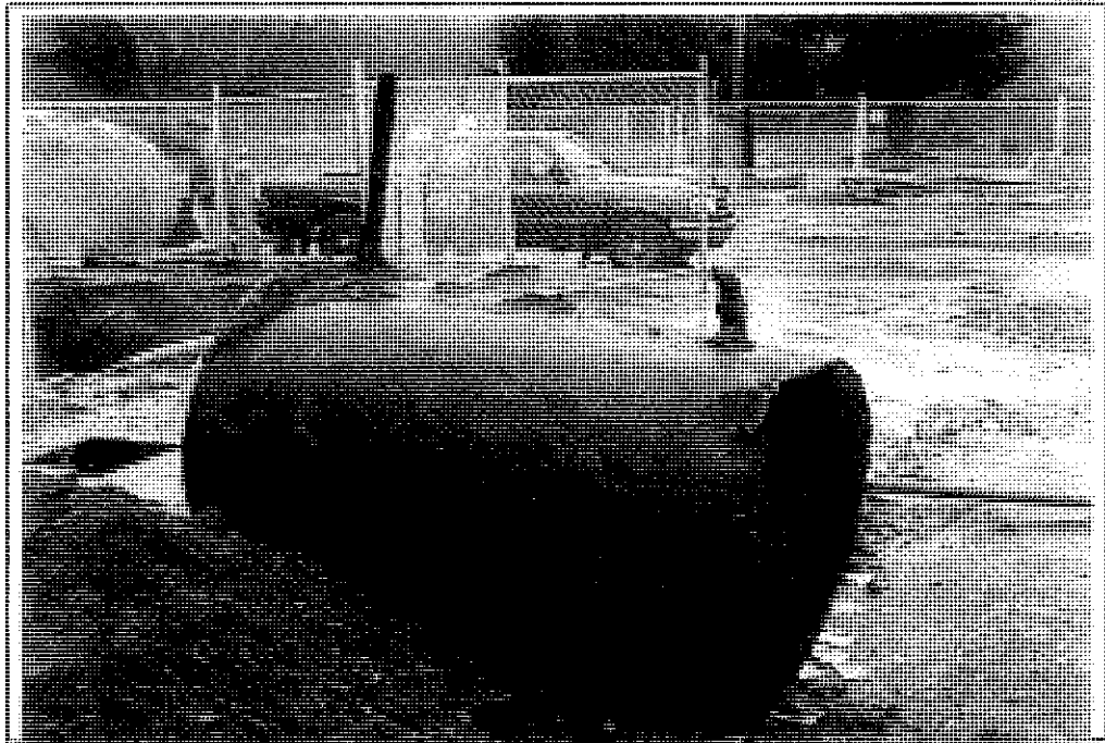
Photo 13. 500-gallon heating oil UST after removal.
