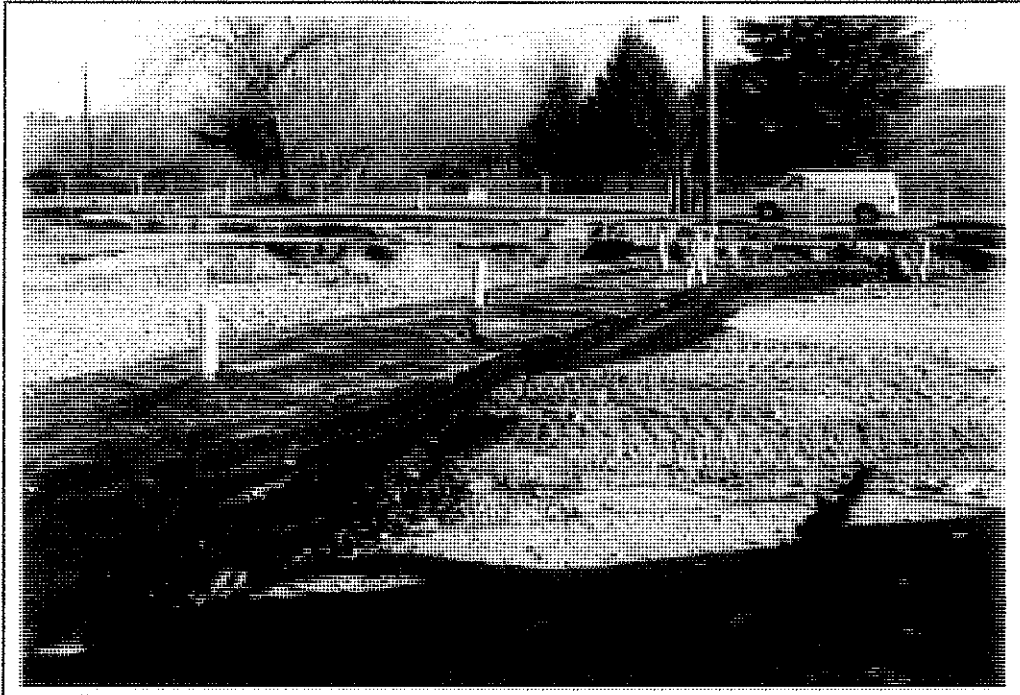
Photo 23. Placing subgrade fabric on top of spalls prior to backfilling with clean site soils. Temporary wells were later completed flush with the surface using steel well monuments.
