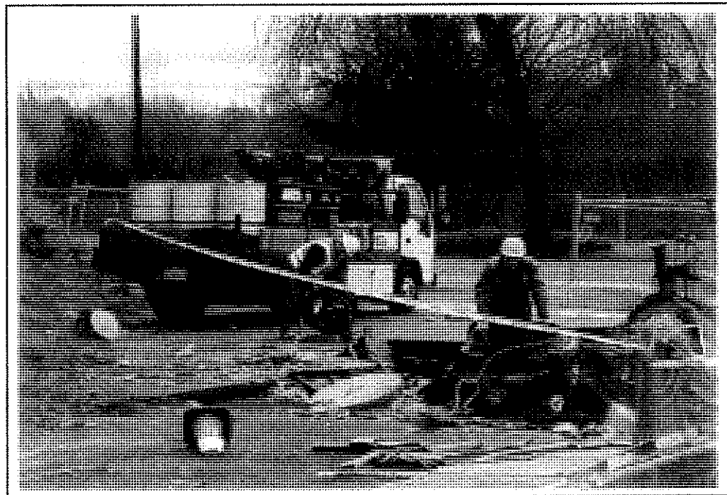
Photo 4. Gasoline and diesel fuel tanks being pumped and rinsed prior to removal.
