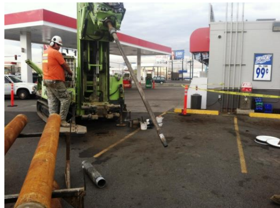
Photo #4: Drilling of borehole MW-8. Photo looking southwest towards the fuel dispenser island
