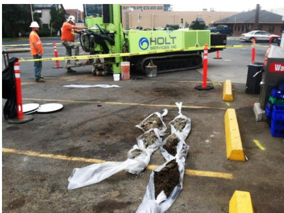
Photo #5: View of boring MW-8 advanced using a sonic rig. Soil cuttings from the boring for lithology description and screening of volatile organic compounds are shown in the foreground.
