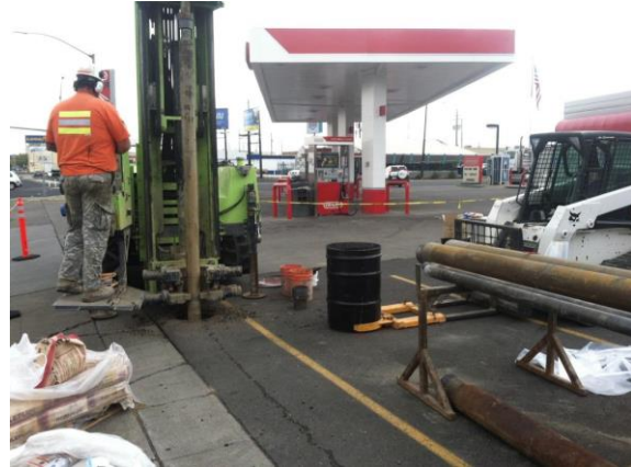
Photo #2: Drilling borehole MW-6 located downgradient from the fuel dispenser island shown in the background. Photo looking west
